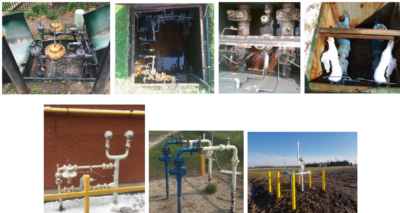
Figure 5.2-66: Examples of Distribution System Stations
