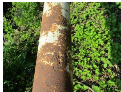
Figure 5.2-14: Coating degradation and corrosion pitting
