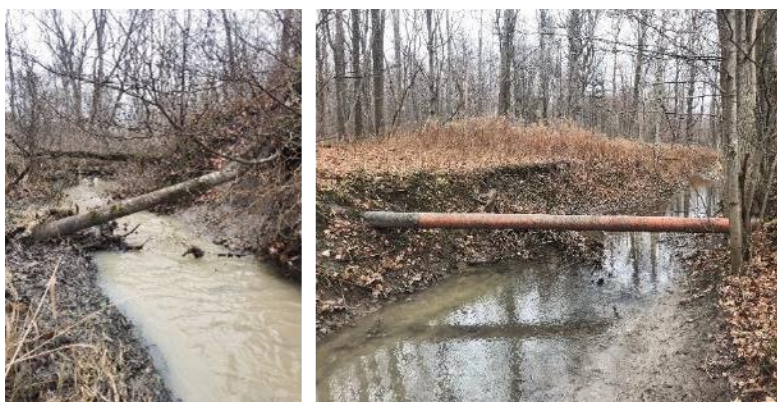
Figure 5.2-55: Corrosion
