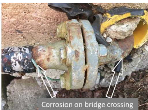
Figure 5.2-9: Severe corrosion on bridge-crossing pipe
