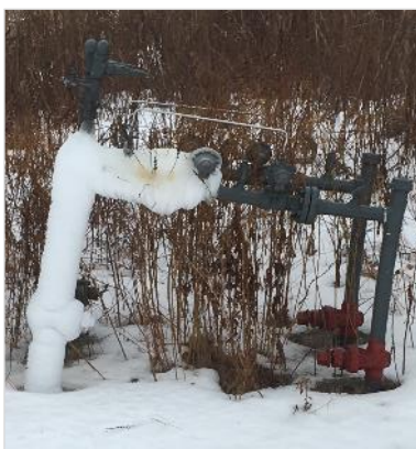
Figure 5.2-68: The Joule-Thomson Effect on a District Station
