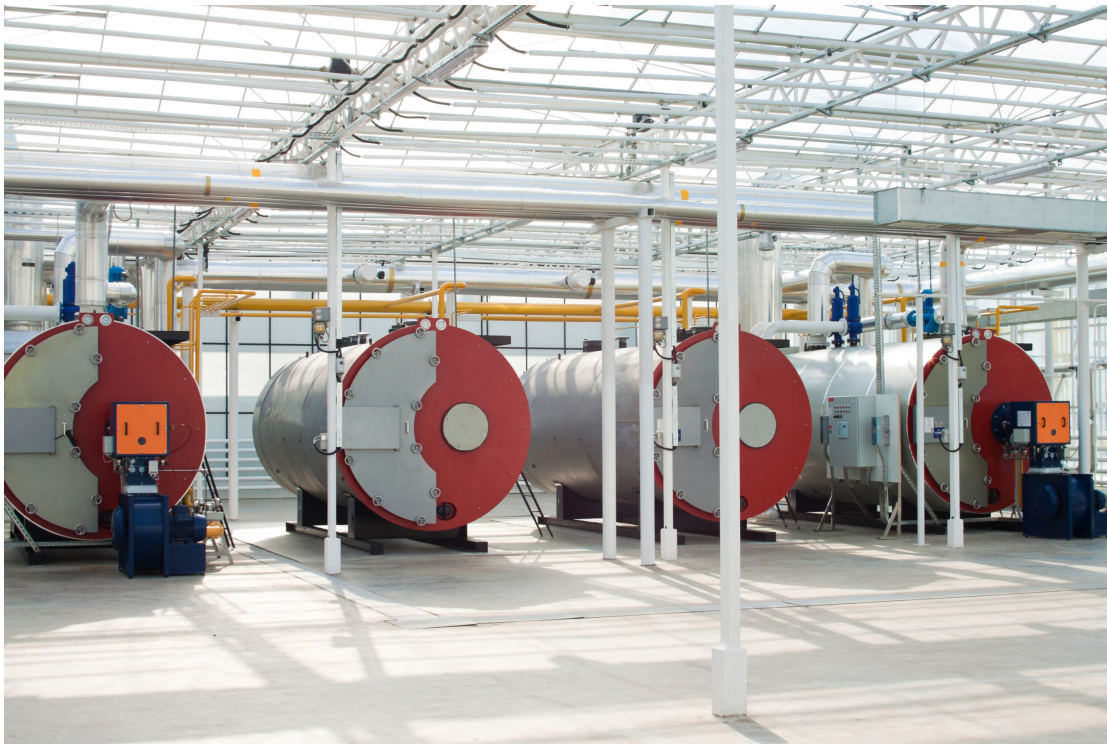
Natural gas powered boilers in a commercial greenhouse. Image from shutterstock.com
