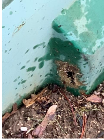
Figure 1: Fibreglass Deterioration Examples – Foundation Holes
