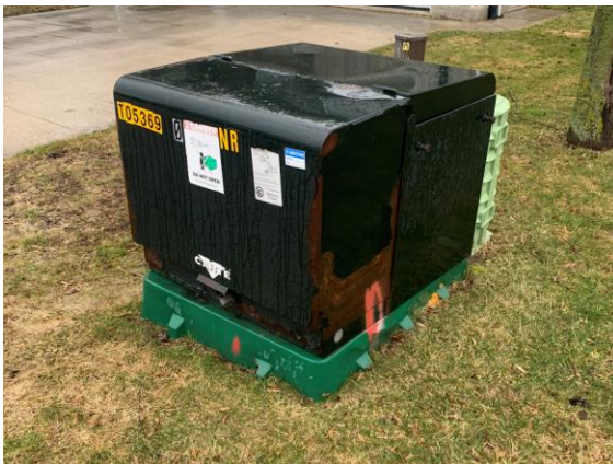
Figure 2: Fibreglass Deterioration Examples – Foundation Dips
