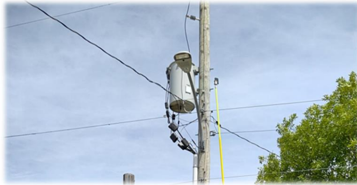
A Pole-Mounted Transformer
