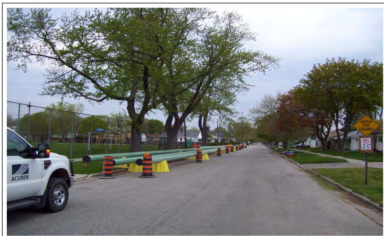
Whenever possible, pipe was stored in front of non-residential areas to allow access to driveways. In this case, the pipe was strung and welded in front of city parkland.
