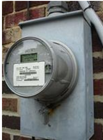
Figure 17: Smart Meter Installation at Customer Location.
