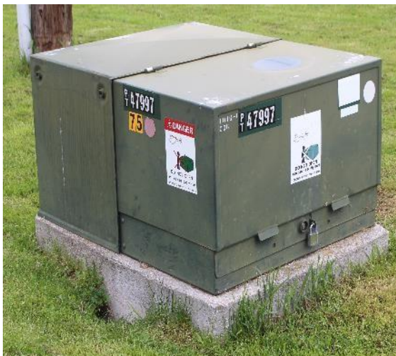
Figure 11: Padmounted Transformer
