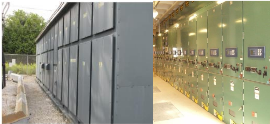
Figure 13: (Left) Outdoor Enclosure Housing Metal clad Switchgear. (Right) Indoor Metal clad Switchgear
