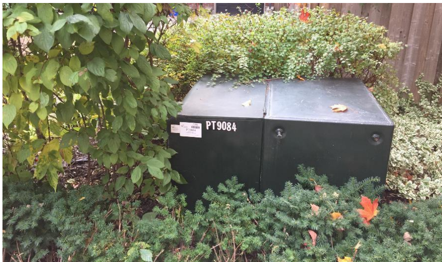
Figure 16: Padmounted Transformer Requiring Vegetation Removal
