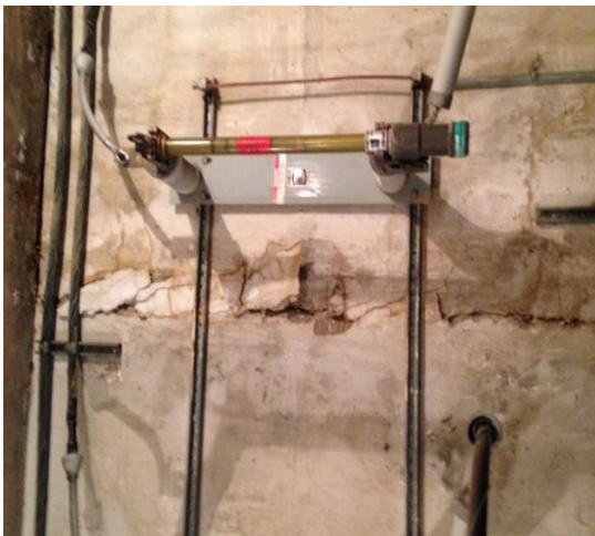
Figure 4: Cracked Walls
