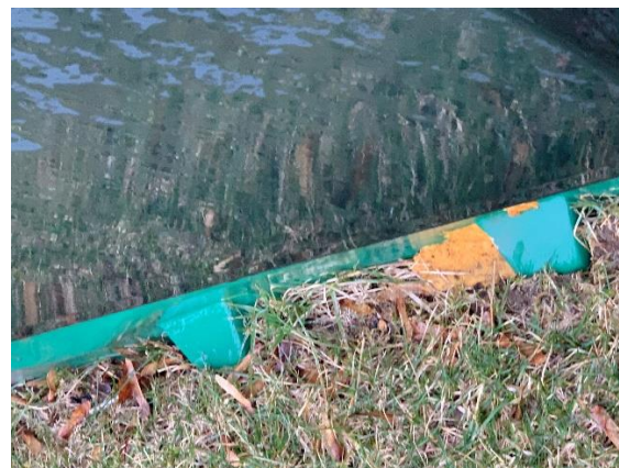
Figure 2: Fibreglass Deterioration Examples – Foundation Dips
