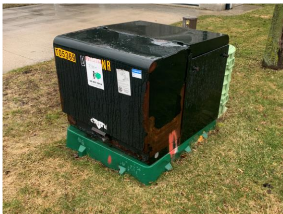
Figure 2: Fibreglass Deterioration Examples – Foundation Dips
