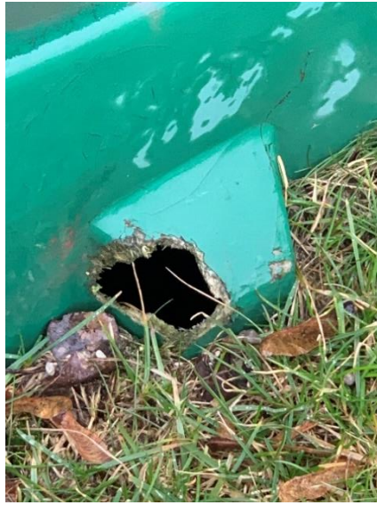
Figure 1: Fibreglass Deterioration Examples – Foundation Holes
