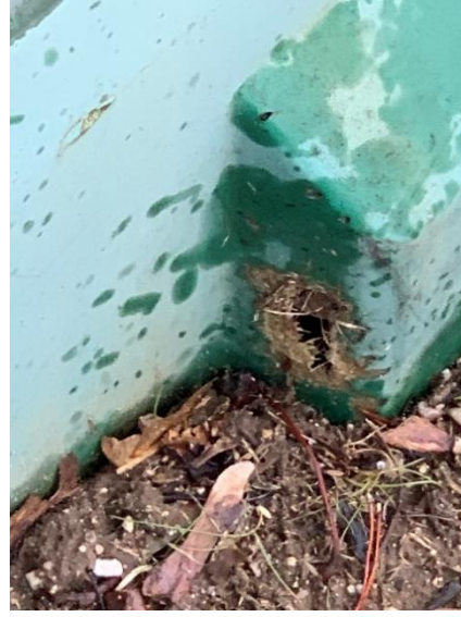
Figure 1: Fibreglass Deterioration Examples – Foundation Holes
