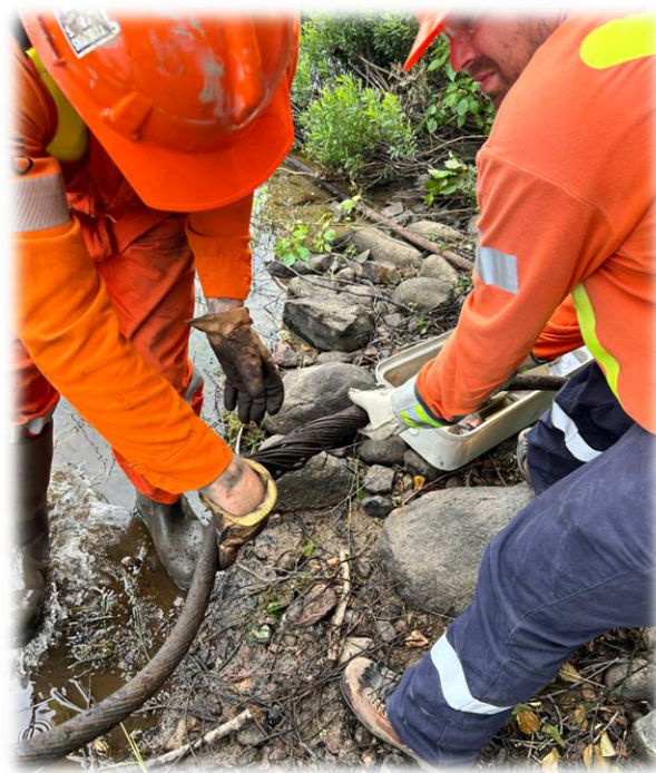
Hydro One and Chapleau PUC Staff Repairing Sub Cable
