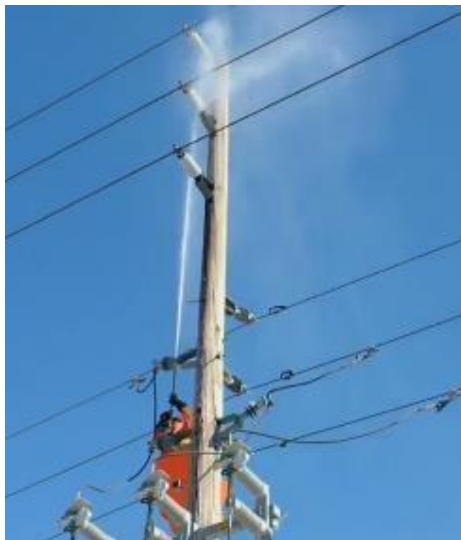
12 Figure 9: Porcelain Insulator Washed Using a High Pressure Water Jet 13
