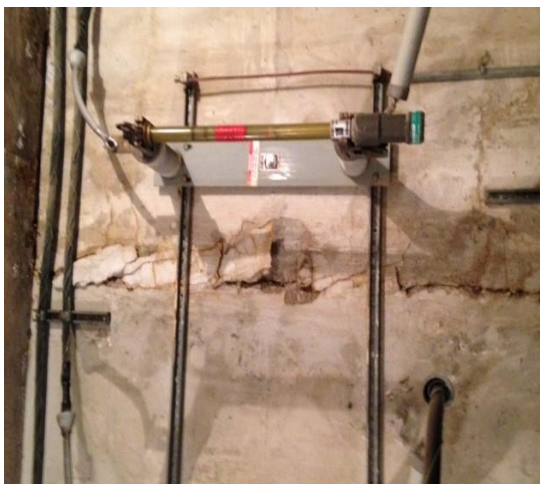
Figure 4: Cracked Walls
