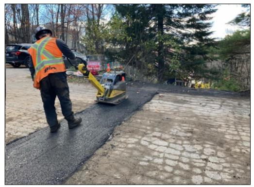
5. Where it was necessary to open cut road crossings or driveways, they were restored as soon as possible following pipeline installation.
