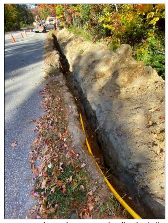
2. Where rocky conditions were encountered, a trench was excavated to allow for pipeline installation.
