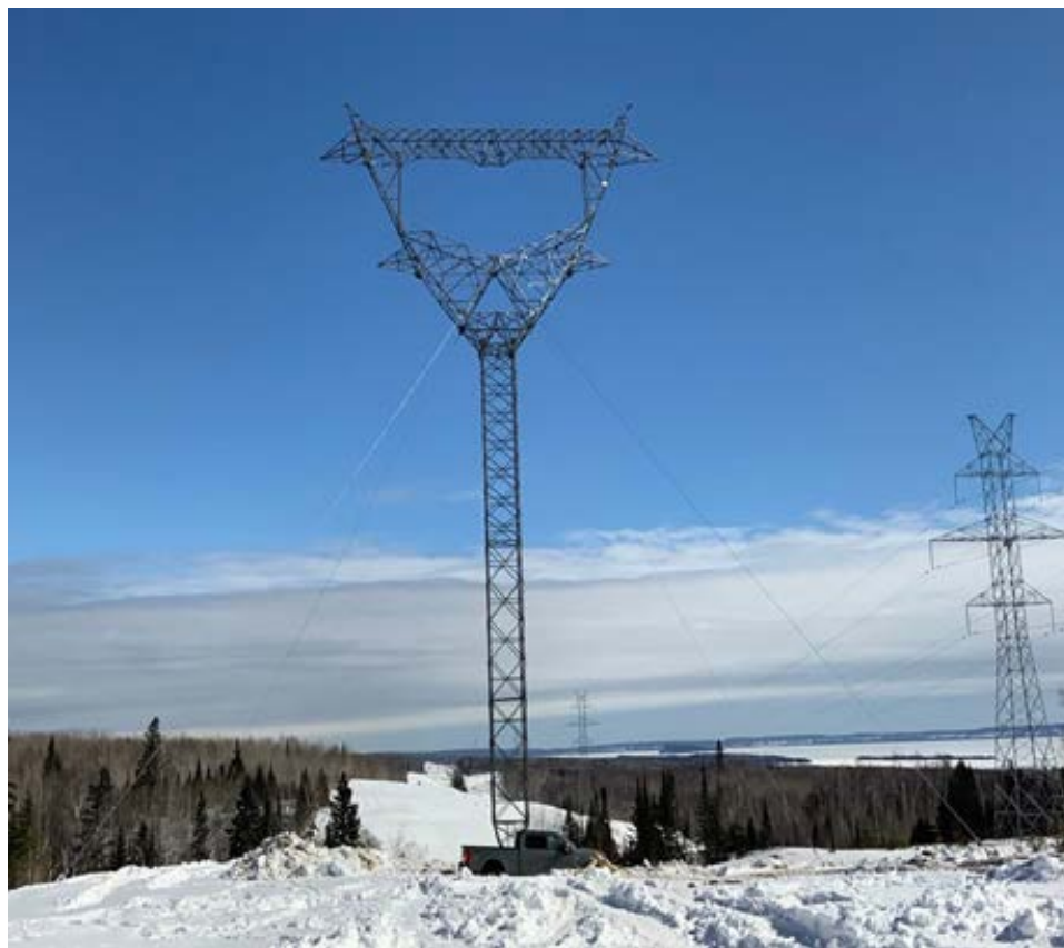
First tower erected February 29 2020
