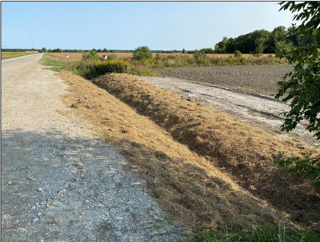
6. Sediment and erosion control measures were installed where required and will remain in place until the land is stable and vegetated.
