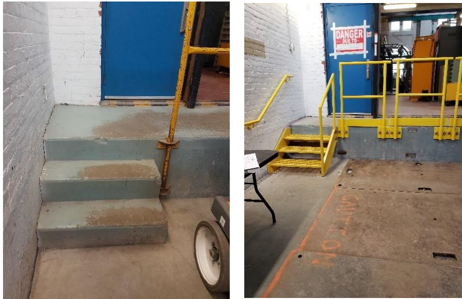
Figure 9: Example of Terauley Station, replacing non-code-compliant stairs and railings with functional ones, and improved dock access.
