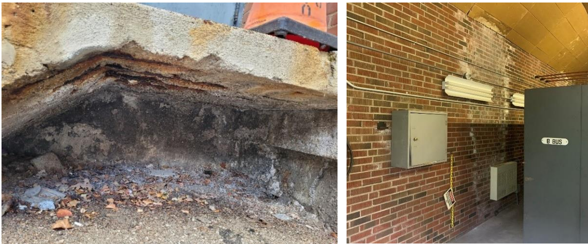
Figure 8: Examples of architectural deterioration at stations, from left to right: George and Duke Station deteriorated concrete stairs, Centre Drive Station water infiltration from roof.
