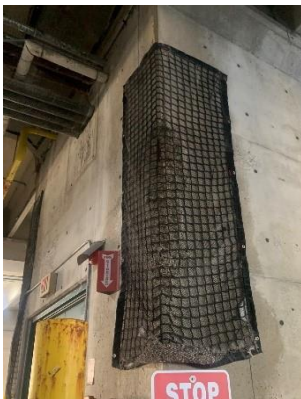
Figure 5: Examples of structural deterioration at work centres, from left to right: 500 Commissioners Building C – spalling concrete wall with preventative netting; 500 Commissioners Building C – exposed deteriorated waterproofing; 500 Commissioners Building C – rusted steel staircase.
