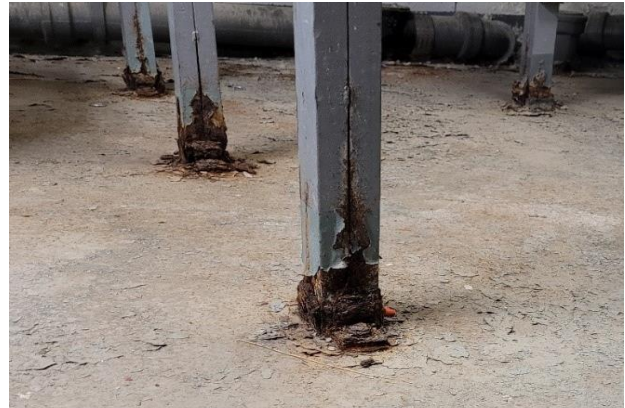
Figure 4: Examples of structural deterioration at stations, from left to right: Windsor Station cracked concrete floor slab, Windsor Station corroded rebar columns.
