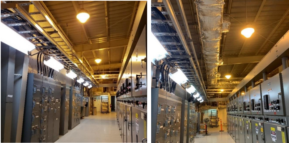
Figure 14: Examples of HVAC additions at Stations: Cavanagh Station without additional air conditioning (left) and after with ducts and venting installed for keeping air temperature and equipment cool (right).
