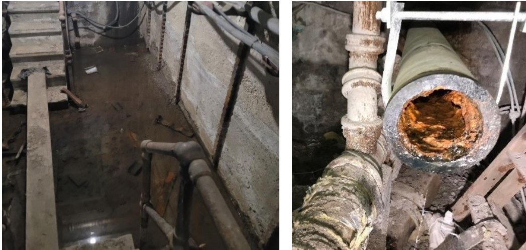
Figure 12: Examples of mechanical and plumbing deterioration at Stations: Terauley Station with a flooded basement and Terauley Station water service line clogged and full of debris.
