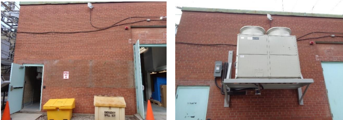
Figure 13: Examples of HVAC additions at Stations: Strachan Station without additional air conditioning (left) and after with two new condensing units installed for keeping air temperature and equipment cool (right).
