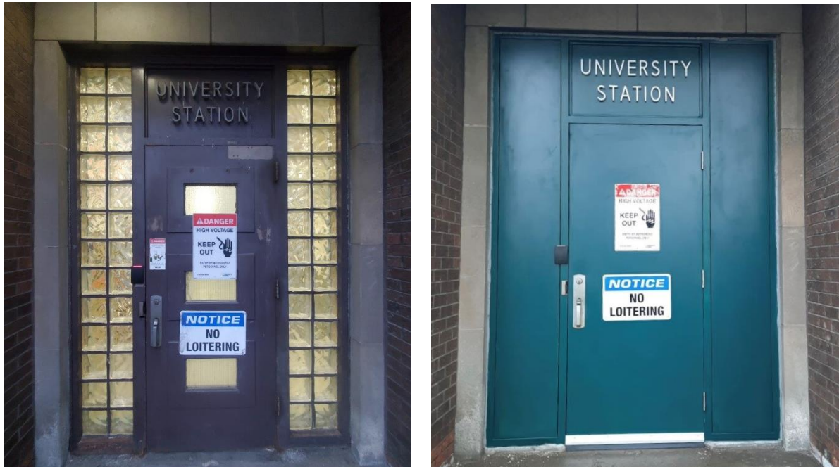
Figure 18: Examples of University Station entrance door in poor condition (left) and after being retrofitted via the station door program (right).
