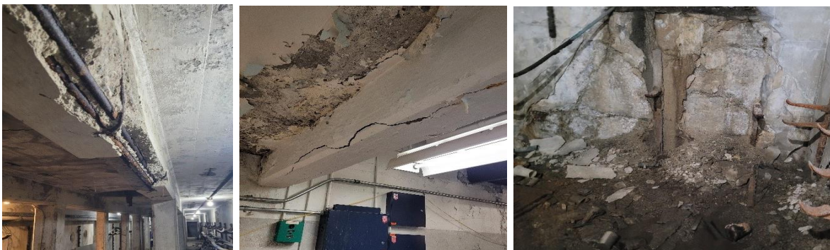
Figure 16: Examples of existing stations in critical condition, from left to right: George and Duke Station, beam with exposed rebar, Defoe Station cracked beam, Junction Station deteriorated foundation wall.
