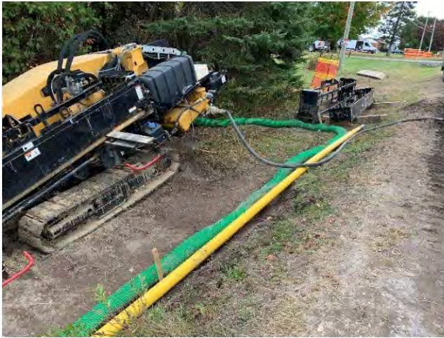
Photo 1: HDD drill rig staged and drilling within the 8 th Line Road ROW ditch. Silt sock established around drill rig during drilling to prevent off-site release of drilling mud.
