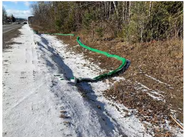
Photo 16: Silt sock retained in place over the winter of 2023/2024 to limit the potential for offsite sedimentation.
