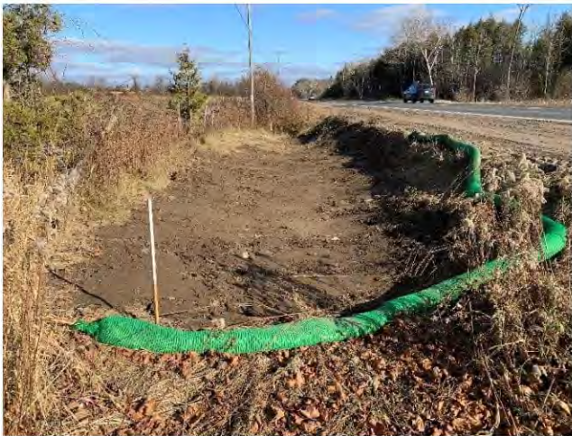
Photo 15: Silt sock retained at a temporarily reclaimed tie-in pit within the 8 th Line Road ROW.
