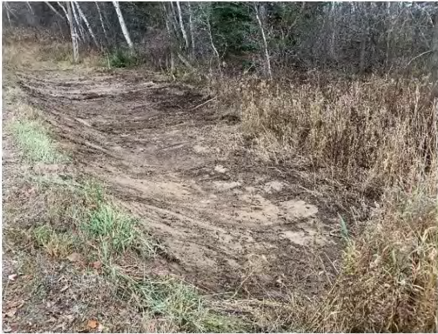
Photo 13: Temporarily restored tie-in pit.
