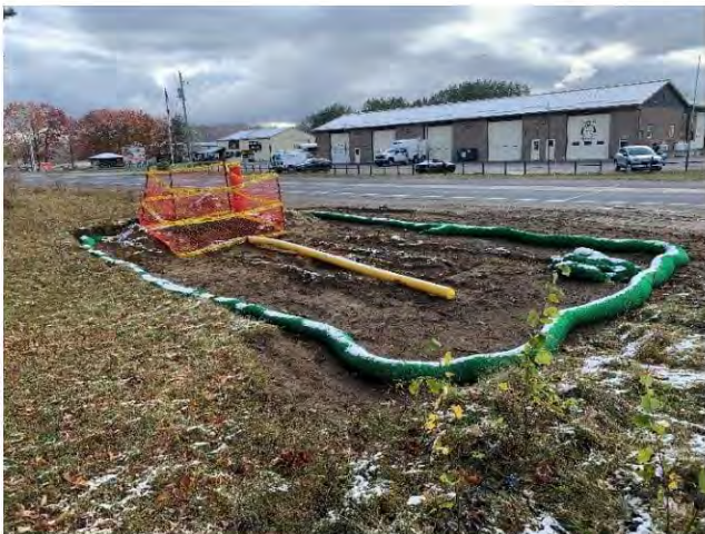
Photo 5: Established silt sock maintained in place after the completion of drilling.
