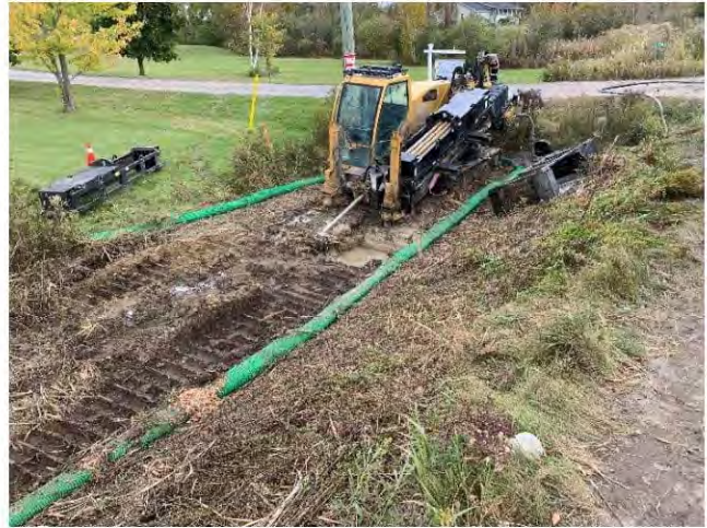
Photo 2: HDD drill rig staged and drilling within the 8 th Line Road ROW ditch. Surface disturbances within the road ROW ditch contained within silt sock barrier.
