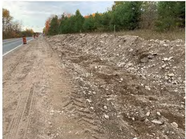
Photo 10: Temporary restoration of gravel slope after open-trench installation requirement along 8 th Line, east of Centreline.
