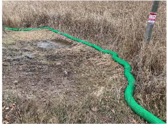
Photo 14: Silt sock established around perimeter of tie-in pit.
