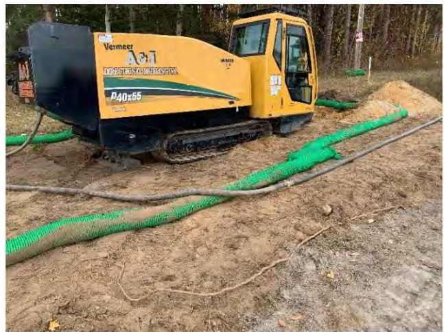
Photo 4: Silt sock surround drilling rig for road crossing at the intersection of 8 th Line and Centre Line.
