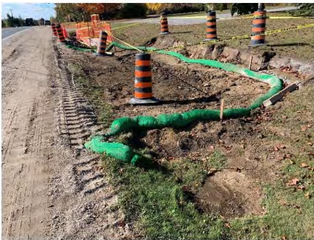
Photo 3: Silt sock maintained in road ROW ditch after mobilization of HDD drill rig.
