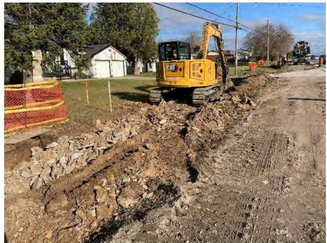
Photo 6: Open trenching within the road ditch near the eastern tie-in for the Project.
