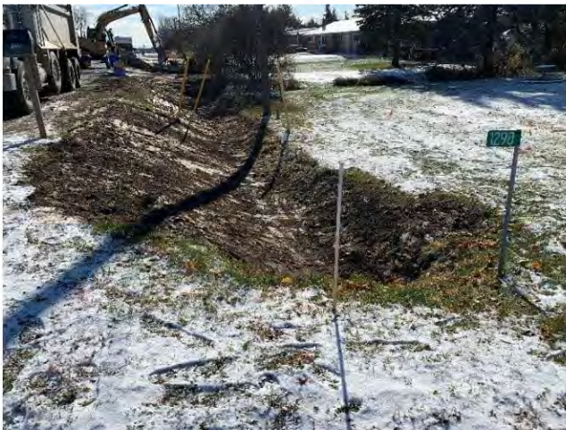
Photo 17: Backfilled and temporarily reclaimed road ditch at tie-in location within the 8 th Line Road ROW.
