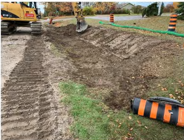
Photo 11: Backfilled and temporarily restored tie-in pit within the 8 th Line Road ROW.
