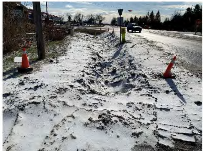
Photo 18: Backfilled Buckhorn Road ROW ditch requiring additional final grading and final restoration.
