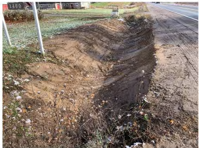
Photo 12: Backfilled and temporarily restored tie-in pit within the 8 th Line Road ROW.
