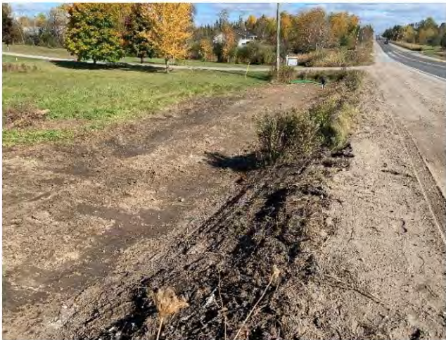
Photo 9: Sydenham River; Graded and seeded HDD rig area is germinating well.
