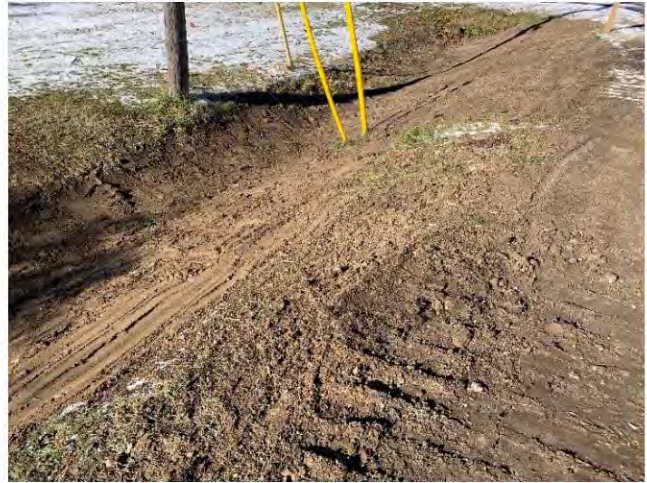
Photo 8: Temporary restoration completed of backfilled open-trench on the Buckhorn Road ROW, south of 8 th Line.
