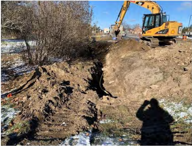
Photo 7: Actively backfilling open-trench excavation along the Buckhorn Road, south of 8 th Line.
