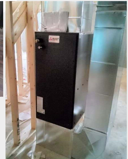
Heat Pump 200% – 425% efficiency COP: 2.00 to 4.25
