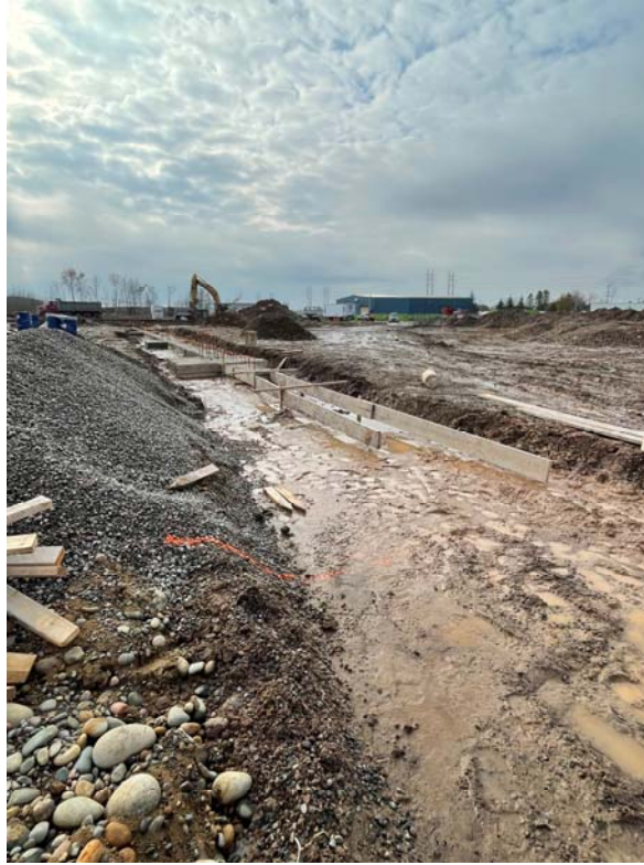
Photo 2 – Perimeter Strip Footing (Looking Southwest)
