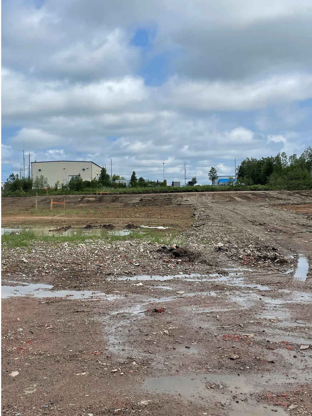
Photo 2 – Looking East from the Sackville Road Entrance Area.
