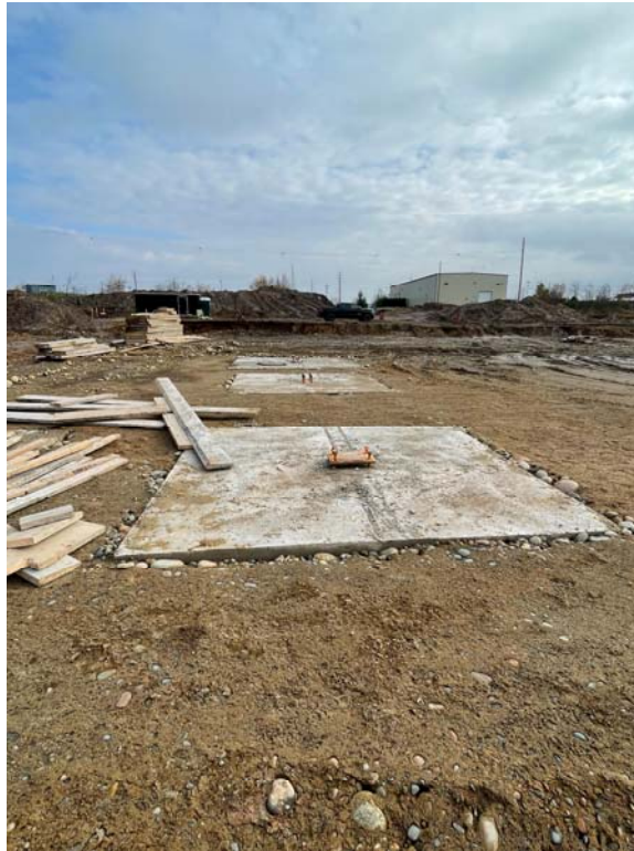
Photo 3 – Interior Spread Footings
