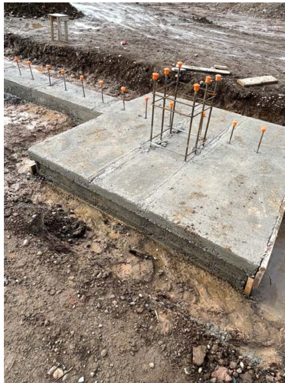
Photo 1 – Perimeter Pier Footing
