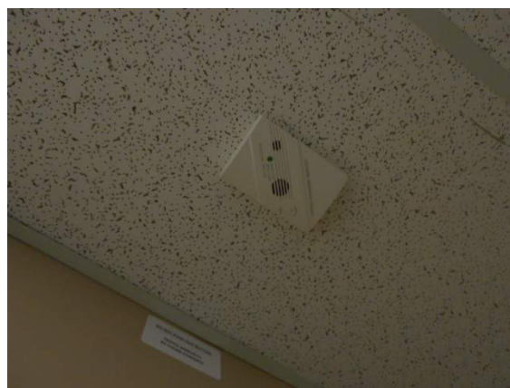
Ceiling mounted Motion Sensor
