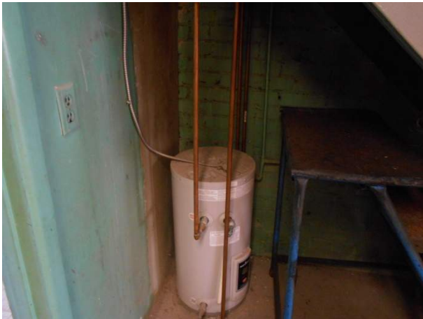
Domestic water heater in truck bay area
