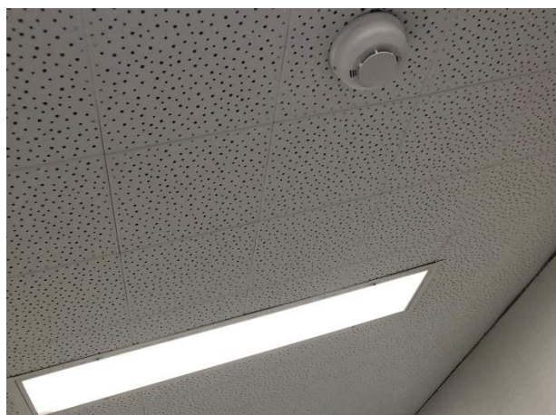
Ceiling Finishes – Acoustic Panel
