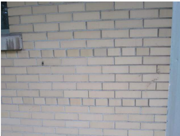
Overall view – brick masonry. Note bonding course every 6 th row of bricks.
