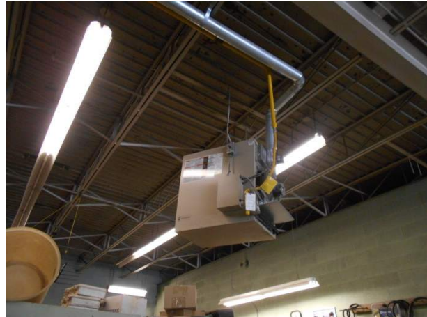
Unit heater in truck bay area
