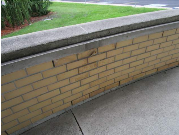
Tiny amount of brick deterioration – one brick.
