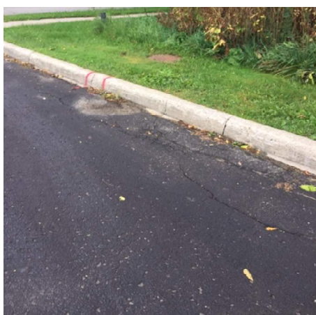
Longitudinal surface cracks in the east parking area
