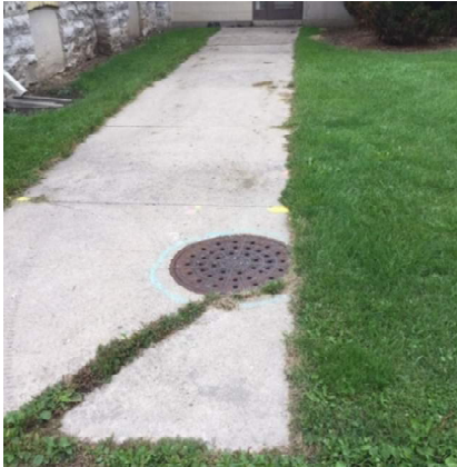
Area of deterioration on concrete walkway
