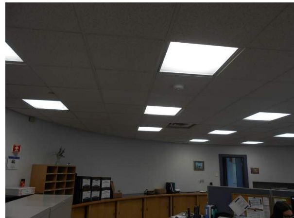
2'x2' Recessed Light Fixture
