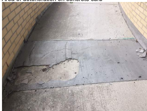
Area of deterioration on concrete walkway
