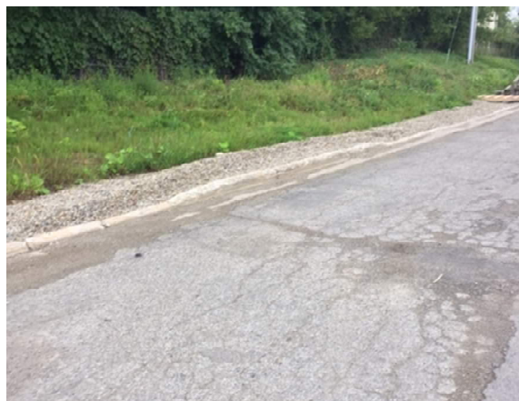
Deterioration in concrete curb
