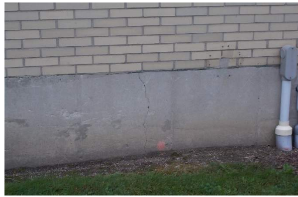
Cracking in foundation wall
