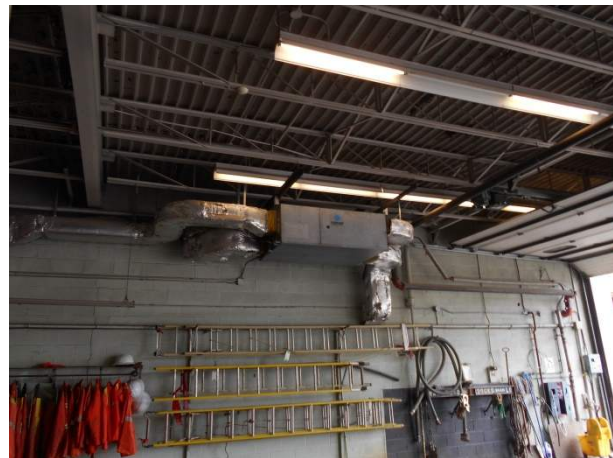
Heat recovery ventilator
