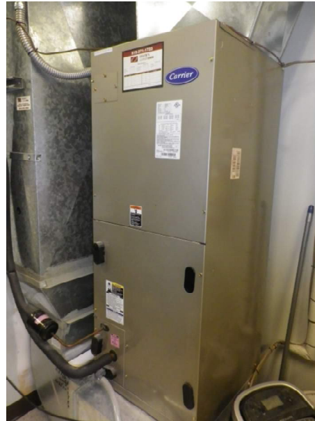
Fan Coil Unit – mechanical room
