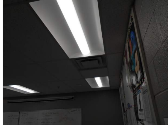
2'x4' Recessed LED Light Fixture
