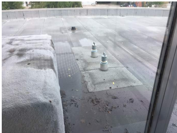
Low roof area – roof anchors added
