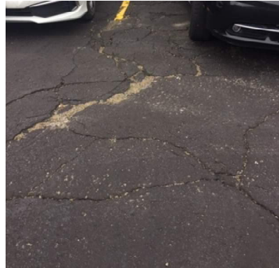
Deterioration in asphalt at loading bay
