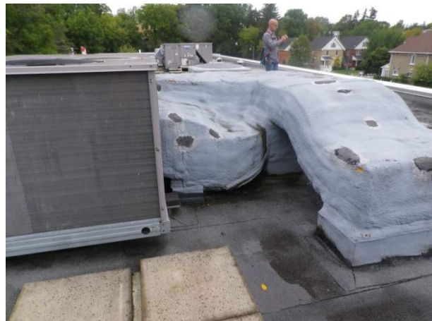
Exterior duct thermal insulation
