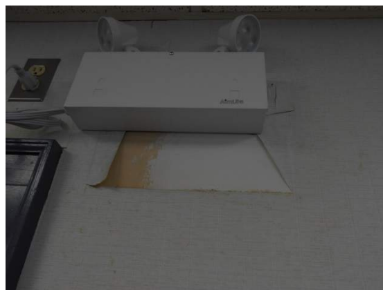
Emergency Battery with two Heads
