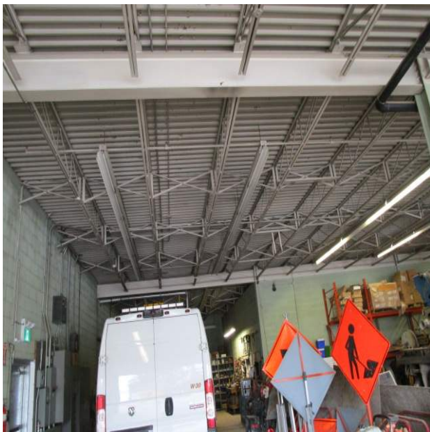
Ceiling – Exposed Painted Metal Deck
