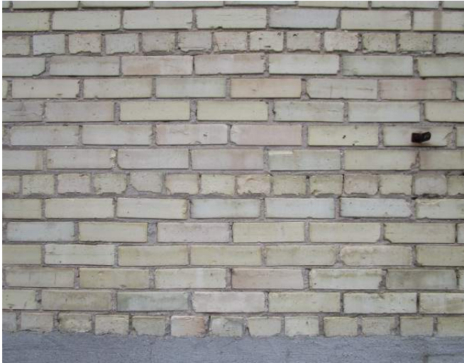
Brick masonry pattern, bonding course every 6 th row. Overall, masonry was found to be in good condition
