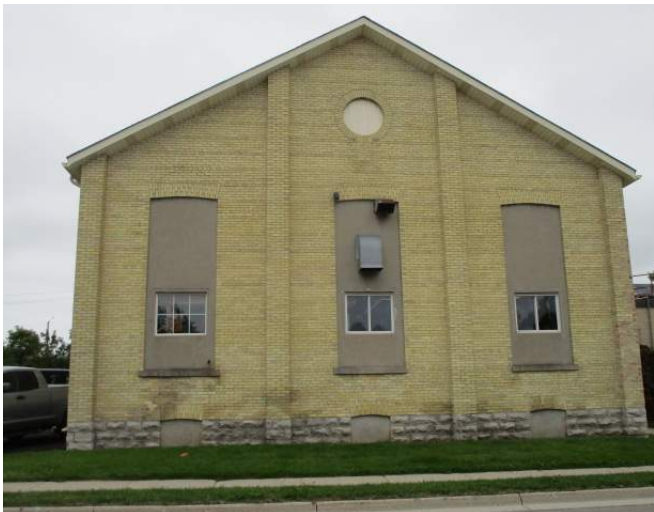
Original windows have been blocked in. Small, vinyl windows have been installed
