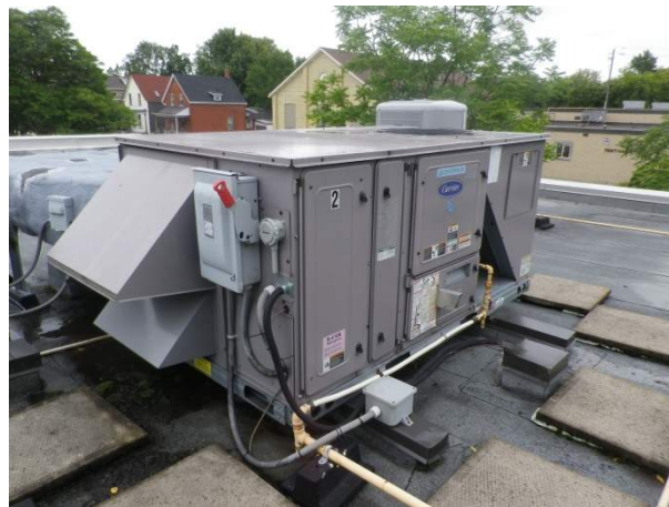
D3052 – Rooftop unit on high roof
