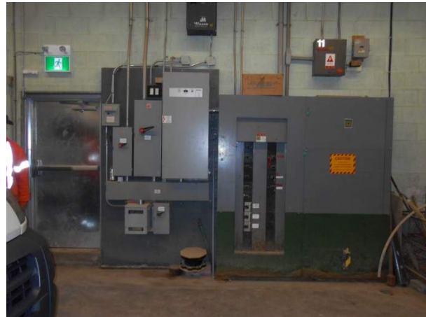
Main Distribution Panel and Transfer Switch
