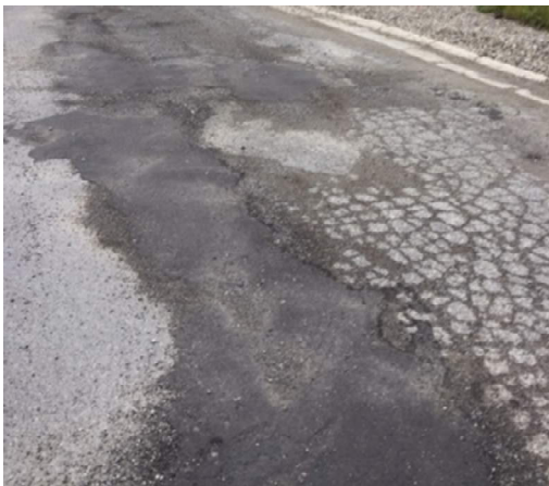
Deterioration in asphalt area north of building
