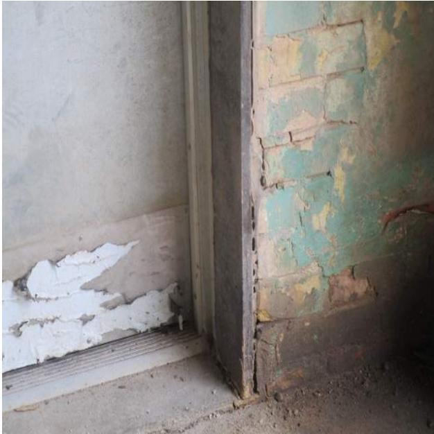
Wall Finishes Garage – Painted Block 1920s
