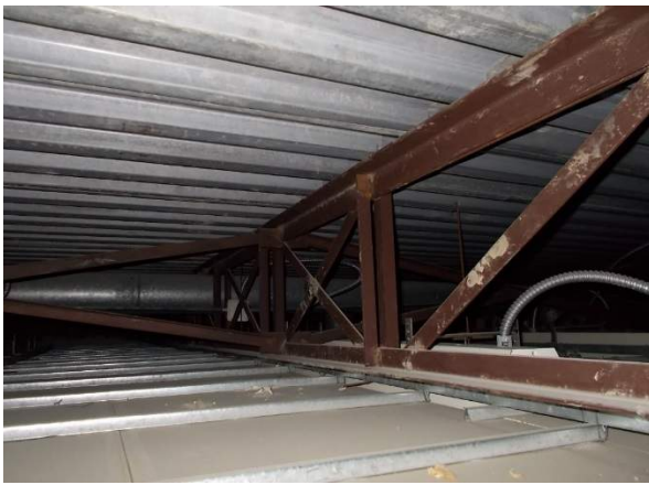
Roof raming of original section
