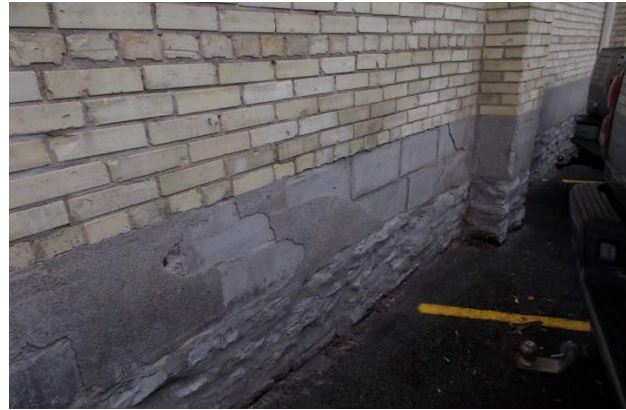
Stone rubble and concrete block with damaged parging on north truck bay building.
