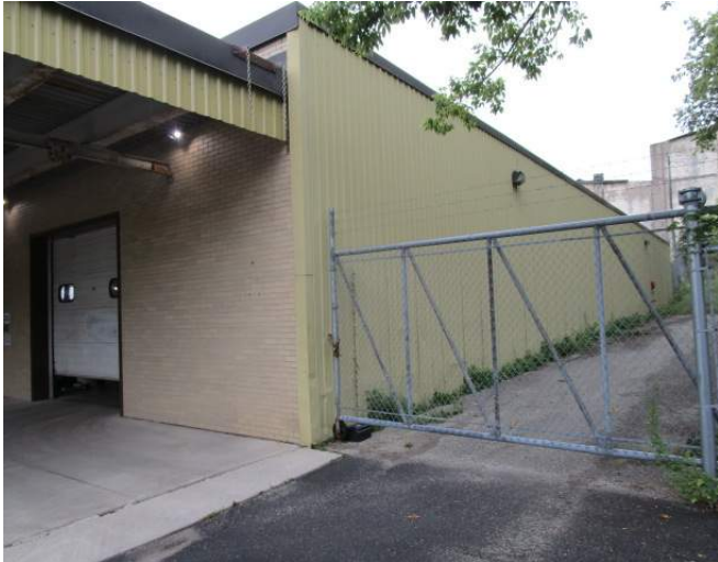
South elevation – 1950's Building Prefinished metal siding
