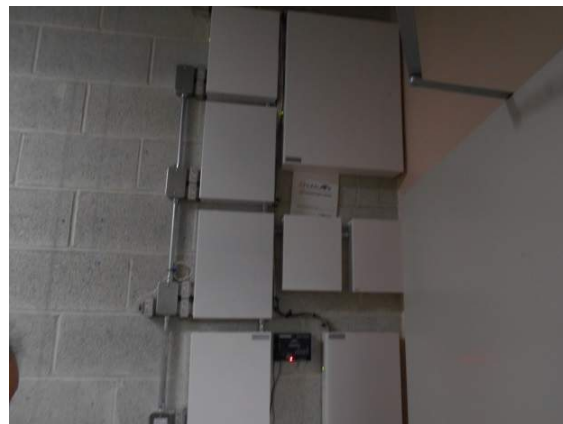
BAS / Security System control panels
