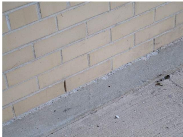
Weeping hole – brick masonry wall
