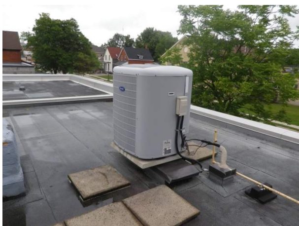
Fan coil condenser on roof
