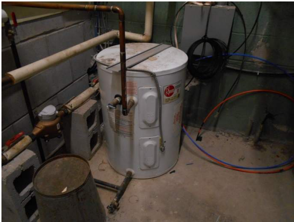
Domestic hot water heater in vault
