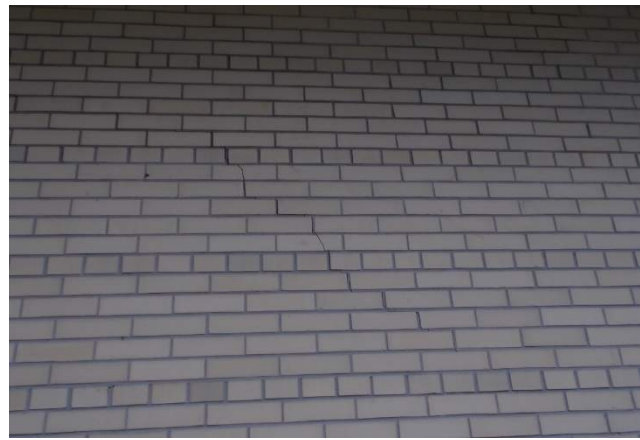
Step crack in exterior brick wall
