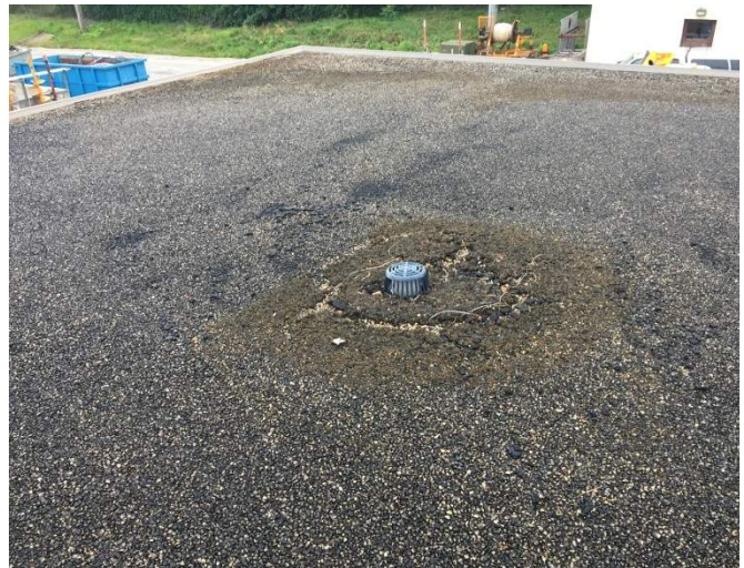
Debris at drain should be cleaned up to promote drainage of the roof.
