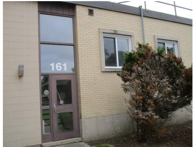
Original, entrance area to 1950's section of building. Original windows have been replaced with vinyl slider style windows.
