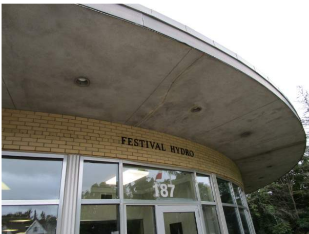
Large overhang – soffit constructed with transite panels
