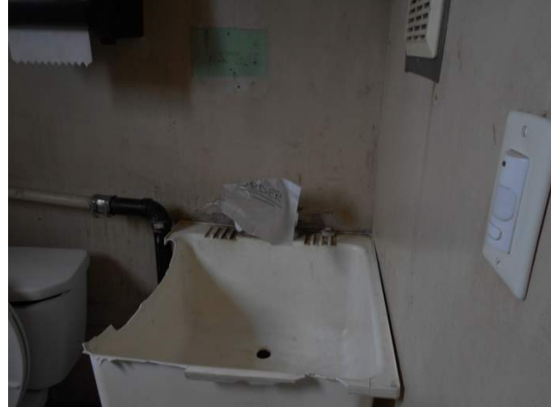
Broken washroom sink in truck bay washroom
