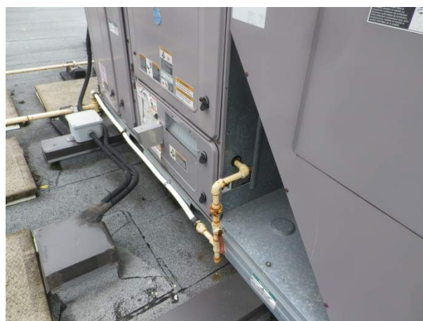
Rusty gas pipe connection
