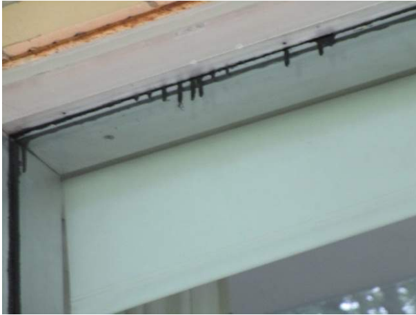
Glazing tape failure in original windows
