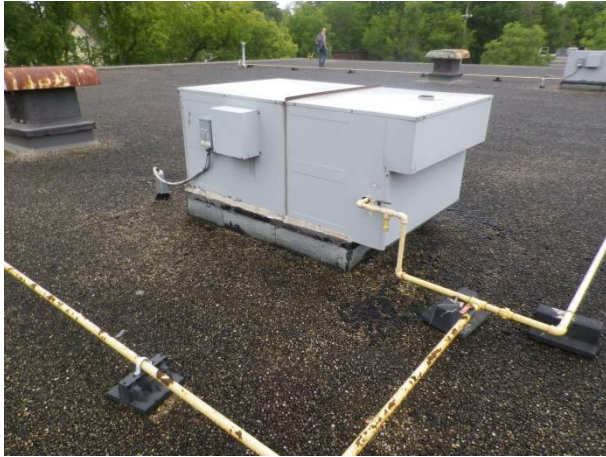
MUA unit serving large truck bay area
