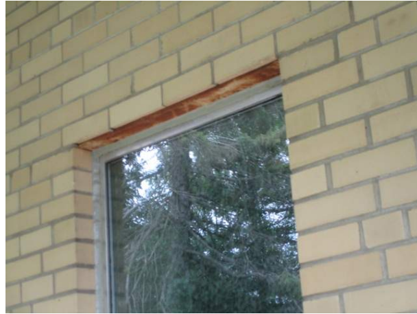
Minor corrosion on lintel
