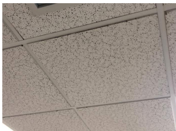
Ceiling Finishes – Acoustic Tile
