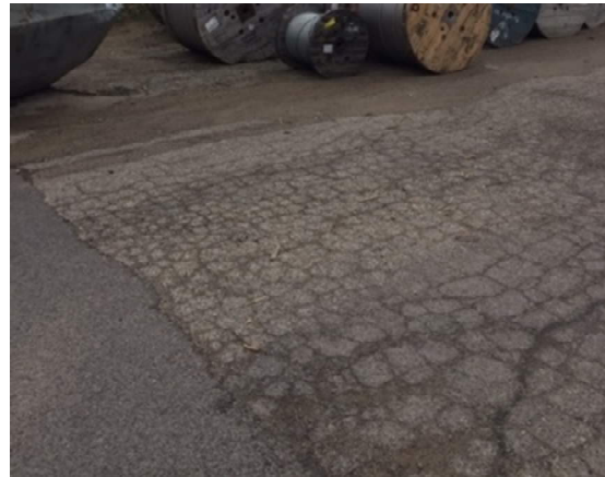
Deterioration in asphalt area north of building
