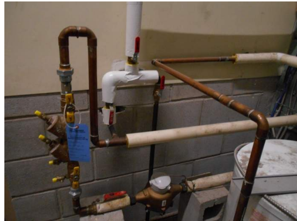
Domestic water meter and backflow preventer
