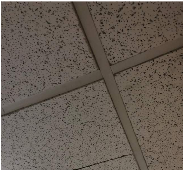
Ceiling – Suspended Ceiling Tile
