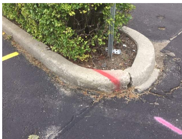
Area of deterioration on concrete curb
