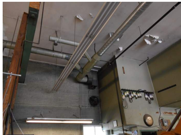
Two exhaust fans in truck bay area
