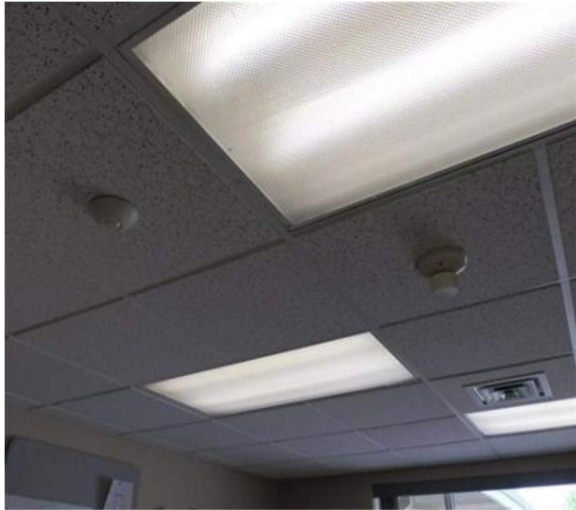
Heat and smoke detectors in addition
