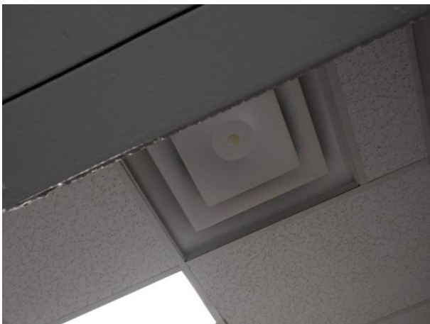
Rectangle ceiling diffuser
