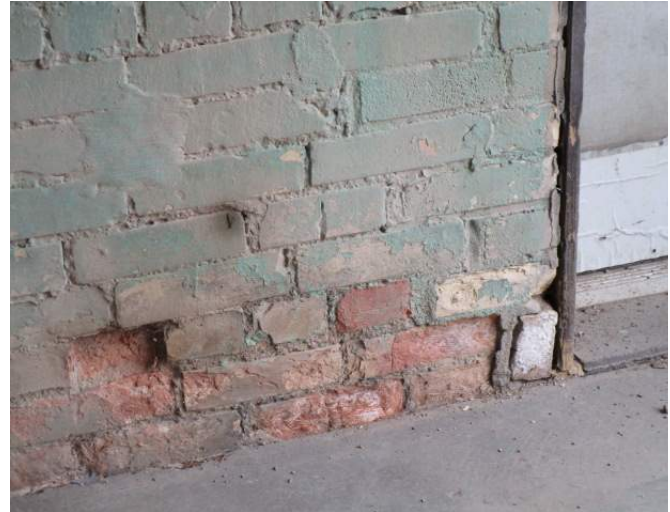
Tiny amount of masonry deterioration at the base of the door frame
