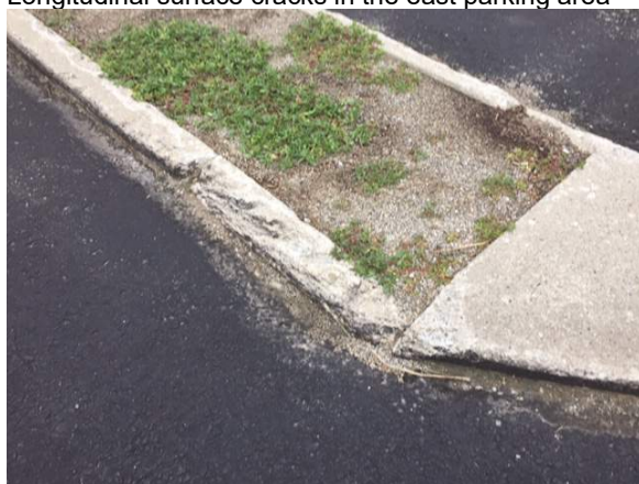
Area of deterioration on concrete curb
