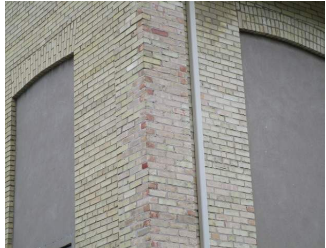
Previous brick masonry repairs – 1920 Building
