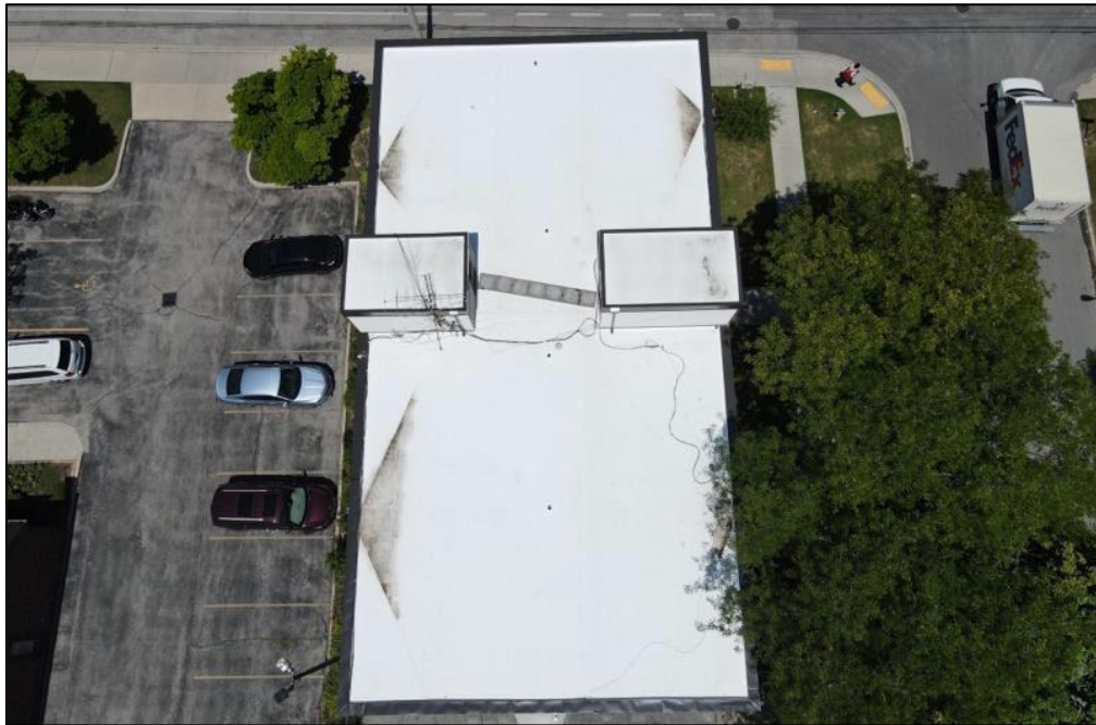
5.36.1.1.1.1.2 Example of recent TPO project.
