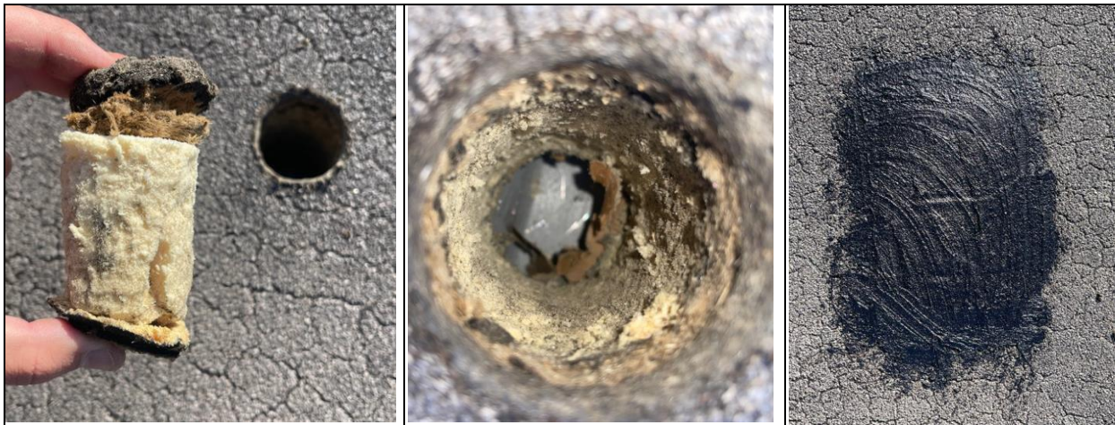
Core Cut of Roof System
