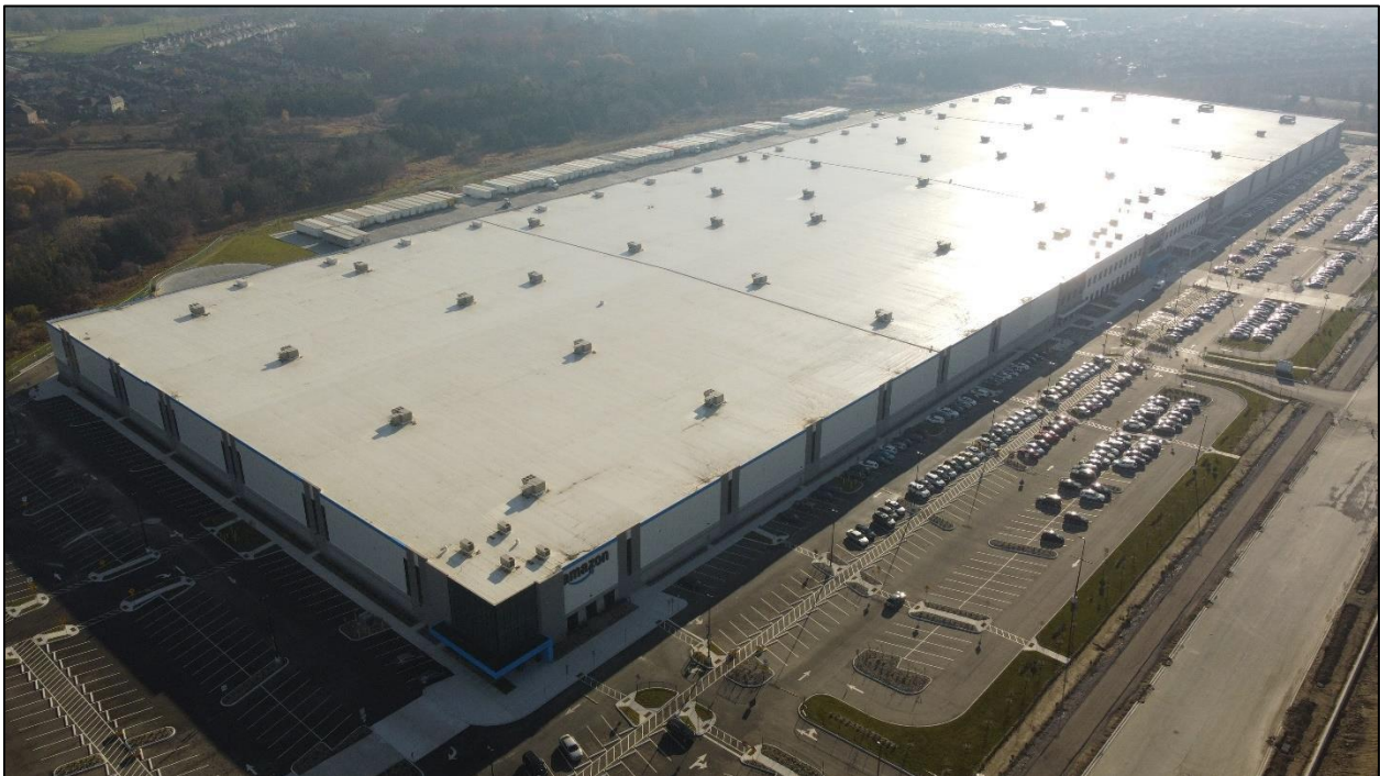
5.36.2.1.1.1.4 Recently Completed TPO Project
