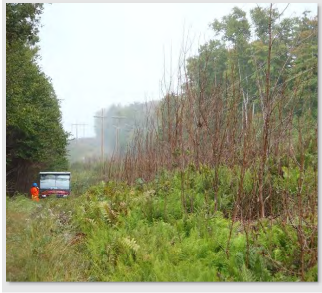
Figure 9: Herbicide Treatment – show a decrease in biomass (tall vegetation) converting ROW to compatible vegetation
