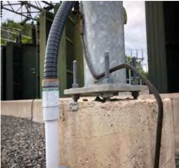
Detached and degraded foundations (left and right picture)
