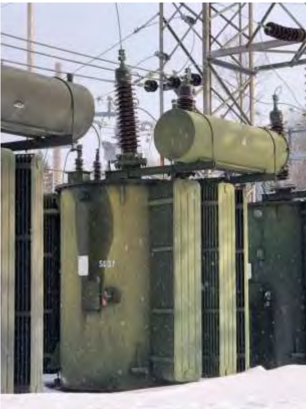
Goulais T1 with signs of oil leak
