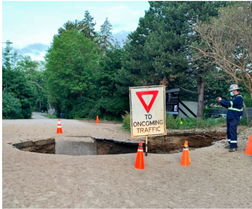
Figure 16: Pipeline Failure on NPS20 Distribution Main Operating at 175psi – Detailed
