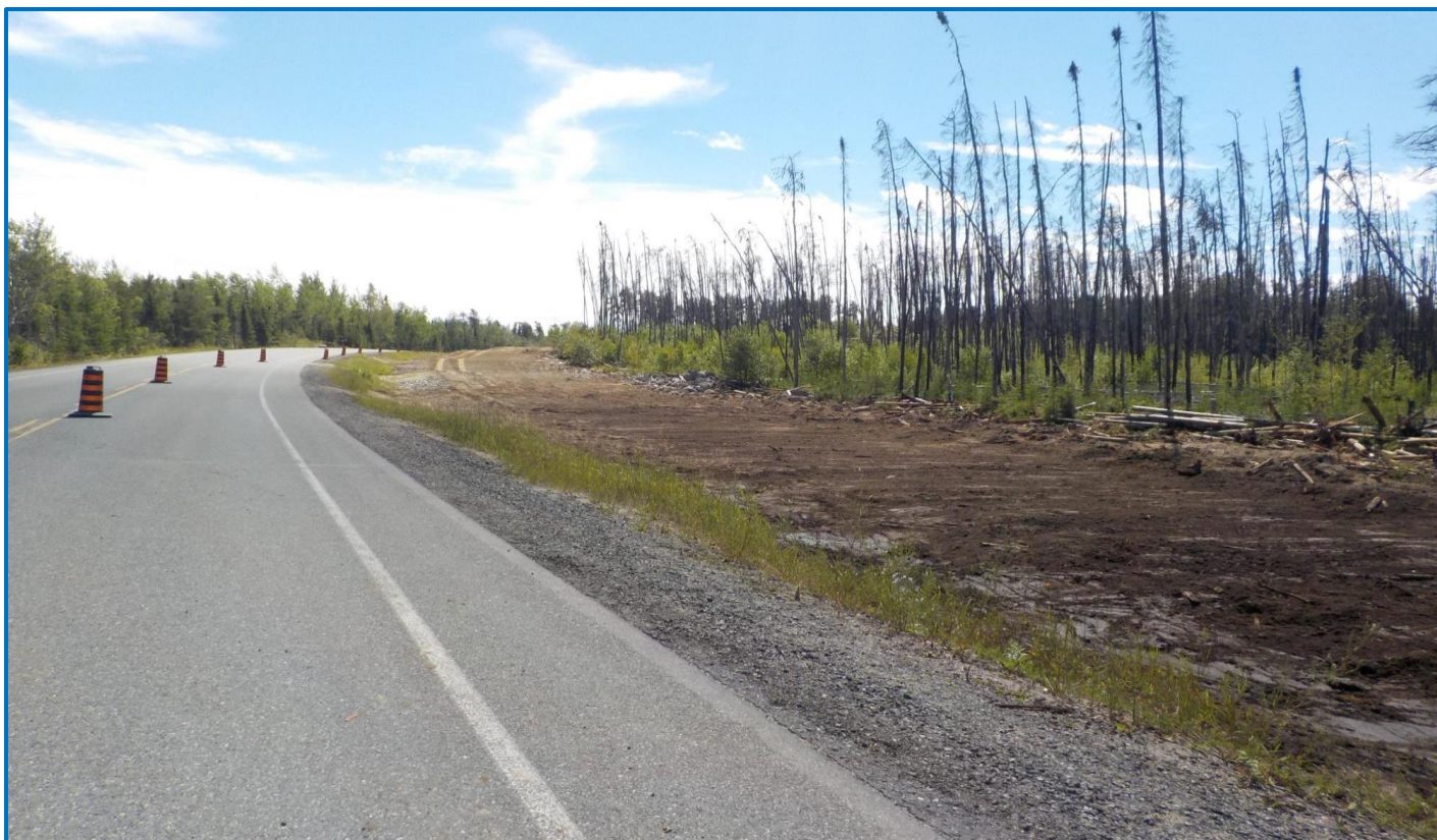
1. Following construction, the right-of-way was graded to as close to the original as possible and seeded.
