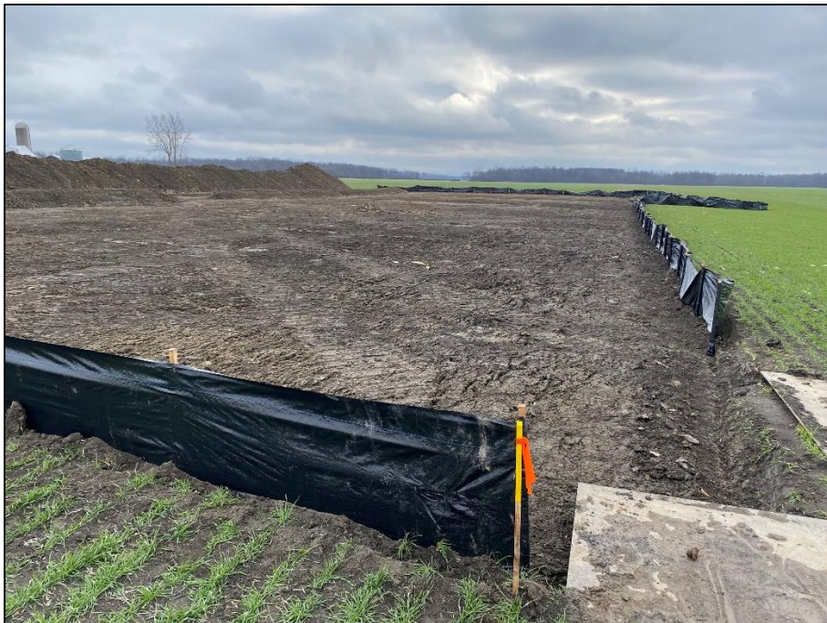
Photo 4 – Erosion and Sediment Control installed around the site.
