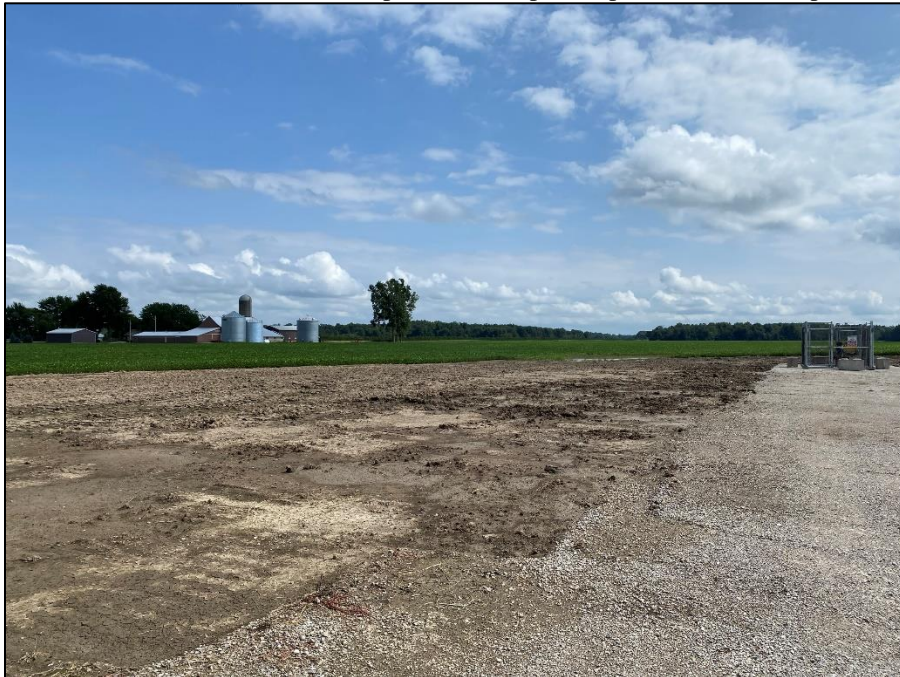
Photo 8 – Restoration of site is completed with topsoil replaced and de-compacted.
