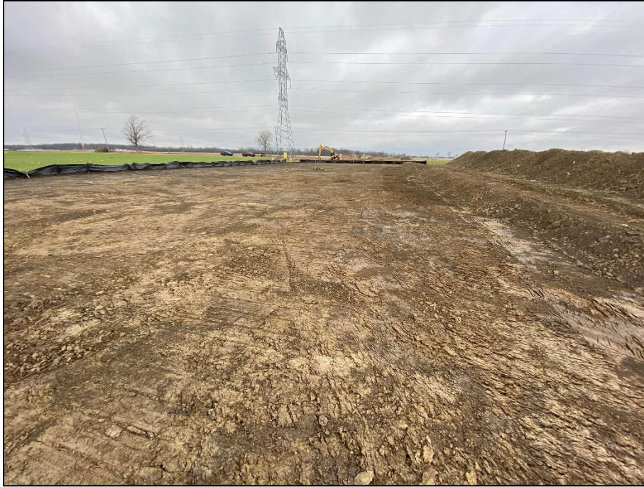
Photo 3 – Topsoil stripping and storage.
