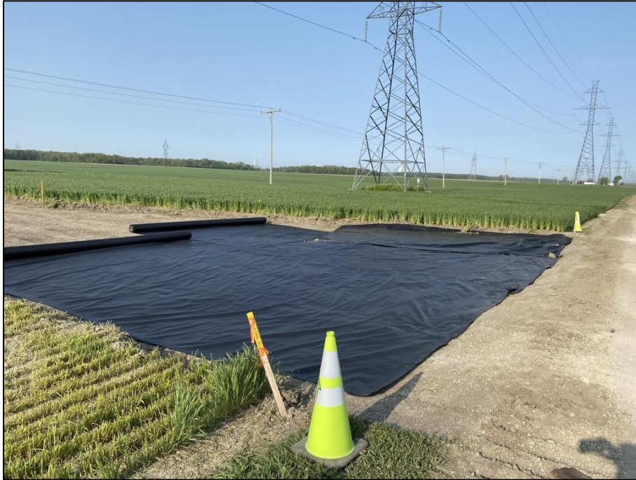
Photo 5 – Geotechnical fabric being placed on subsoil to separate granular pad.
