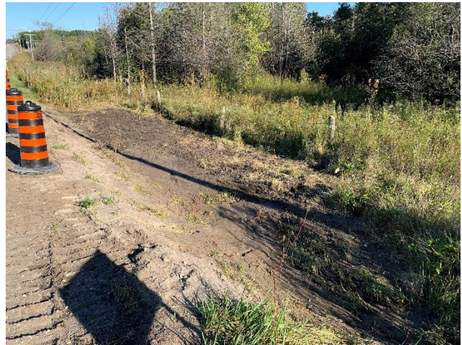
Photo 16: Backfilling completed at the entrance pit for the HDD crossing of Leaksdale Creek (September 26, 2024).
