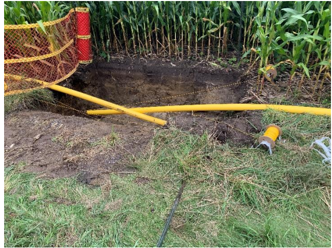
Photo 2: Tie-in pit within Concession 8 road ROW ditch. Tie-in pits were minimized in disturbance across the Project where possible (August 19, 2024).
