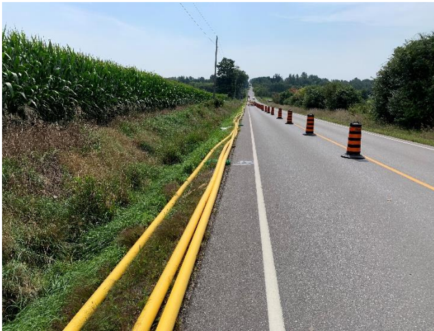
Photo 3: Mainline pipeline strung along road embankment within the Concession 6 road ROW (August 27, 2024).
