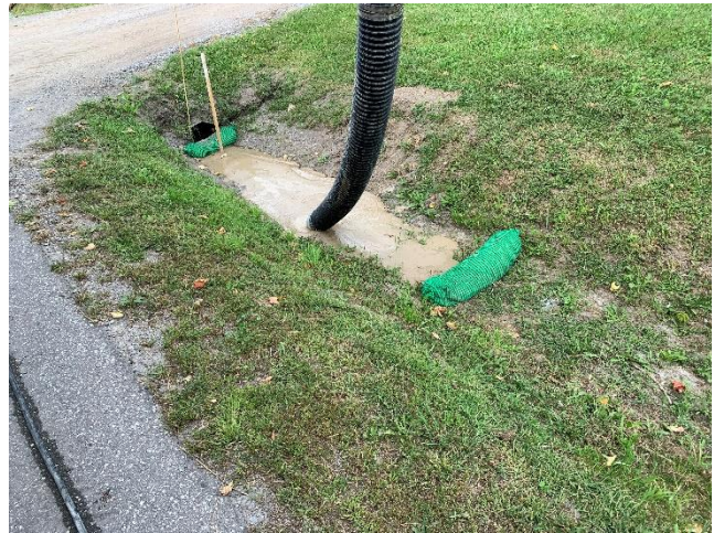
Photo 4: Small inadvertent release of drilling fluid within the ROW immediately isolated and cleaned-up along the Concession 6 road ROW ditch (August 29, 2024).
