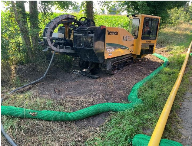
Photo 1: HDD drill rig staged and drilling within the Concession 6 road ROW ditch. Silt sock established around drill rig during drilling to prevent off-site release of drilling mud (August 16, 2024).
