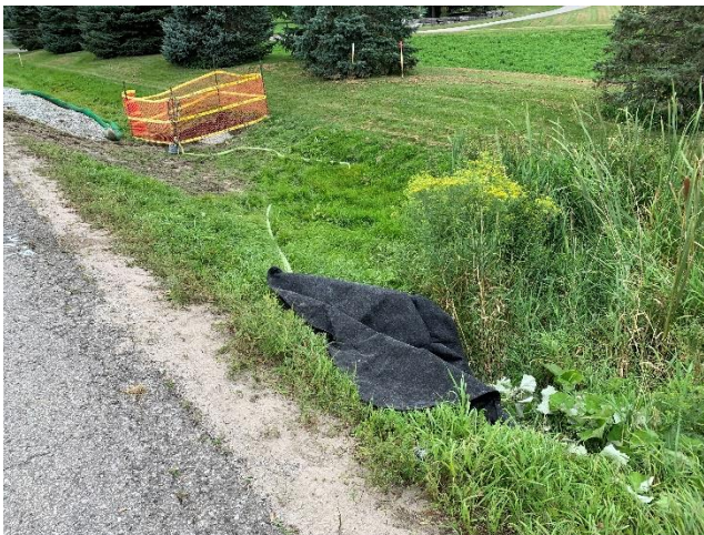
Photo 5: Established de-watering through a filter bag at tie-in pit on Ball Road (August 29, 2024).
