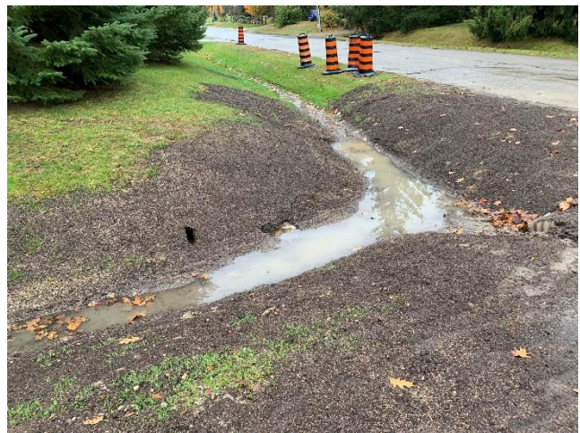
Photo 24: Water ponding after restoration at the corner of Smith Drive and James Place in the Village of Sandford (October 29, 2024).
