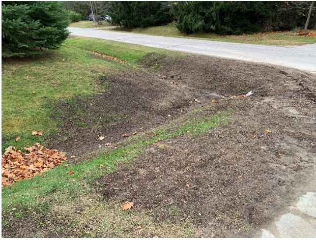
Photo 25: Regrading of restored area at the corner of Smith Drive and James Place in the Village of Sanford to address water ponding observed in Photo 24 (November 14, 2024).
