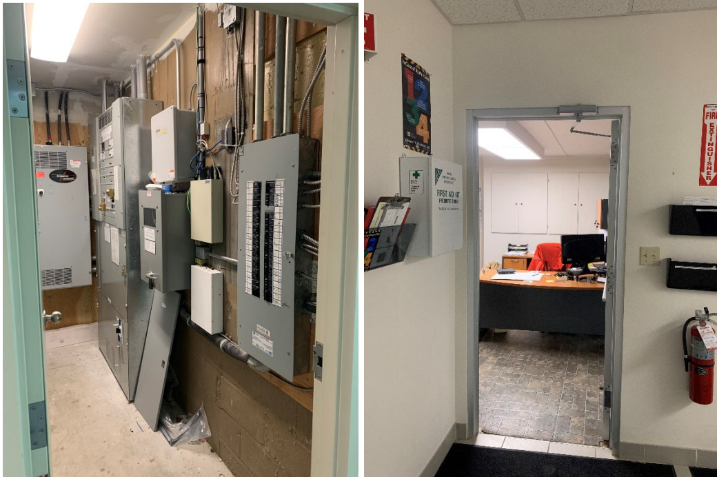
Figure 4 – Electrical Rooms – 3 phase service is located behind cupboard doors in this office
