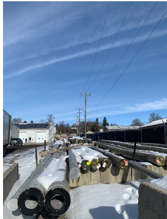
Figure 3.1 – Pole Bunk directly under 27.6kv
