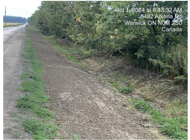
Photo 20 Shoulder of road where hydroseeding had been applied. Additional monitoring for germination may be required in 2025.
