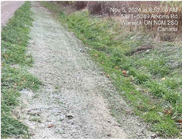
Photo 25 East side road shoulder on Arkona Rd. requiring additional hydroseeding and will be addressed in spring of 2025.
