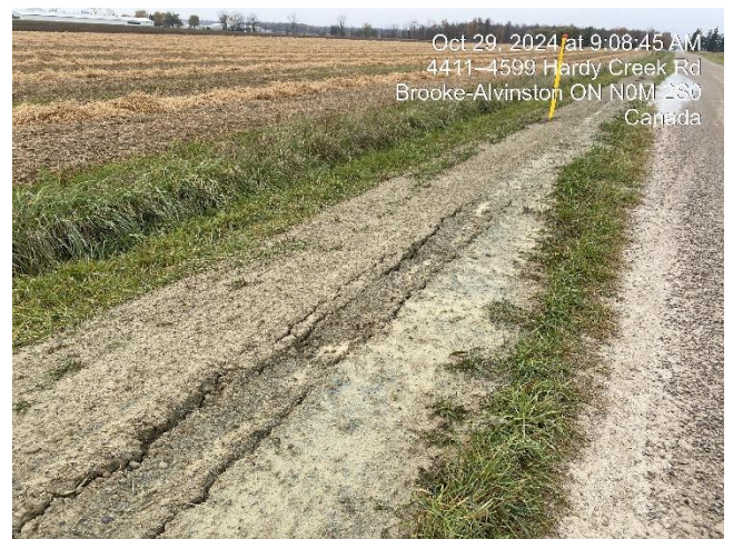
Photo 24 Settling observed along specific locations within ROW. Additional monitoring will be required in spring of 2025.
