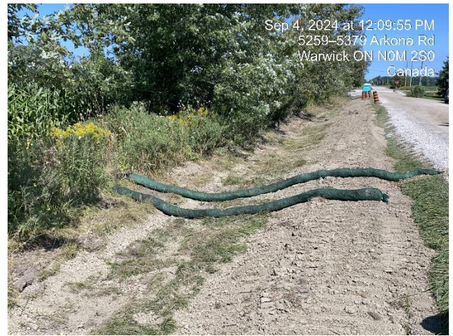
Photo 14 Temporary placement of sediment sock for use as a checkdam while hydroseeding is completed.
