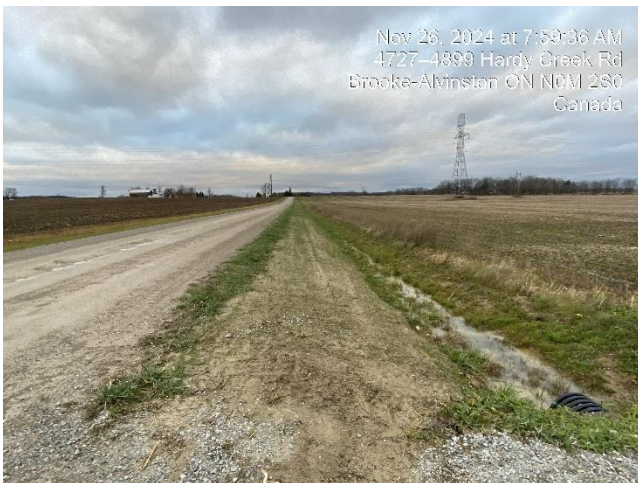
Photo 35 Minimal germination observed on shoulder of road. Additional application may be required in spring 2025.
