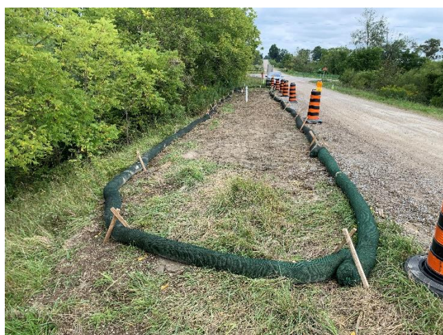
Photo 11 Installation of sediment sock to isolate recent restorative measures.
