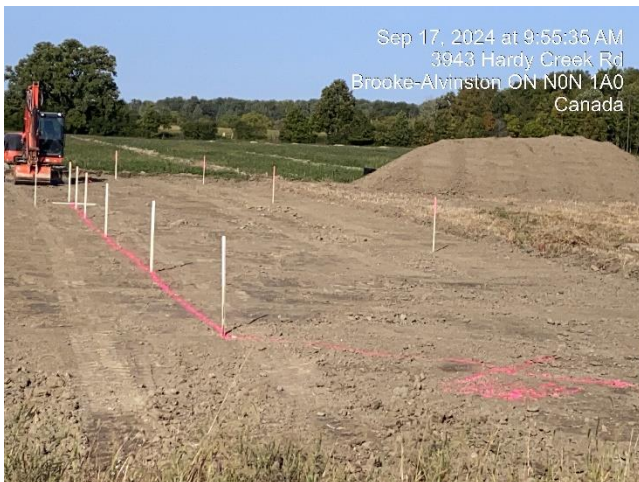
Photo 17 Topsoil stripping and soil isolation at Enbridge Gas mainline block valve station.
