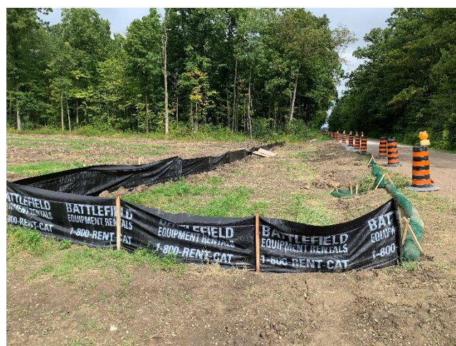
Photo 12 Installation of sediment fencing and sediment sock prior to construction of dewatering basin.
