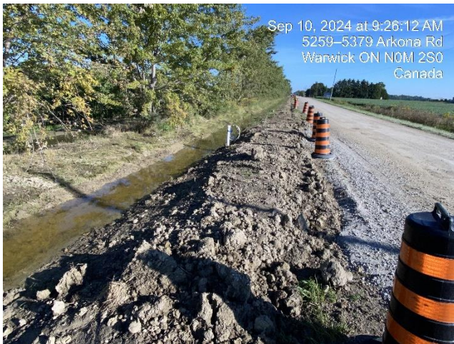
Photo 15 Crowning of subsoil to address with future settling.
