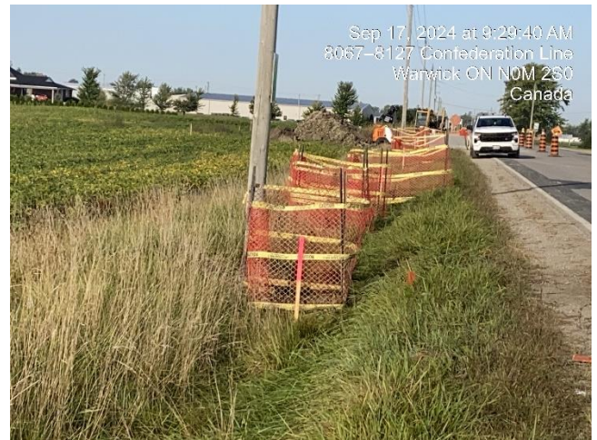
Photo 16 Monitoring pits isolated awaiting backfilling on Confederation Line.
