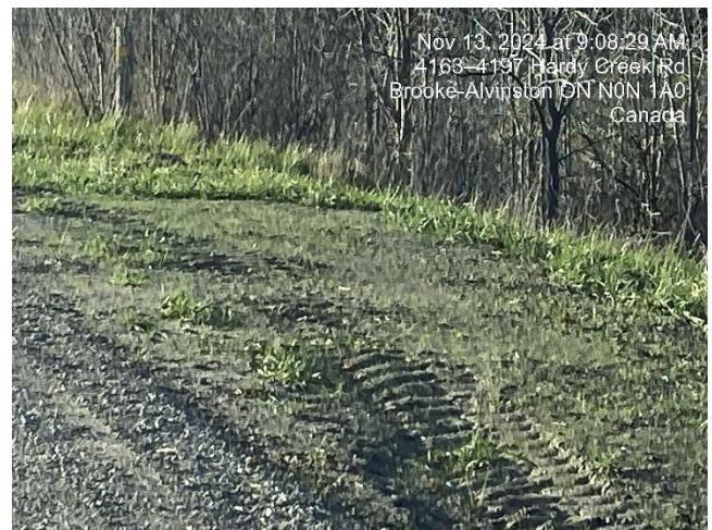
Photo 28 Minimal germination evident on shoulder of road. Recent settling may require additional topsoil and seeding in the spring 2025.
