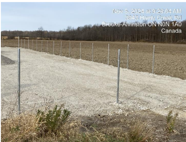
Photo 27 Completion of gravel pad and security fencing at Enbridge Gas mainline block station.
