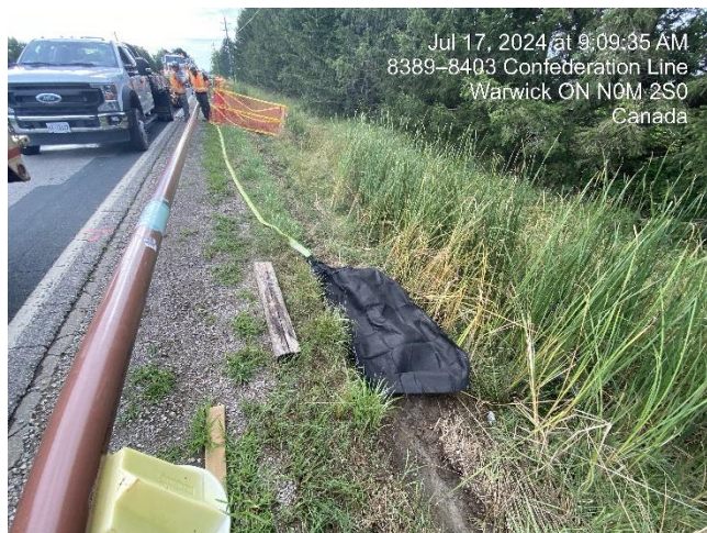
Photo 7 Utilization of sediment bag during dewatering activities after rain event.
