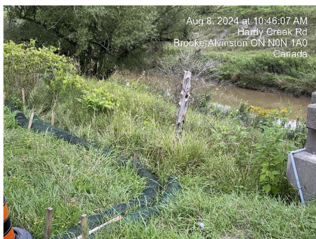
Photo 9 Preemptive installation of sediment sock on the south side of Hardy Creek at 30-m setback.
