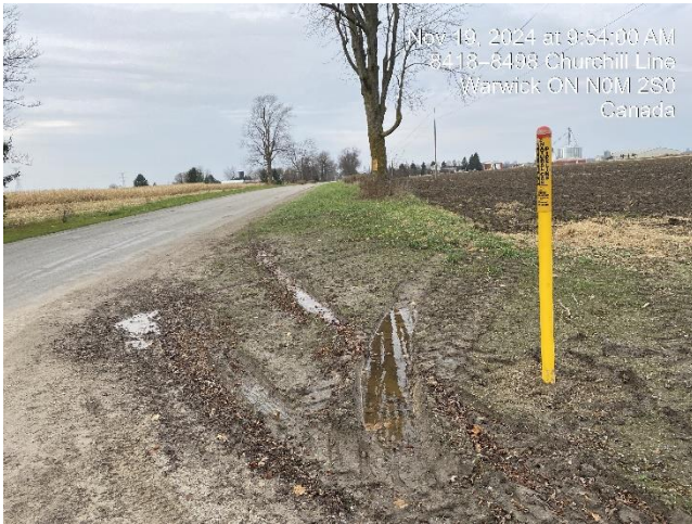
Photo 31 Additional topsoil required. Issue will be monitored and addressed in spring 2025.
