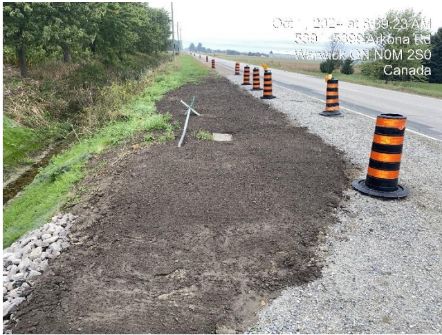
Photo 19 Topsoil placement and final grading at corner of Confederation Line and Arkona Rd.
