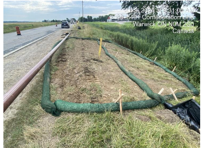
Photo 6 Typical installation of sediment socks to isolate restored shoulder of road after restoration of the ROW.
