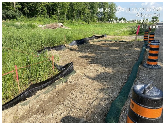
Photo 8 Installation of sediment fencing (with sediment sock) to isolate restored shoulder of Arkona Rd. after work had been completed.
