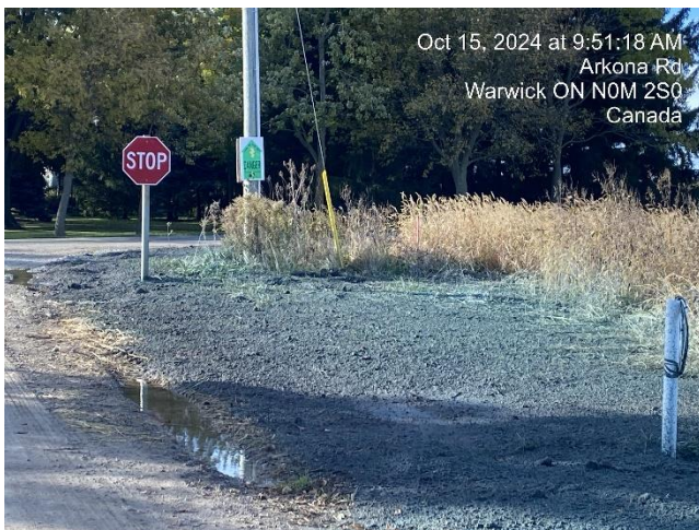
Photo 23 Restored corner of Arkona Rd. with topsoil and hydroseeding applied.
