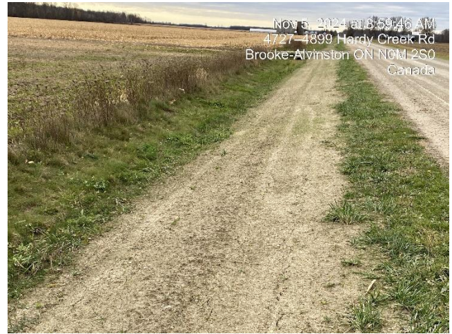
Photo 146 East side shoulder of Hardy Creek Rd. Additional hydroseeding may be required in spring of 2025.
