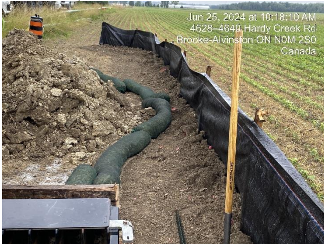
Photo 5 Standard ESC measures implemented to isolate stockpile prior to backfilling of trench.
