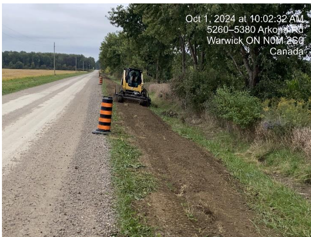
Photo 21 Prepping of shoulder in advance of topsoil placement and hydroseeding.
