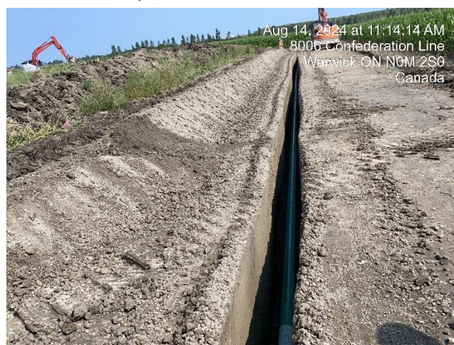
Photo 10 Open cut trenching leading towards Twin Creeks Environmental Centre.
