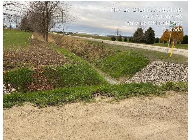
Photo 32 Completed and stabilized roadside ditch.
