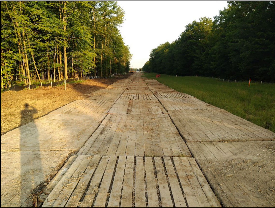
5. Access matting was utilized to minimize disturbance in more natural areas of the ROW.
