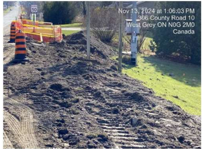
Photo 20 Restorative measures outstanding attie in pit. Grading and stabilization to occur in spring 2025.
