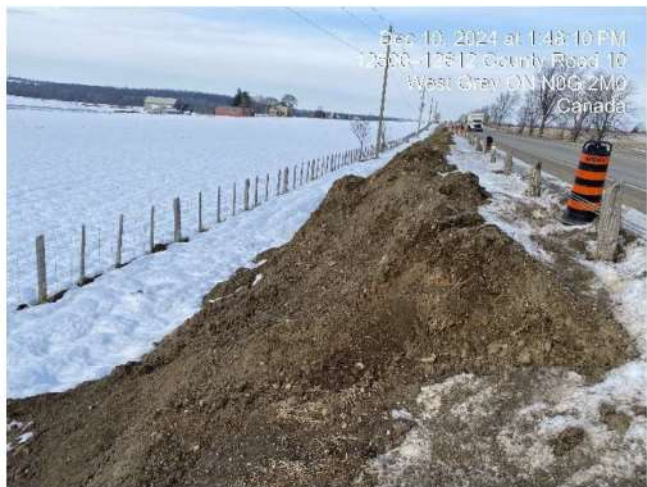
Photo 28 Shoulder of road where rough grading was unable to be completed. Restorative measures to be completed in spring of 2025.
