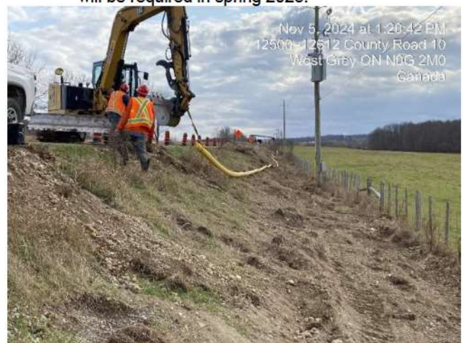
Photo 18 Open cut installation in ROW.
