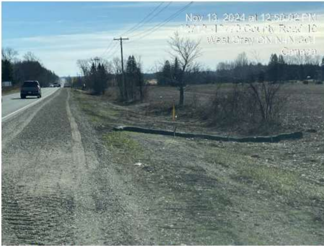
Photo 19 Finished grading and utilization of sediment sock to prevent off-site sedimentation.
