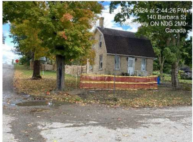
Photo 12 CHR where vibration monitoring occurred.
