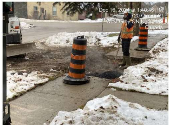
Photo 36 Sidewalk repairs are ongoing on Queen Street
