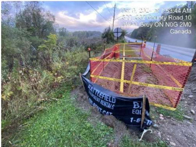
Photo 11 Tie in pit secured with ESC measures as per EPP.
