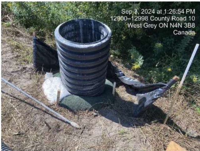
Photo 3 Relief pit with appropriate mitigation measures in place.
