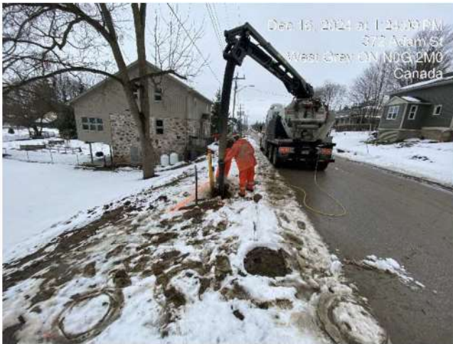
Photo 33 Daylighting on Adams Street.
