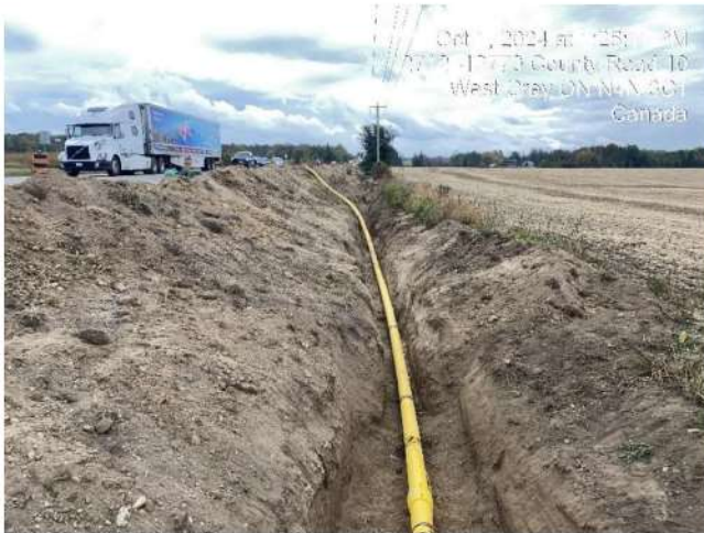
Photo 9 Open cut trench installations were backfilled at end of each day.
