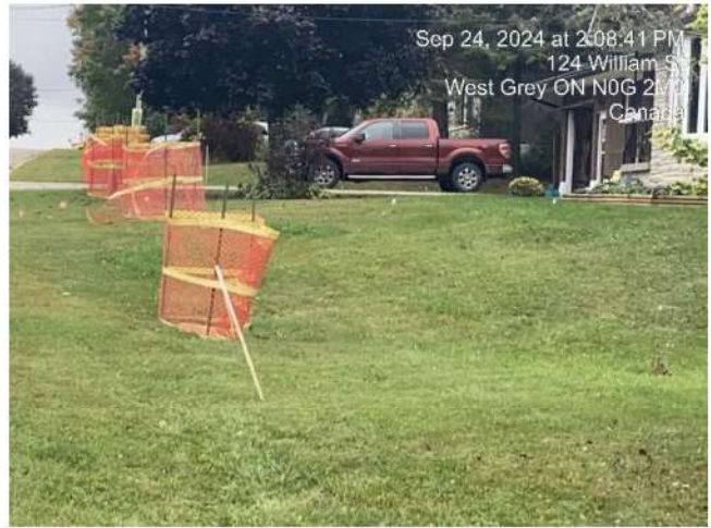
Photo 8 Utility sight holes surrounded by protective fencing in municipality.
