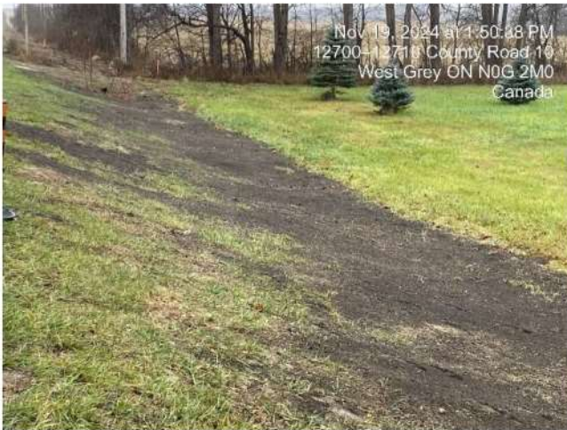
Photo 21 Restored roadside shoulder with topsoil and broadcast seeding.
