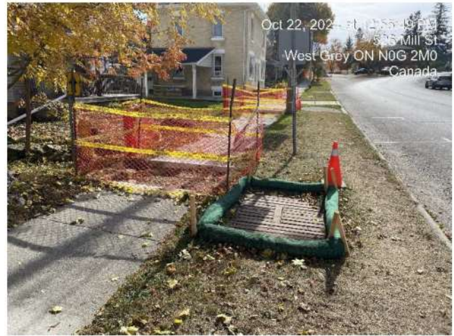
Photo 14 Pre-emptive ESC mitigation measures at catch basins within community of Neustadt.
