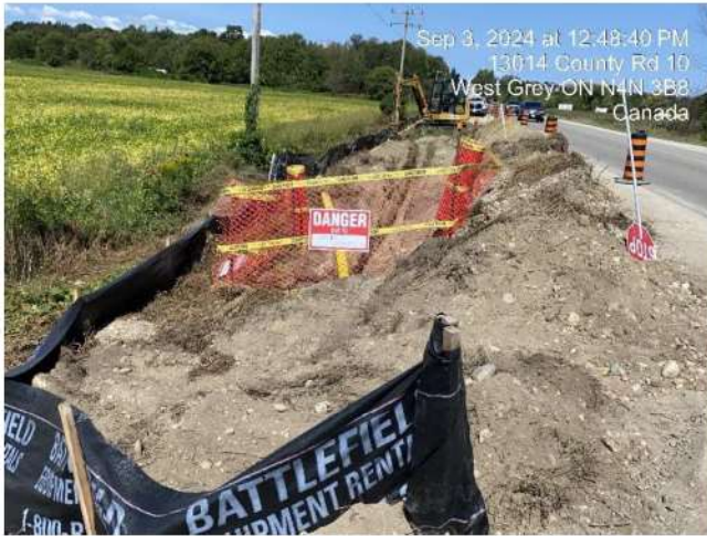
Photo 1 Isolation of ROW and tie in pits with ESC fencing.
