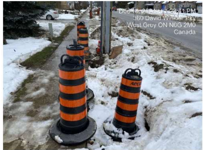
Photo 34 Final restoration is hampered due to recent weather events.
