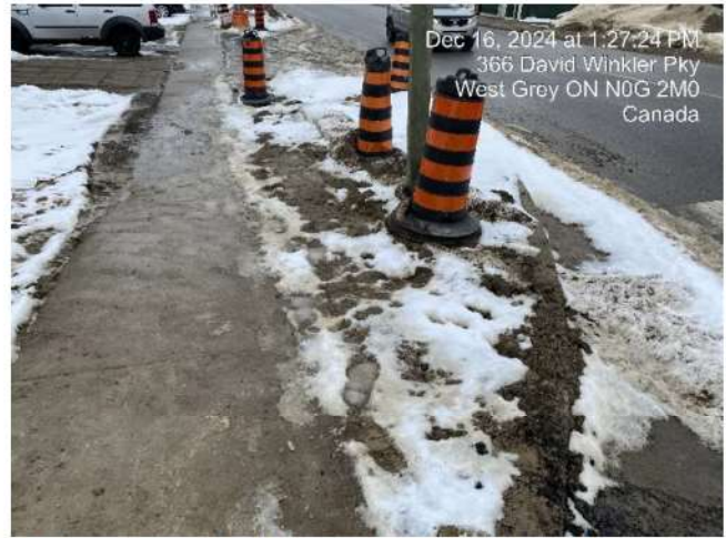
Photo 32 Settling and final restoration to be completed
