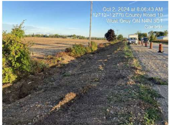
Photo 10 Completion of backfilling open cut trench on shoulder of road.
