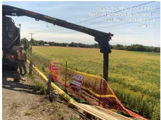
Photo 4 Hydro-vac on site to assist with HDD activities.
