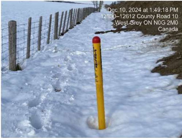
Photo 31 Pipeline location marker in place.
