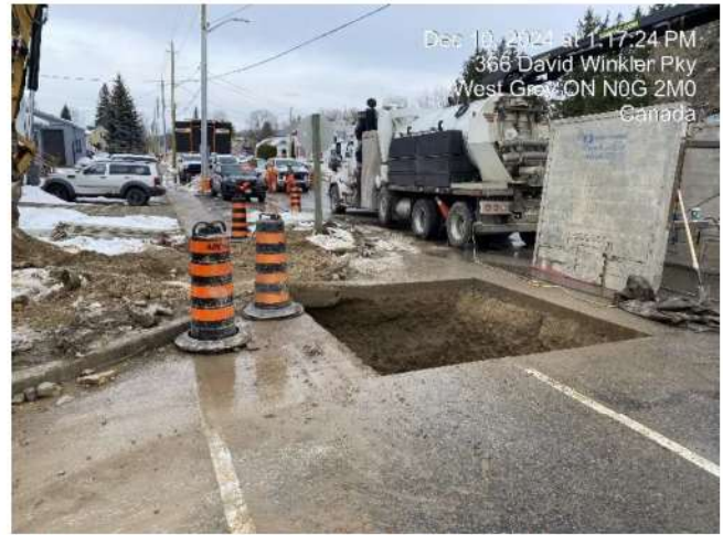
Photo 26 Tie in pit located in road intersection.
