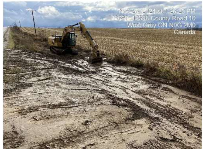
Photo 24 Grading of roadside shoulder.
