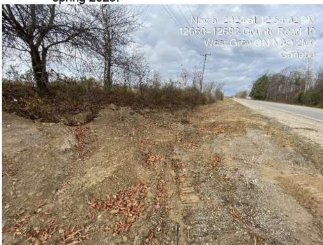
Photo 17 Rough grading after backfilling of open cut trench.
