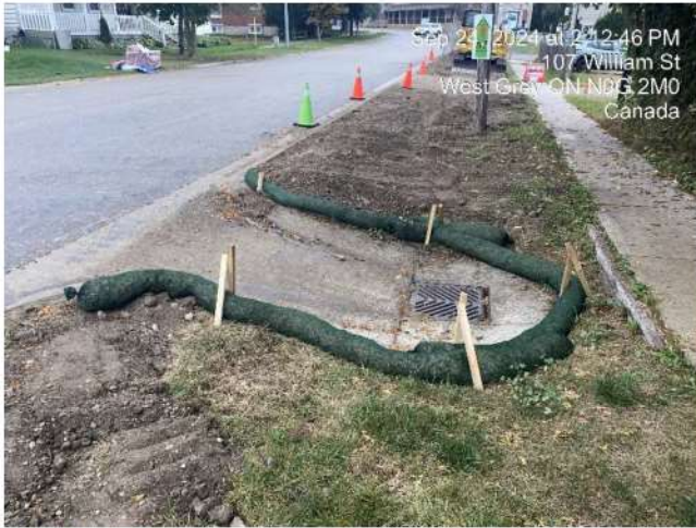
Photo 7 ESC mitigation in place around storm basin in municipality.
