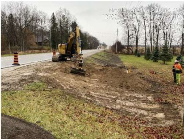
Photo 23 Final grading along roadside shoulders.
