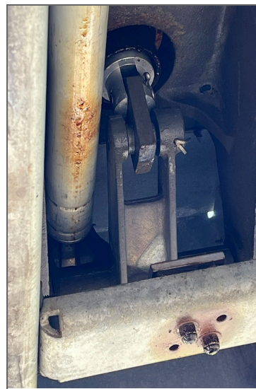
(b) Switching equipment lubrication leaks
