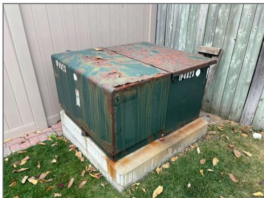
(a) Underground transformer corrosion
