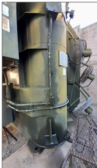
(a) Station transformer corrosion and leaks
