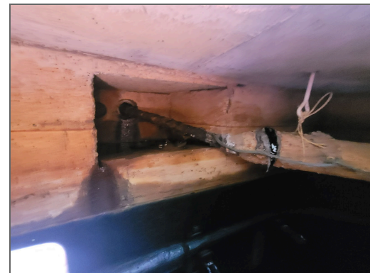
(b) Underground cable failure
