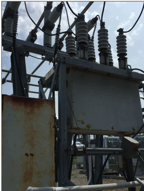
(e) Station outdoor infrastructure deterioration
