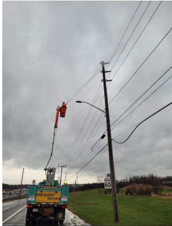
Figure 6: Burlington Hydro's Contractor Performing Insulator Washing
