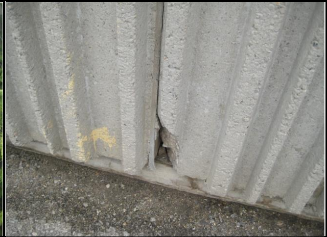
Photo #52: Damaged Precast Panels
