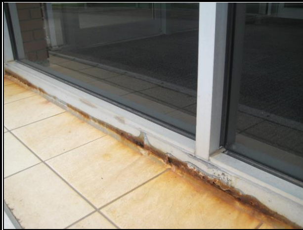
Photo #57: Corroded Metal Flashing at bottom of Window
