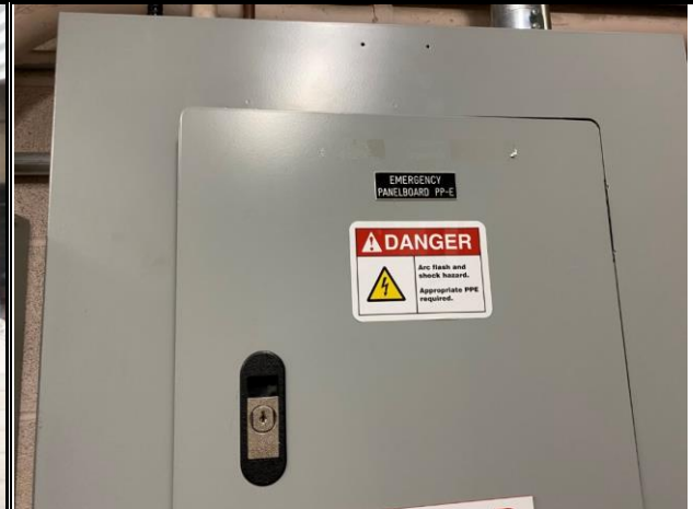
Photo #98: Emergency Panel Board
