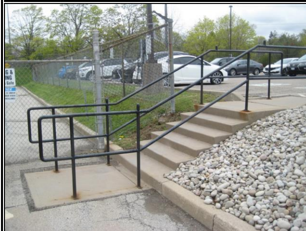
Photo #117: Corroded Metal Railings at Concrete Stairs
