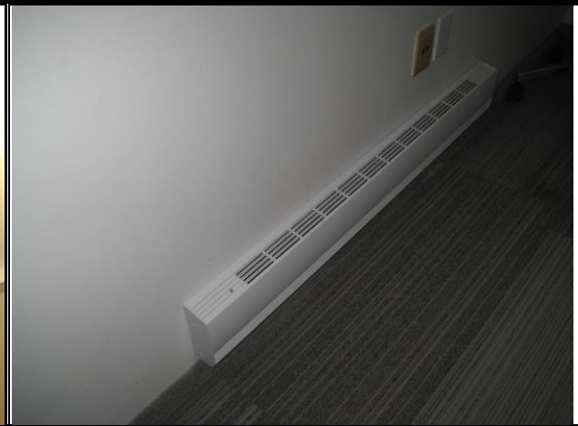
Photo #76: Electric Baseboard Heater
