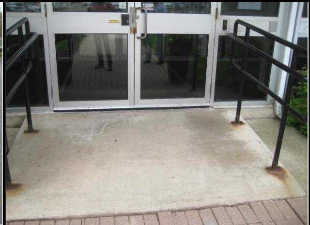
Photo #116: Corroded Metal Railings at Secondary Entrance
