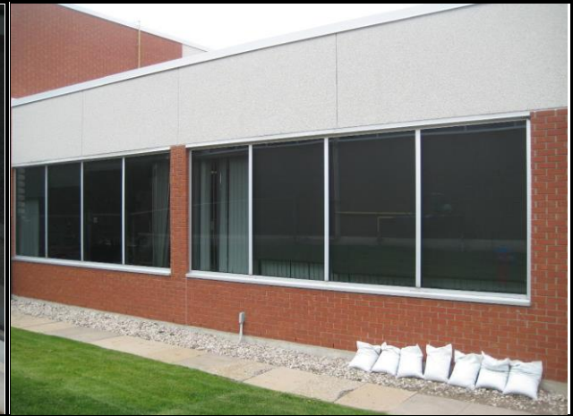
Photo #58: Typical Office Addition Aluminum Window
