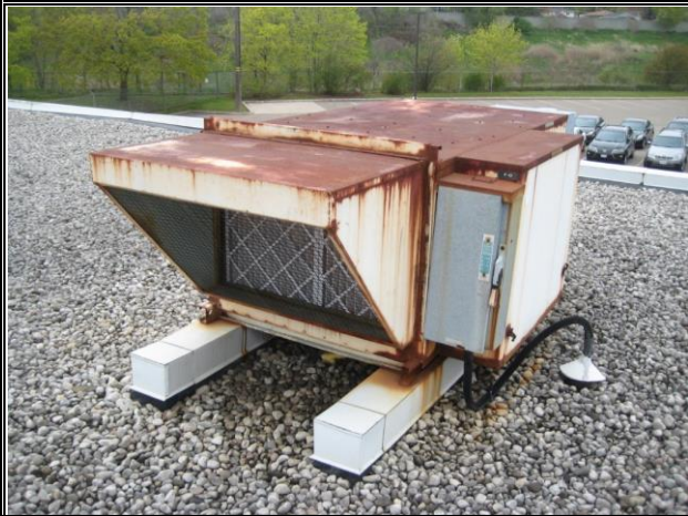
Photo #72: Decommissioned Roof Top Unit
