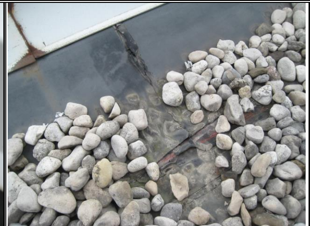
Photo #30: Corroded Metal Capping and Thorn Seam
