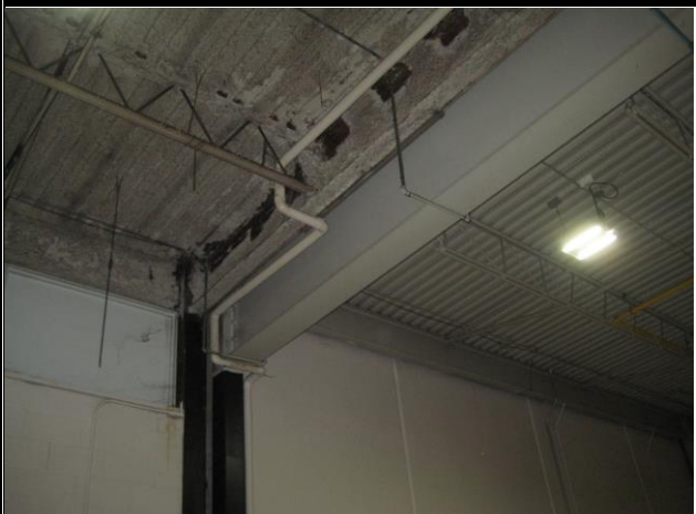
Photo #8: Expansion Joint between Original Service Centre and Addition
