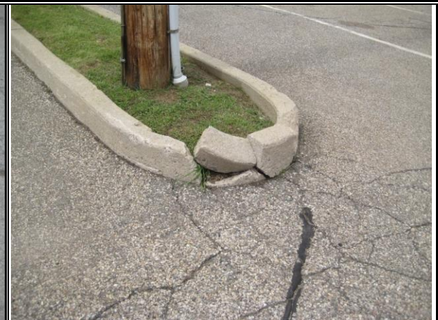
Photo #104: Damaged Concrete Curb
