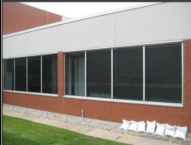
Photo #53: Exposed Aggregate Panels at Office Addition
