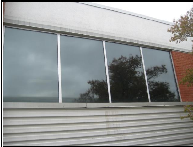
Photo #47: Stained Metal Cladding at Office Building
