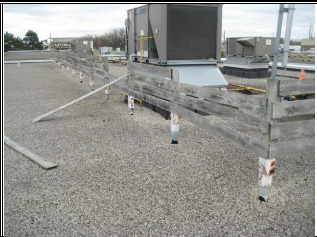
Photo #18: Deteriorated Roof Screen
