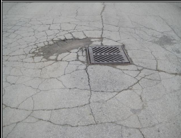
Photo #103: Asphalt Pavement Settlement at Catchbasin
