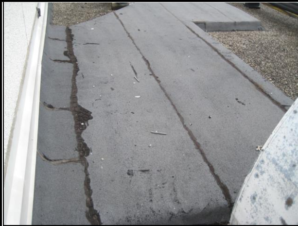
Photo #25: Mod-Bit Roofing at South Link
