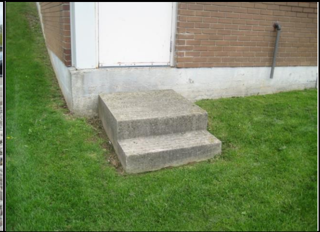
Photo #110: Precast Concrete Steps at Stockroom Exit Door
