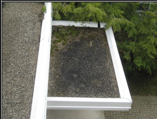
Photo #23: Vegetation Growth at Secondary Entrance Low Roof
