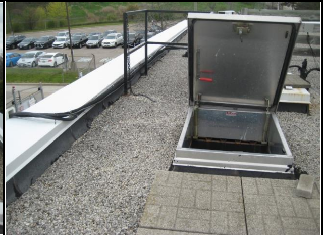
Photo #20: Roof Access Hatch less than 6 feet from Roof Edge
