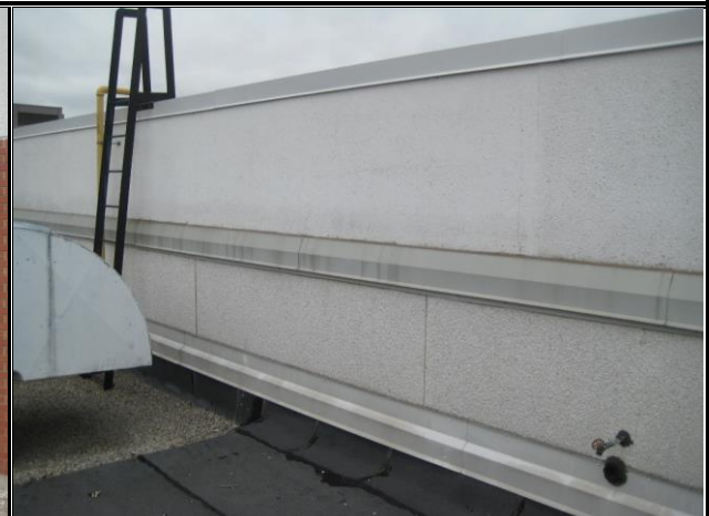
Photo #54: Exposed Aggregate Panels at Office Original Building
