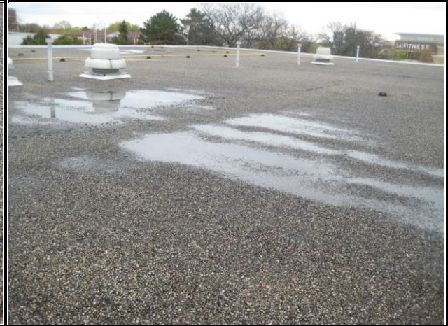
Photo #28: Water Ponding
