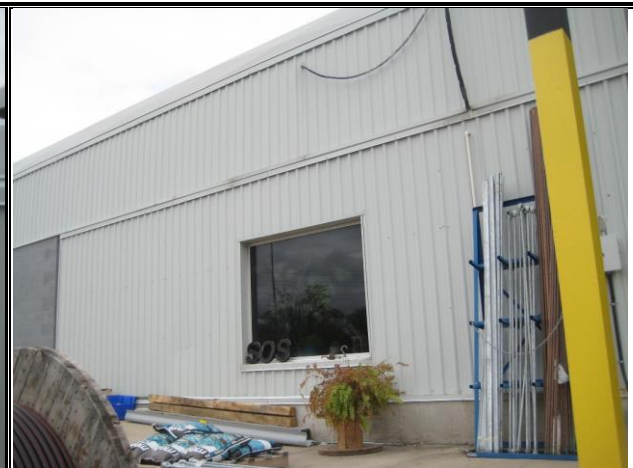
Photo #46: Service Centre Metal Cladding
