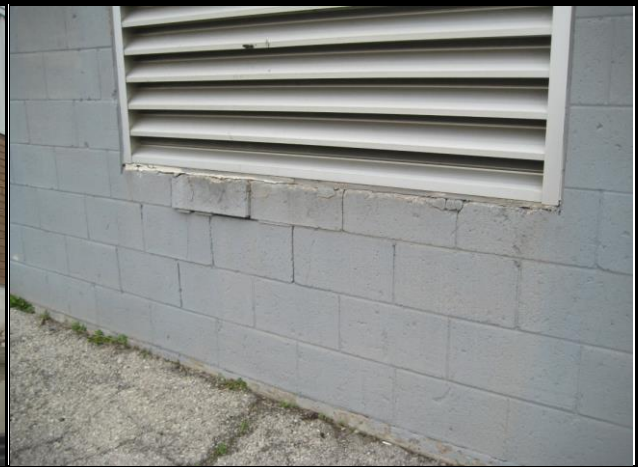
Photo #44: Loose Concrete Block Units below Mechanical Louvre
