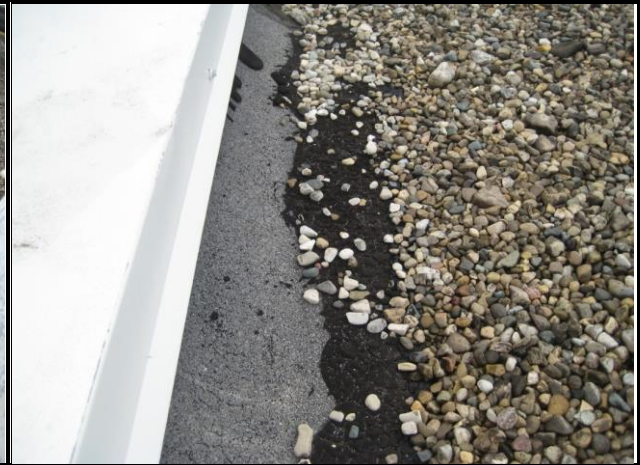
Photo #26: Mod-Bit Upturn at Parapet
