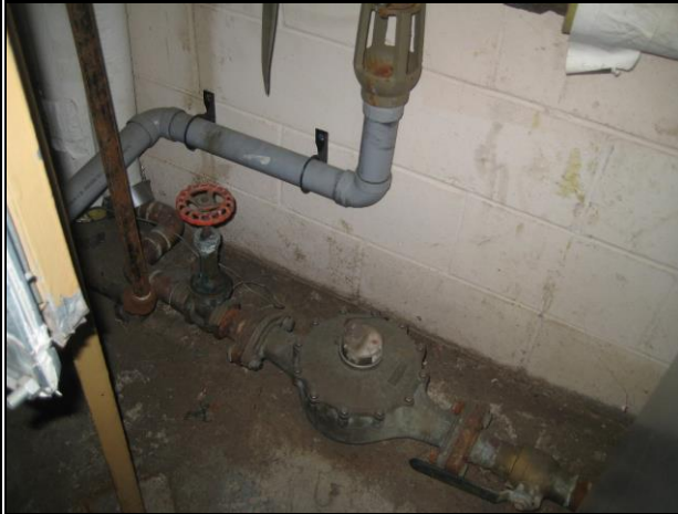
Photo #79: Domestic Water Supply and Meter
