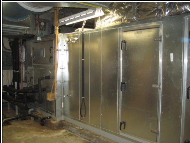
Photo #73: Basement Air-Handling Unit
