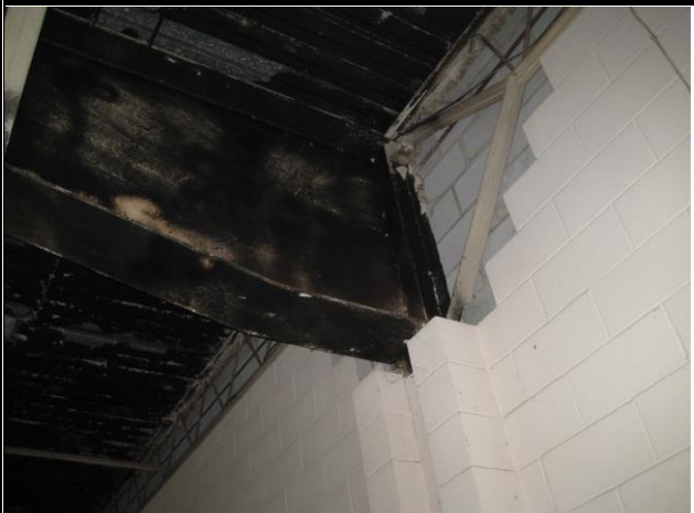
Photo #6: Stockroom Steel Beam Supported by Column
