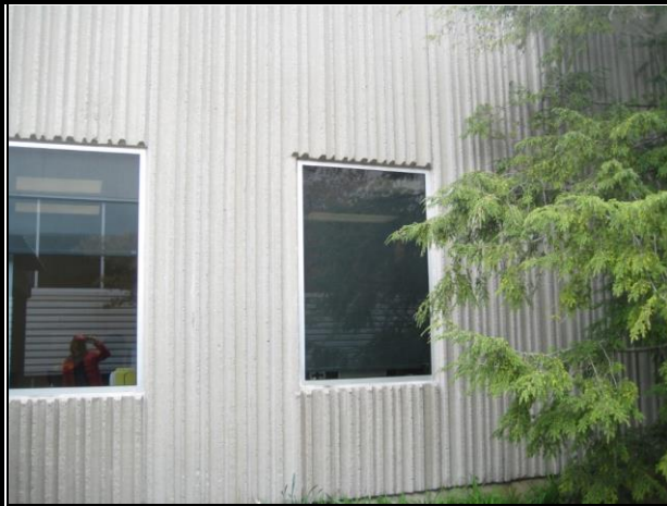
Photo #51: Precast Panels at Service Centre Windows
