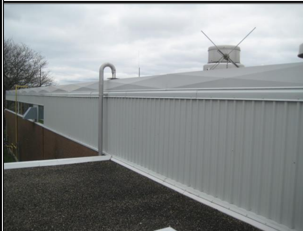
Photo #45: Service Centre Upper Wall Metal Cladding
