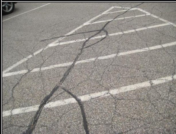
Photo #101: Cracked Asphalt Pavement
