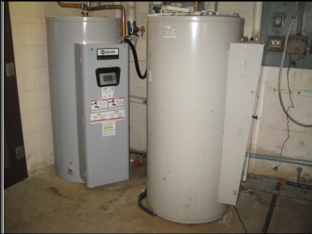
Photo #80: Domestic Water Heaters
