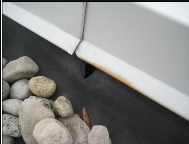
Photo #29: Ripped EPDM Membrane at Service Centre Addition Roof
