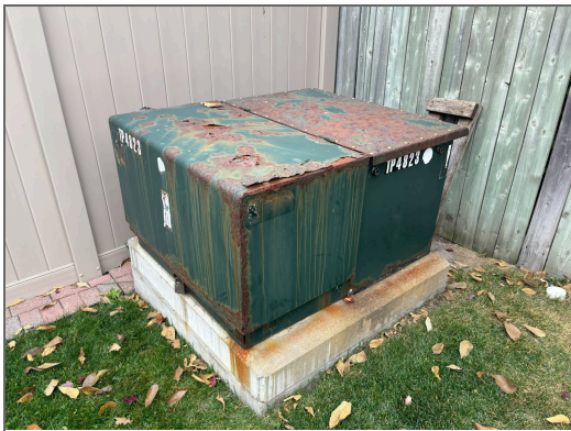
(a) Underground transformer corrosion
