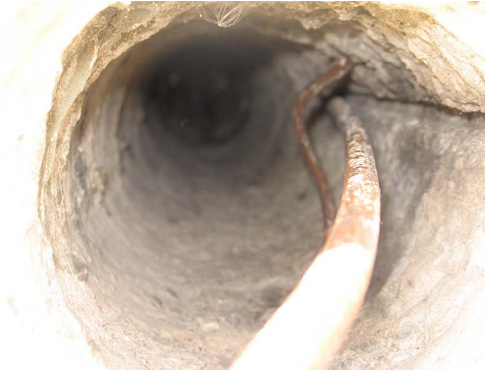
Figure 4: Rusted rebar - close to the rebar support tie
