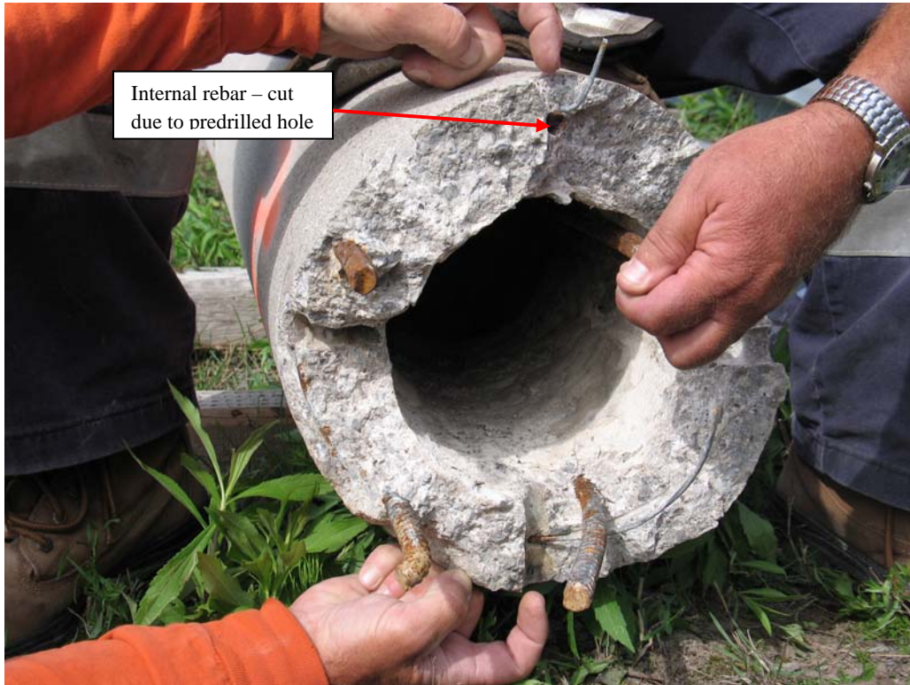
Figure 2: predrilled hole provided by the manufacturer - cutting one of the internal rebar
