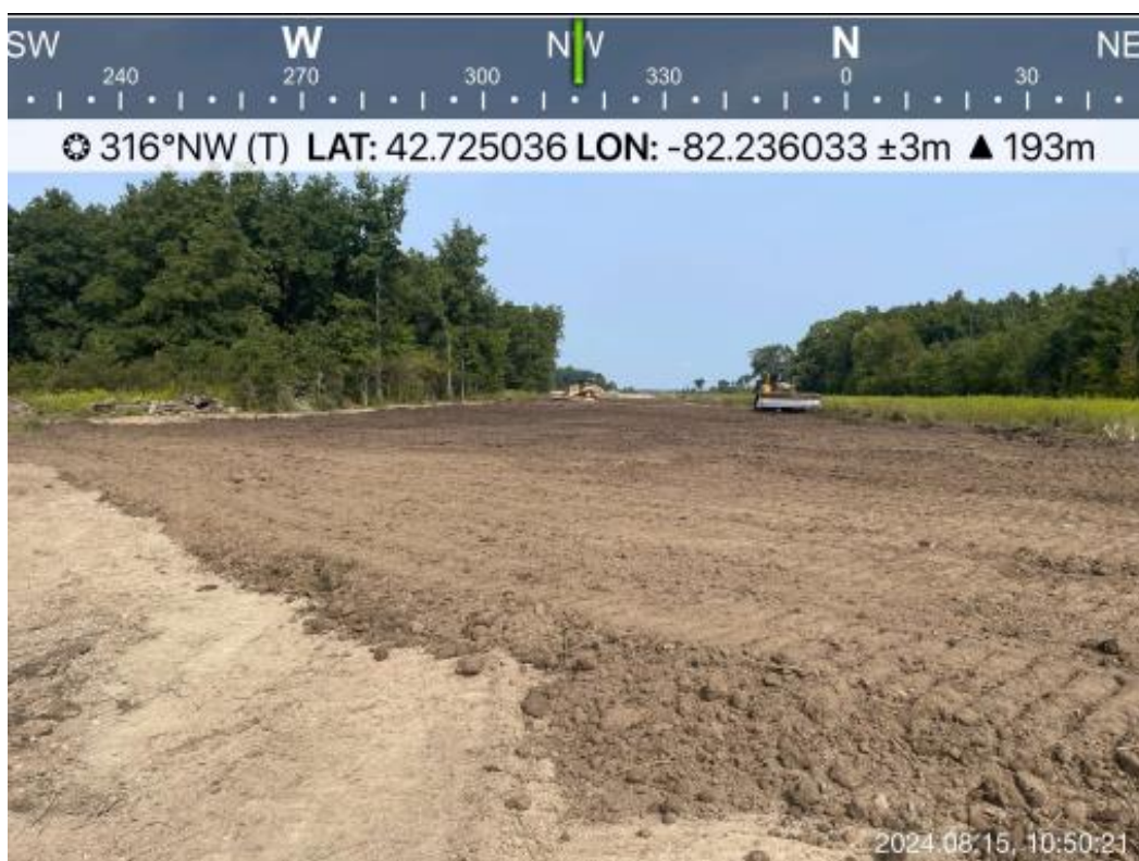
11. Spreading and leveling topsoil
