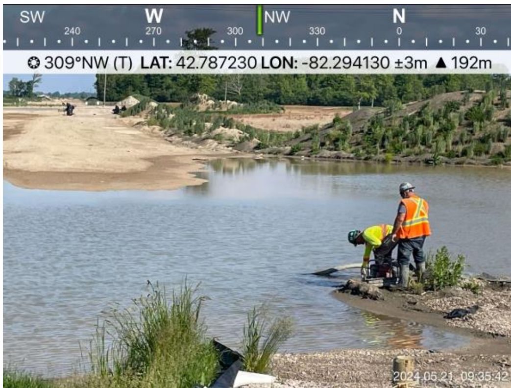
4. Pumping ponded easement to dry soils prior to restoration.
