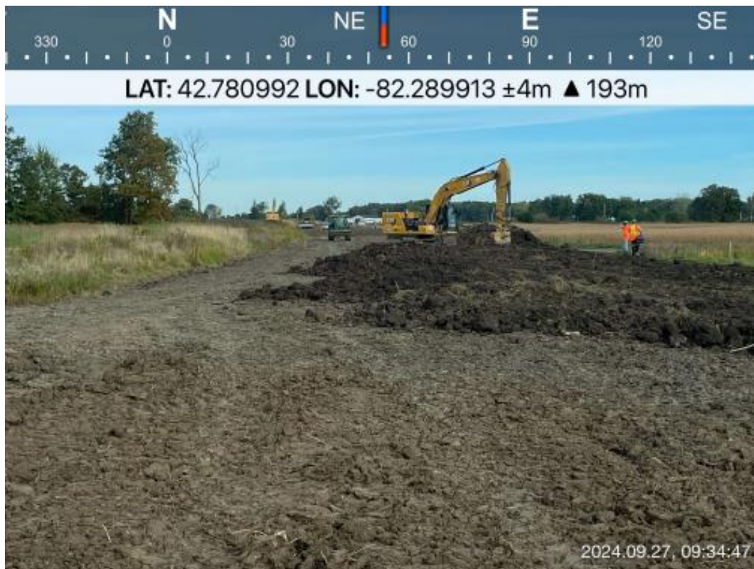
12. Pulling topsoil and casting it across easement to dry prior to spreading
