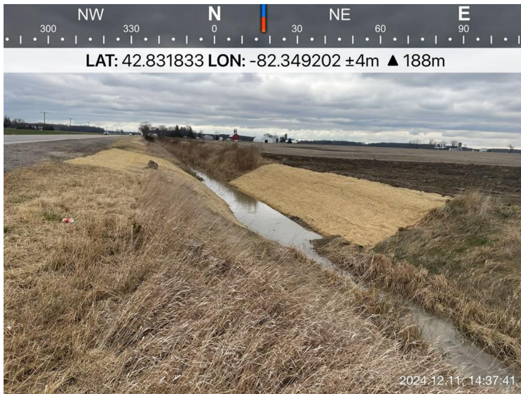
15. Drain restoration following removal of temporary culvert crossing.
