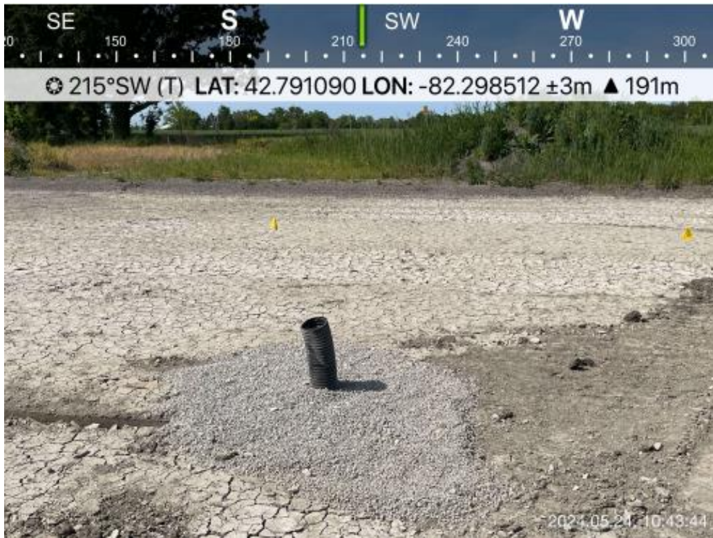
3. Completed French drain.
