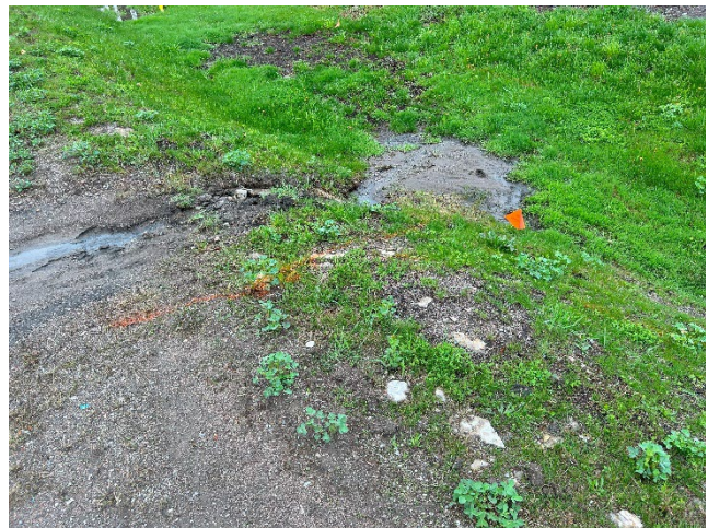
Photo 12: Some minor erosion occurring at swale outlet at the northwest corner of 8 th Line and Buckhorn Road (May 6, 2025).
