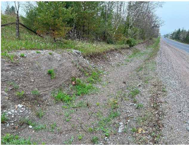
Photo 9: Stabilized rocky and sand road embankment adjacent to natural road embankment (May 6, 2025).
