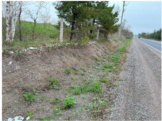
Photo 10: Stabilized gravel slope road embankment (May 6, 2025).
