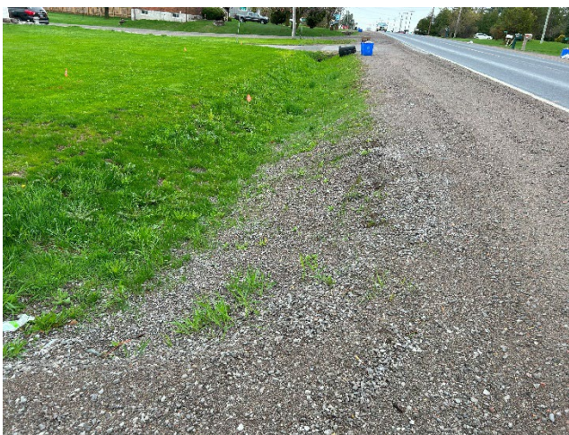
Photo 5: Restored ROW with some minor washout of gravel onto ROW from shoulders of 8 th Line (May 6, 2025).
