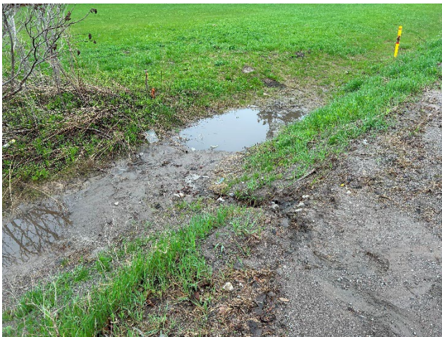
Photo 11: Some minor erosion occurring at swale outlet at the southwest corner of 8 th Line and Buckhorn Road (May 6, 2025).
