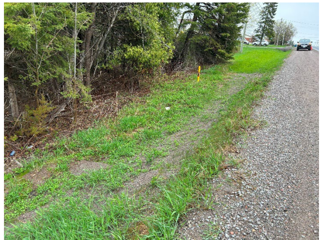
Photo 4: Washout of gravel onto ROW from shoulders of 8 th Line, West of Buckhorn Road (May 6, 2025).
