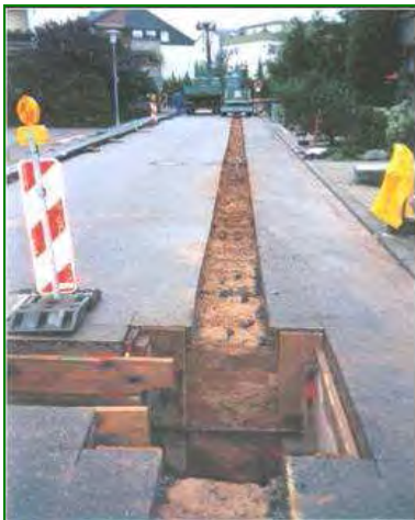
Figure 11.5 Laying District Heat Feeders in Mannheim
