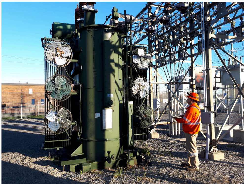
5 6 Figure 68 - Visual Inspection of a Station Transformer
