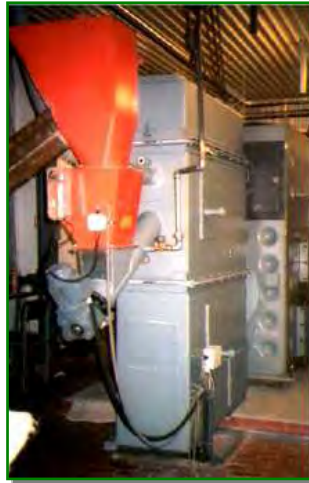
Figure 11.6 Typical Modern 1 MW (Thermal) Wood Boiler
