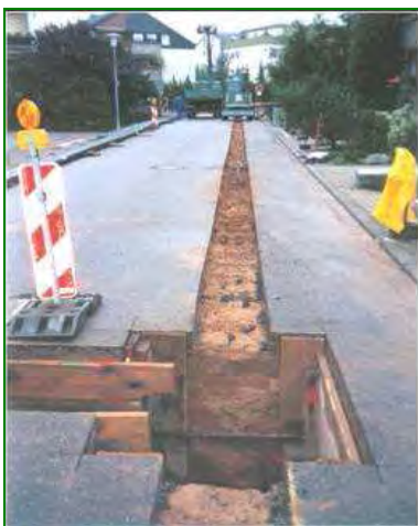
Figure 11.5 Laying District Heat Feeders in Mannheim
