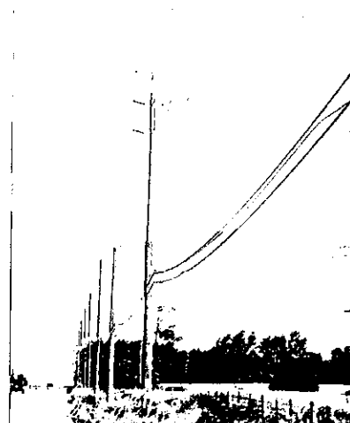
Pole Line to Connect Turbine Sites to Substation Poles Placed in Road Allowance
