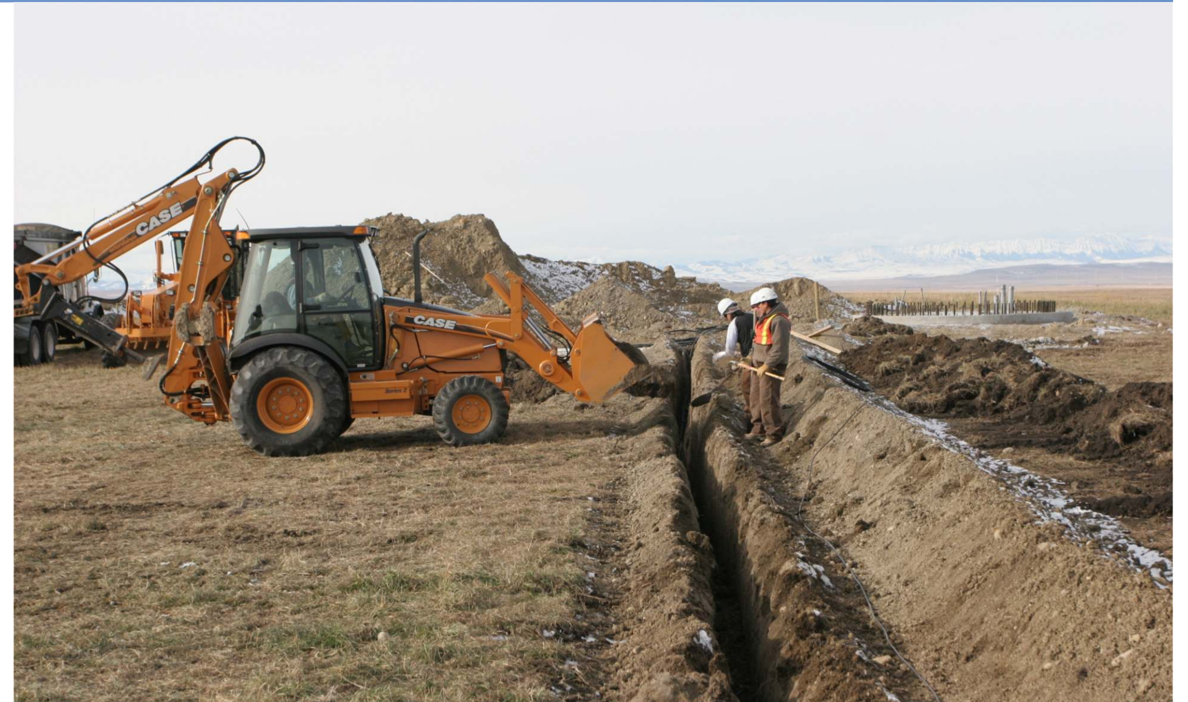
Placing sand in trench
