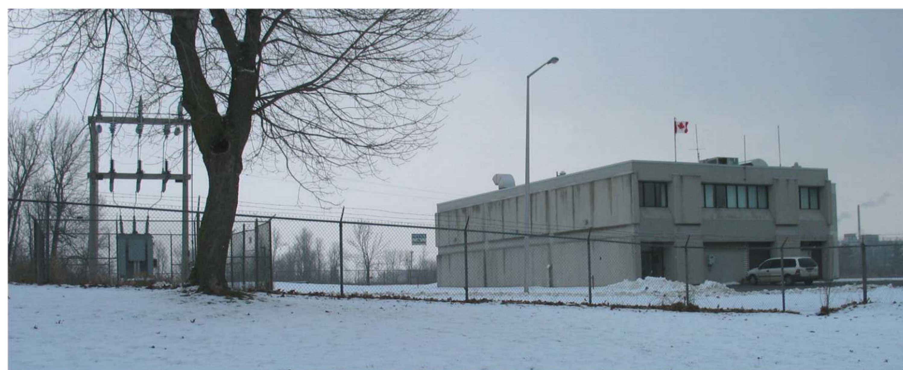
Water Treatment Plant building and transformer (looking northeast)
