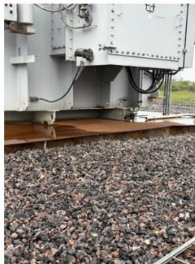
Figure 3: Temporary Transformer T2 on Wood Structure Support
