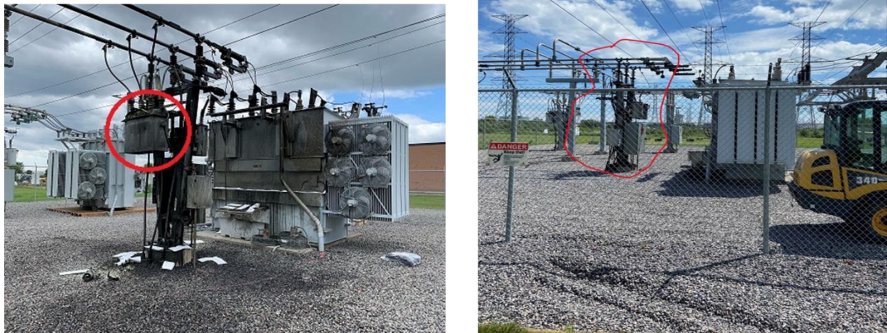
Figure 4: F1 Recloser Failure in July 2022
