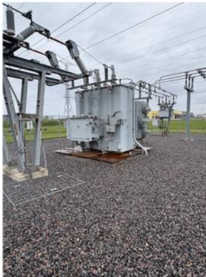
Figure 3: Temporary Transformer T2 on Wood Structure Support
