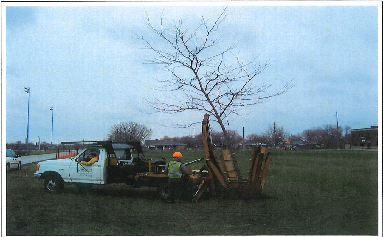
Trees which needed to be relocated within the park were done so using a tree spade.
