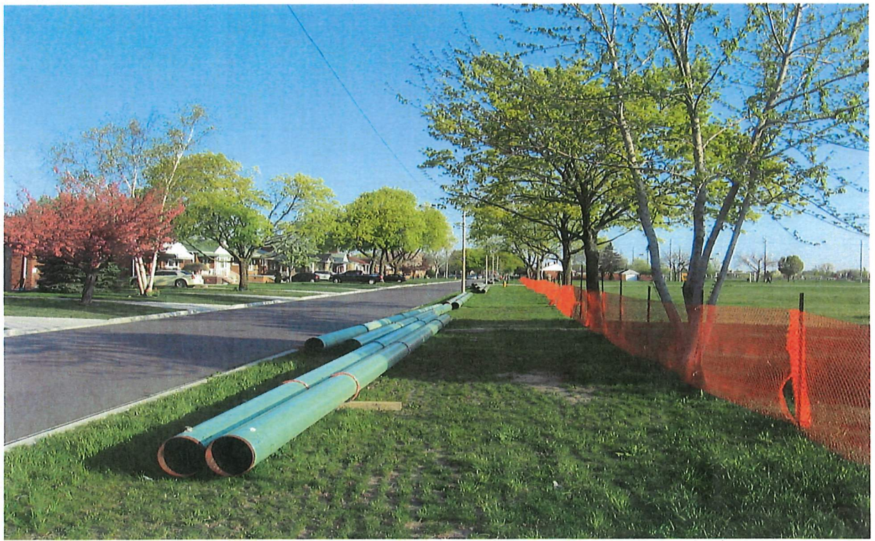
Temporary fencing was installed along school yards for added safety.
