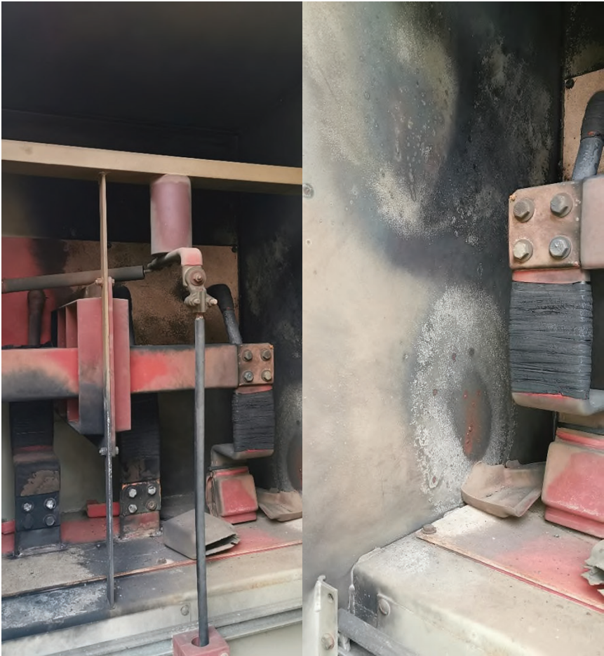
Figure 31: Images of a recent outage at a OPUCN owned switchgear
