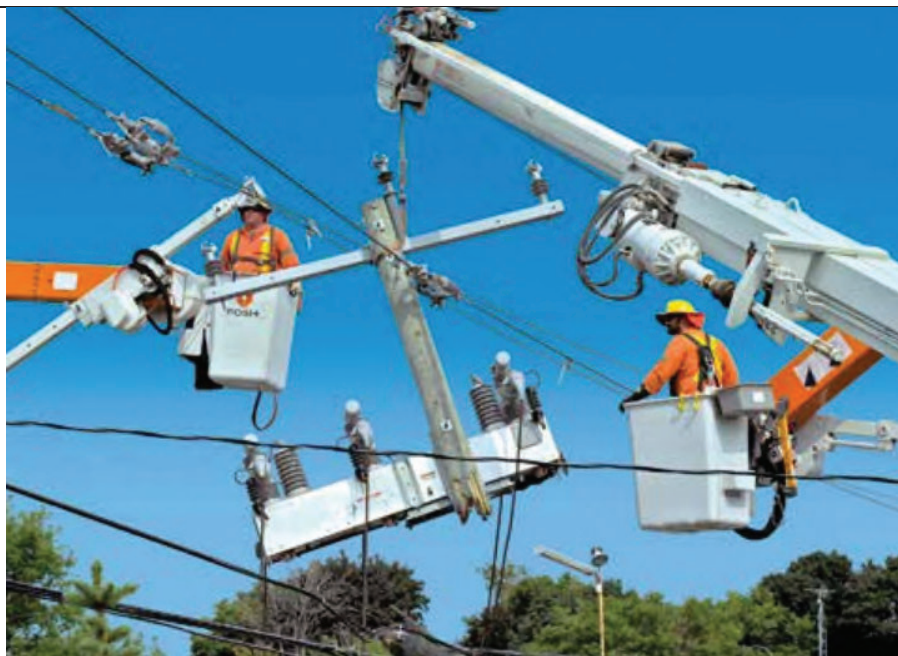
Figure 42 - An Automated Switch Mounted On A Pole That Was Struck By A Vehicle
