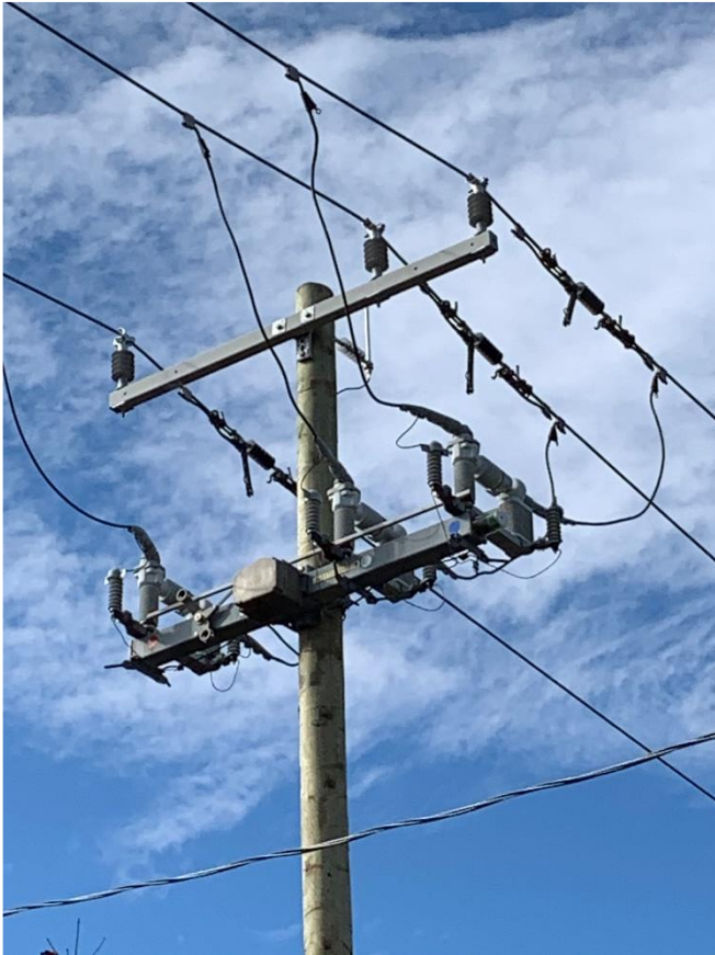
Intelligent (automated) switches
