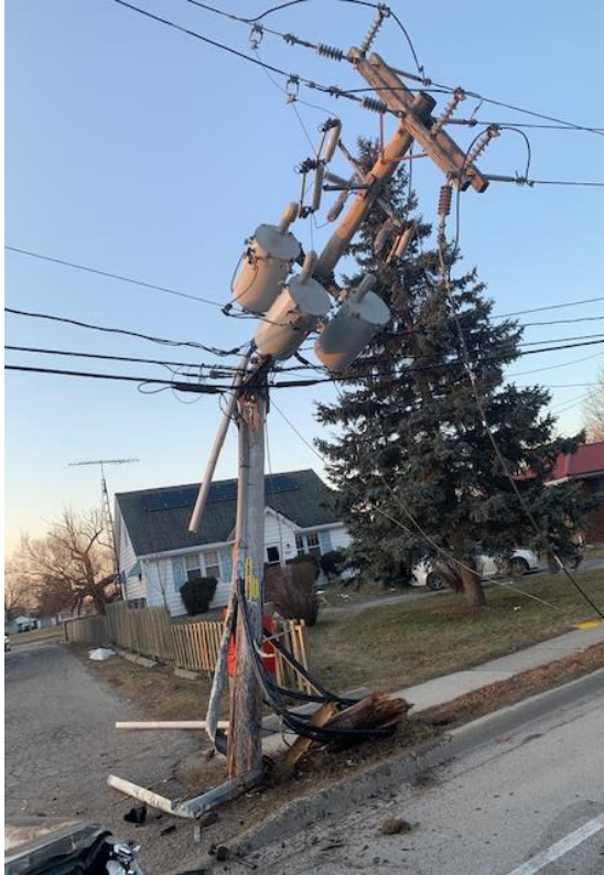
A damaged Entegrus distribution pole.
