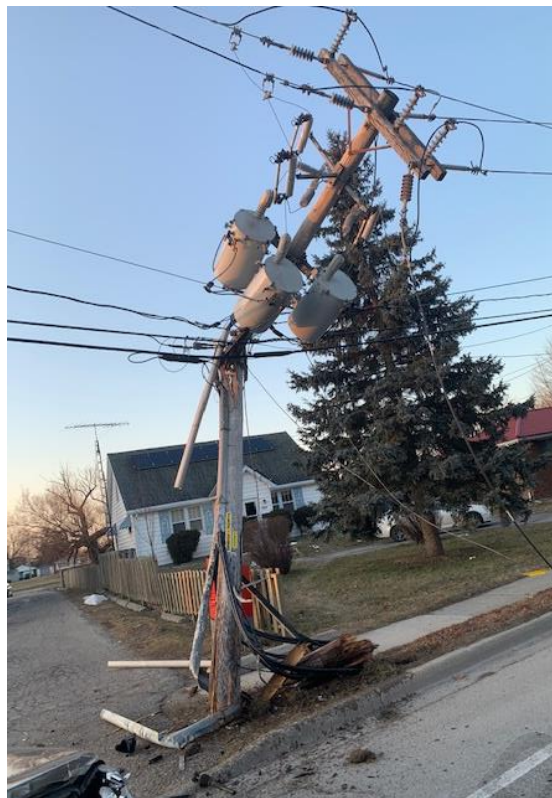
A damaged Entegrus distribution pole.
