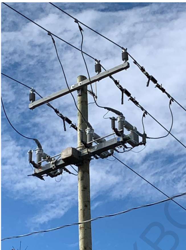
Intelligent (automated) switches
