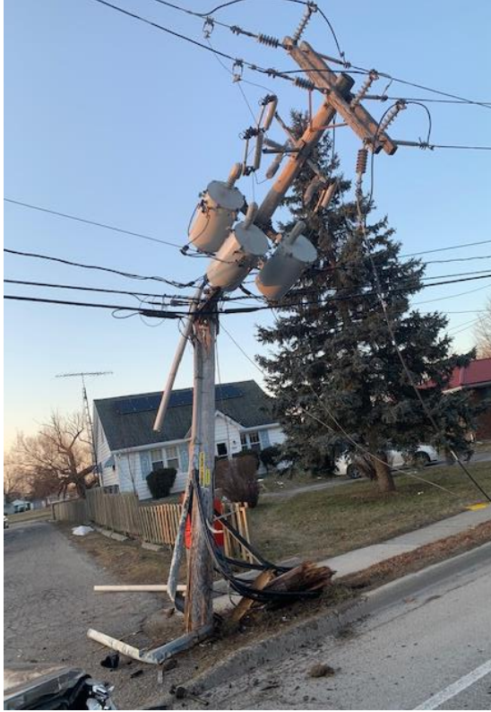
A damaged Entegrus distribution pole.
