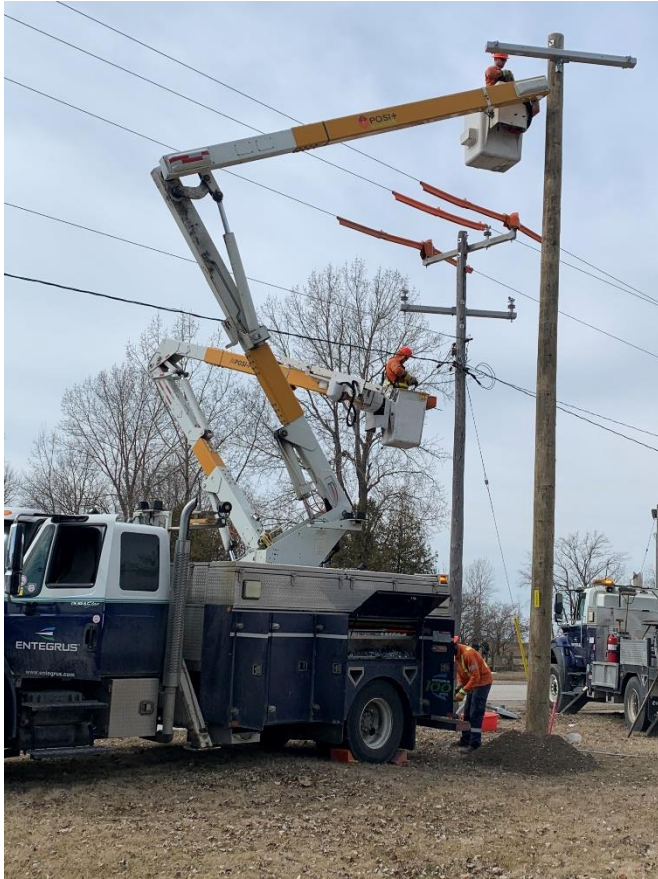
An Entegrus crew installing a new pole.
