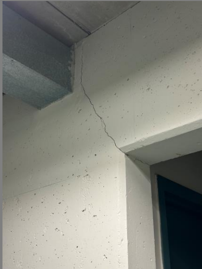
Cracks in Basement Walls Location : Stores Area
