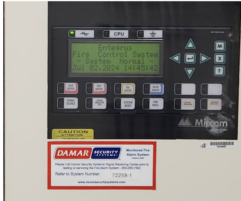
Figure 51: Fire Alarm Control Panel
