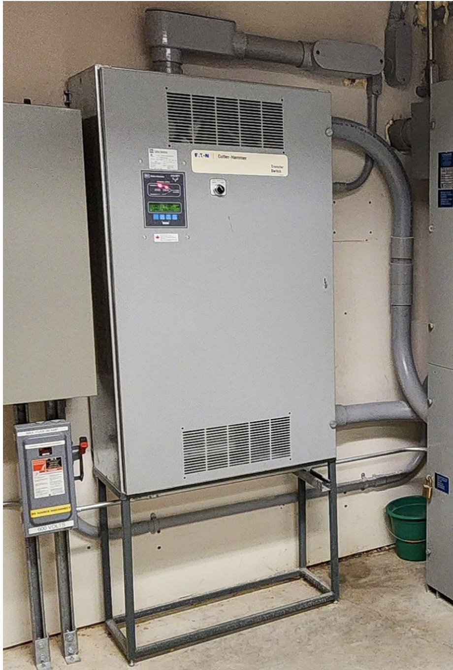
Figure 45: 400A Automatic Transfer Switch
