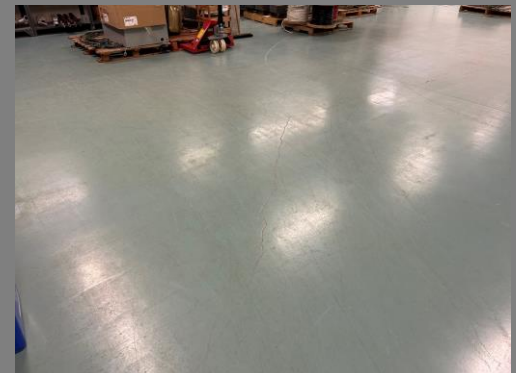
Basement slab cracking through epoxy flooring.
