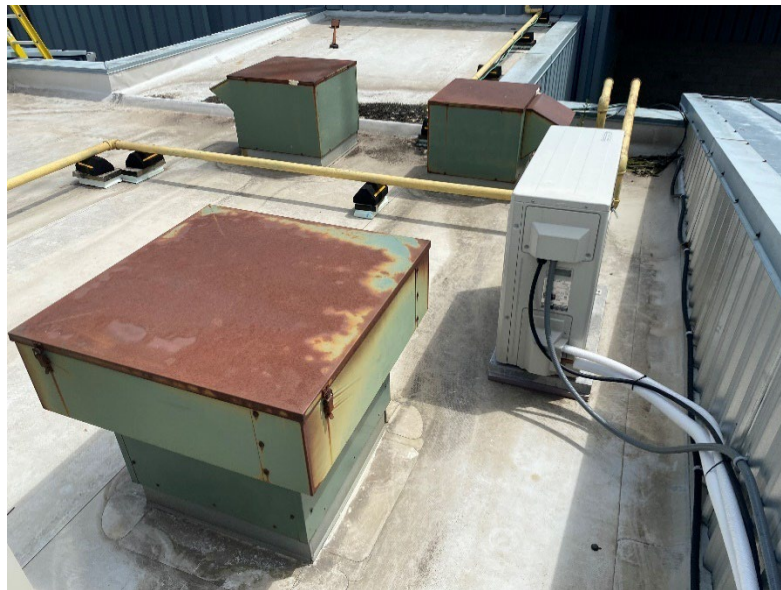
Figure 34: Exhaust Fans on Flat roof
