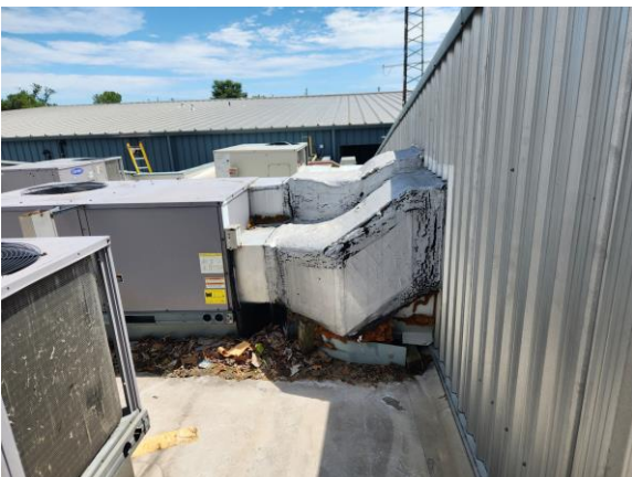
Debris collecting by AHU. Location: Main Office
