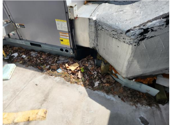
Debris collecting by AHU. Location: Main Office
