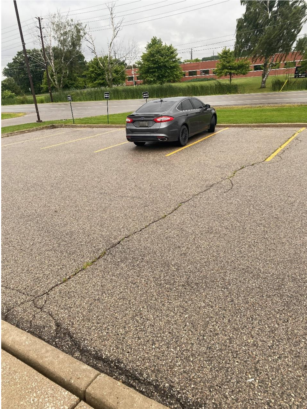
Visitor parking area – front entrance – some minor asphalt cracking. Minor repairs/ filling recommended. Monitor for further damage
