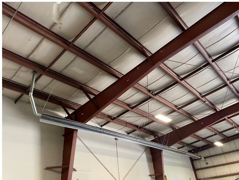
Figure 38: Infrared Tube heater (typ)
