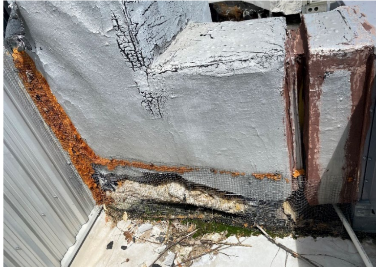
Figure 30: Existing exterior ducting insulation
