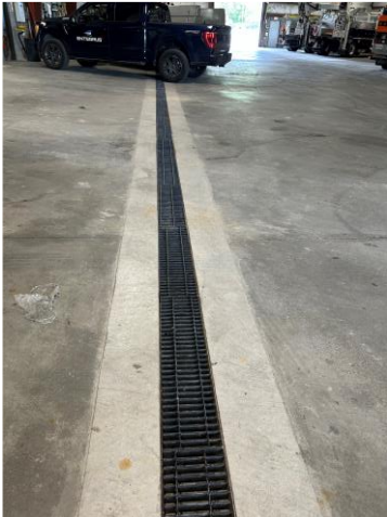
Reconstructed floor trench. Location : Garage
