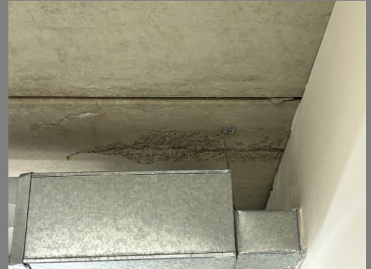
Localized precast concrete soffit spalling Location : Women's Washroom
