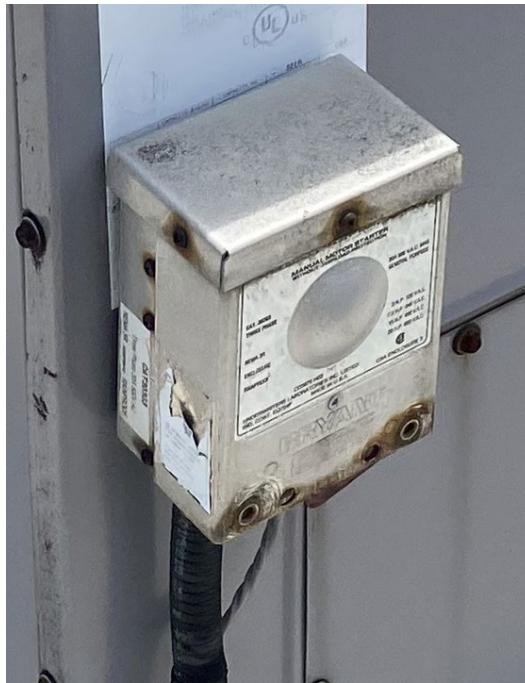
Figure 41: Rusty Rooftop Disconnect Switch
