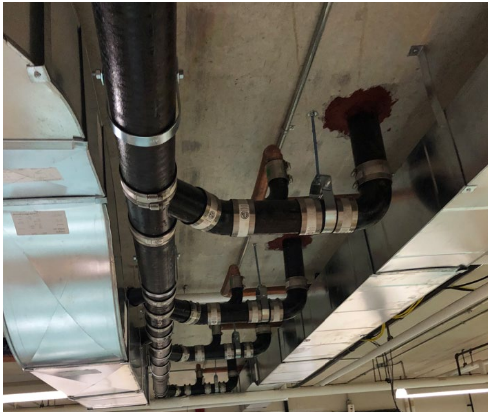
Figure 7: Example of exposed sanitary piping in storage room.
