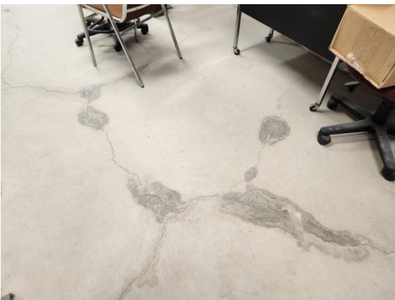
Signs of water infiltration (monitor) Location: Basement electrical room
