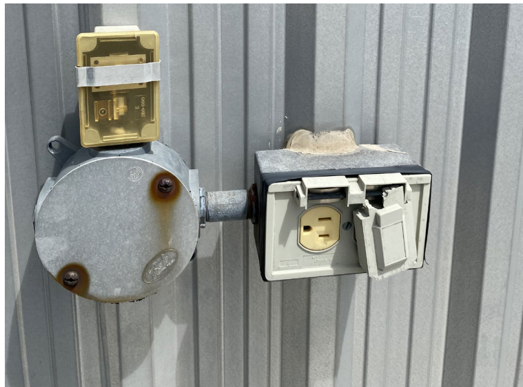
Figure 58: Broken Receptacle Cover on Roof
