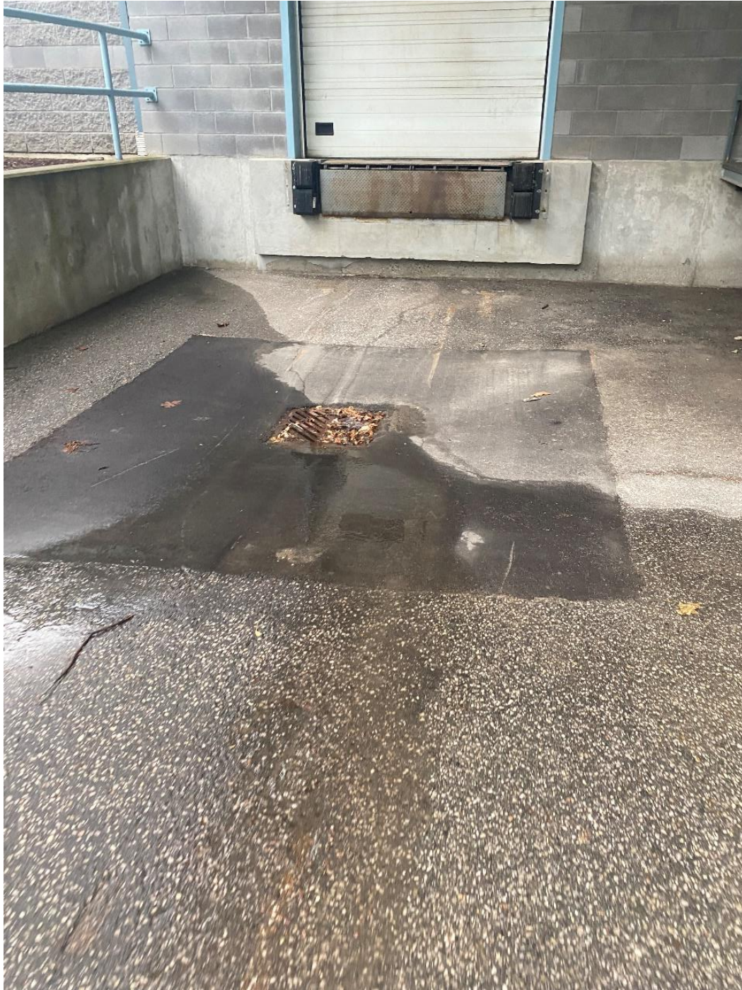
Driveway loading dock – some asphalt appears to have been repaired. Monitor to ensure cracking or further settlement does not occur.
