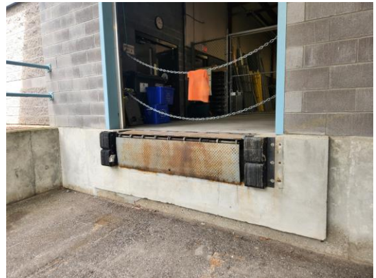
Rusting appearing on Loading Dock Location: Garage
