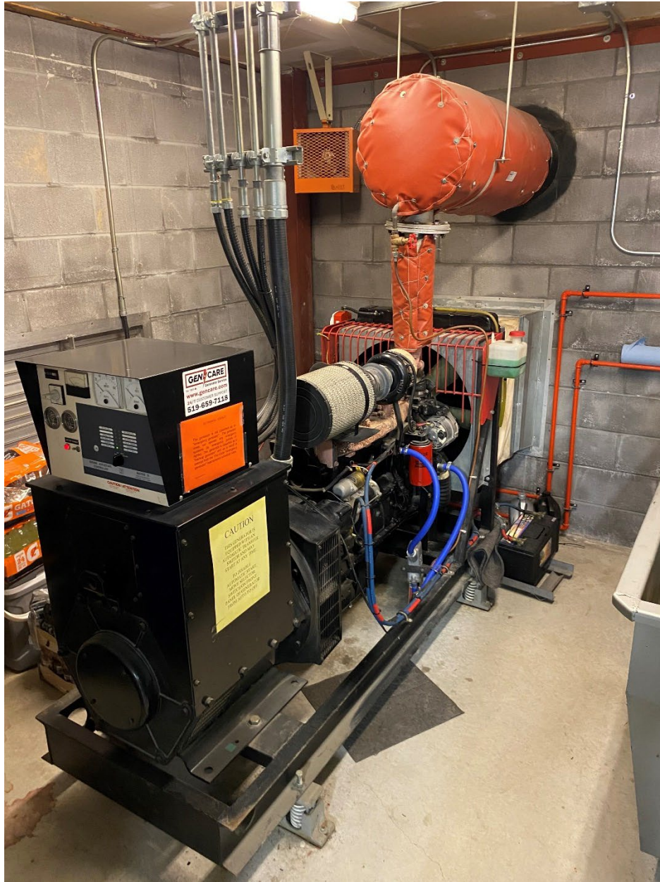
Figure 44: 100 kW Generator
