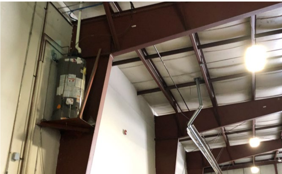
Figure 26: Gas fired heater located in Garage as well as water heater
