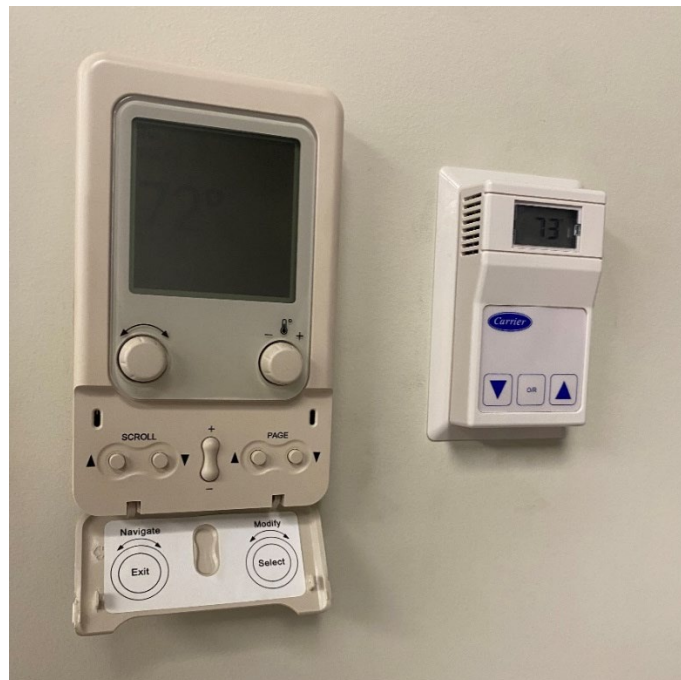
Figure 29: Controls/T-stat within interior Spaces
