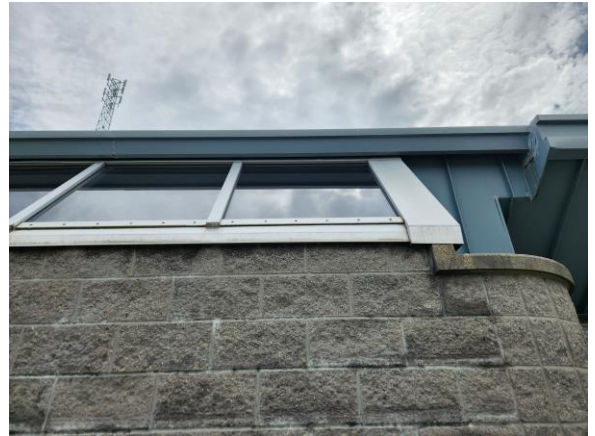
Efflorescence on Split Face Block – Main Entrance
