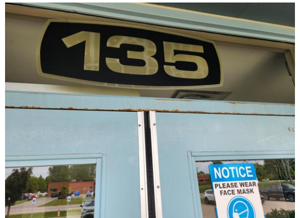
Monitor: Rust forming on window framing (Repaint) Location: Main Office
