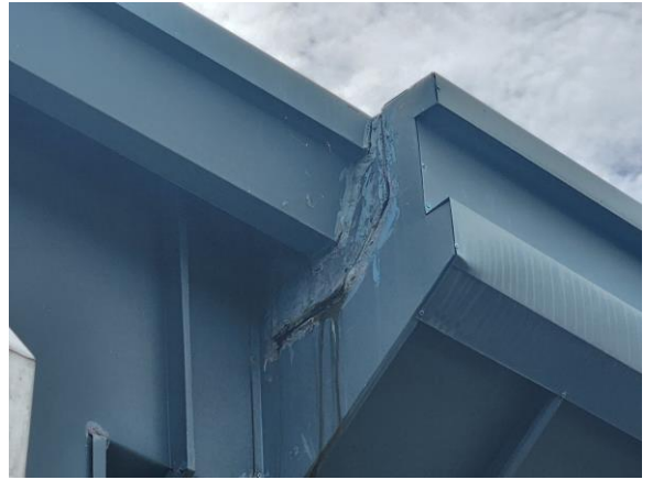
Paint deterioration (minor) on eaves and gutter.
