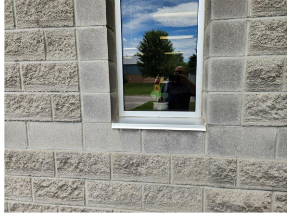
Sample of Aluminum Windows and Sill Location: Main office
