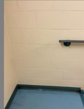
Masonry Stepped cracking Location : Stairwell
