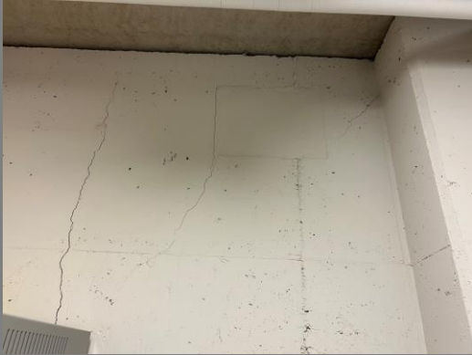
Cracks in Basement Walls Location: Stores Area
