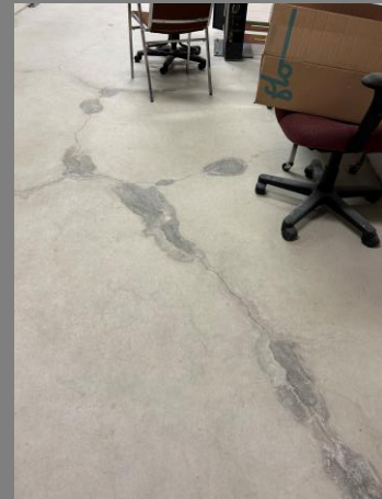
Basement slab cracks and staining Location: Electrical Room
