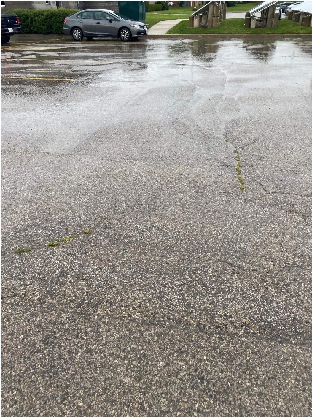
Employee parking – asphalt cracking noted in a few locations. Generally, asphalt in good shape. Minor repairs/ filling recommended. Monitor for further damage
