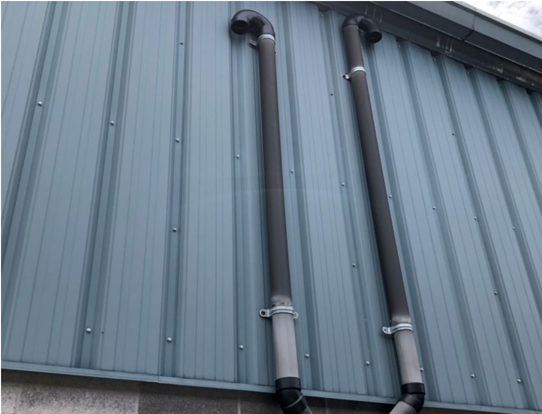
Figure 16: Oil Interceptor Vents
