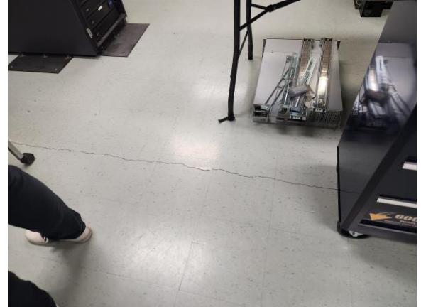
Crack in VCT flooring. Monitor Location: IT room
