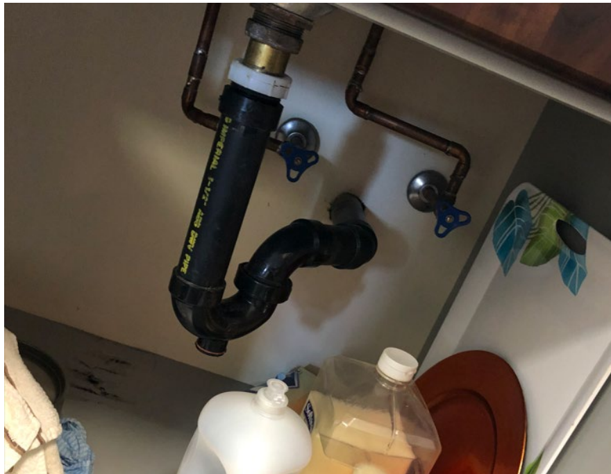
Figure 13: Typical ABS under counter.
