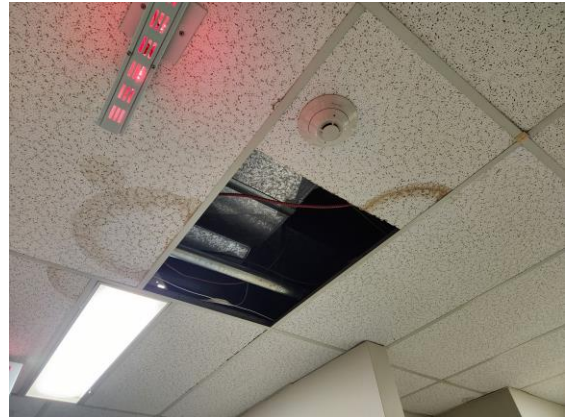
Water staining related to HVAC equipment Location: Main Office
