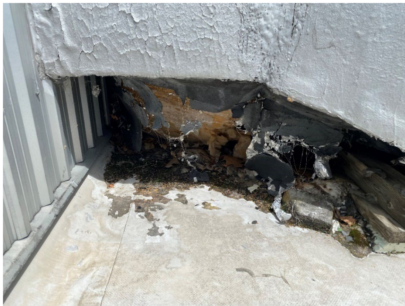
Figure 31: Existing torn ducting insulation
