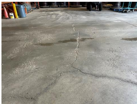
Regular slab on grade cracking. Location : Garage
