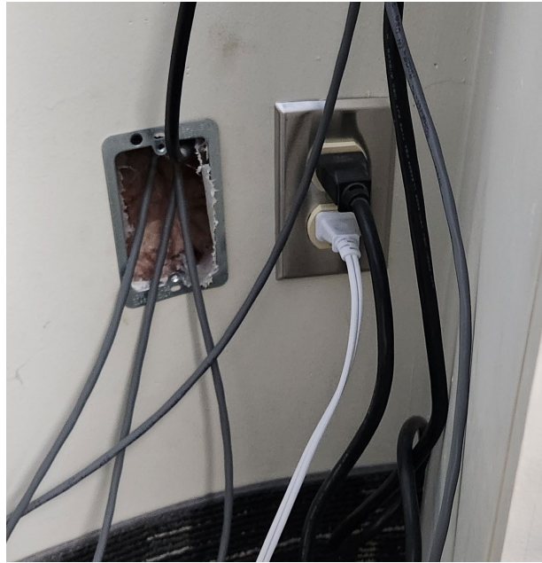
Figure 57: Cover plate missing
