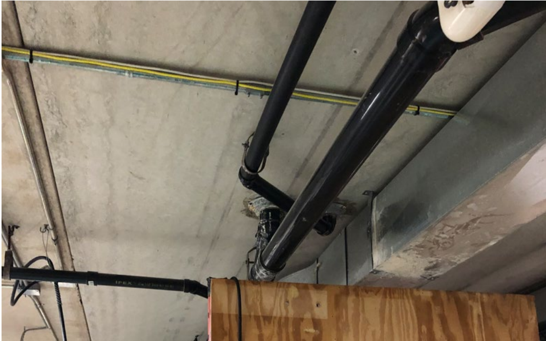
Figure 14: Typical ABS in ceiling spaces.
