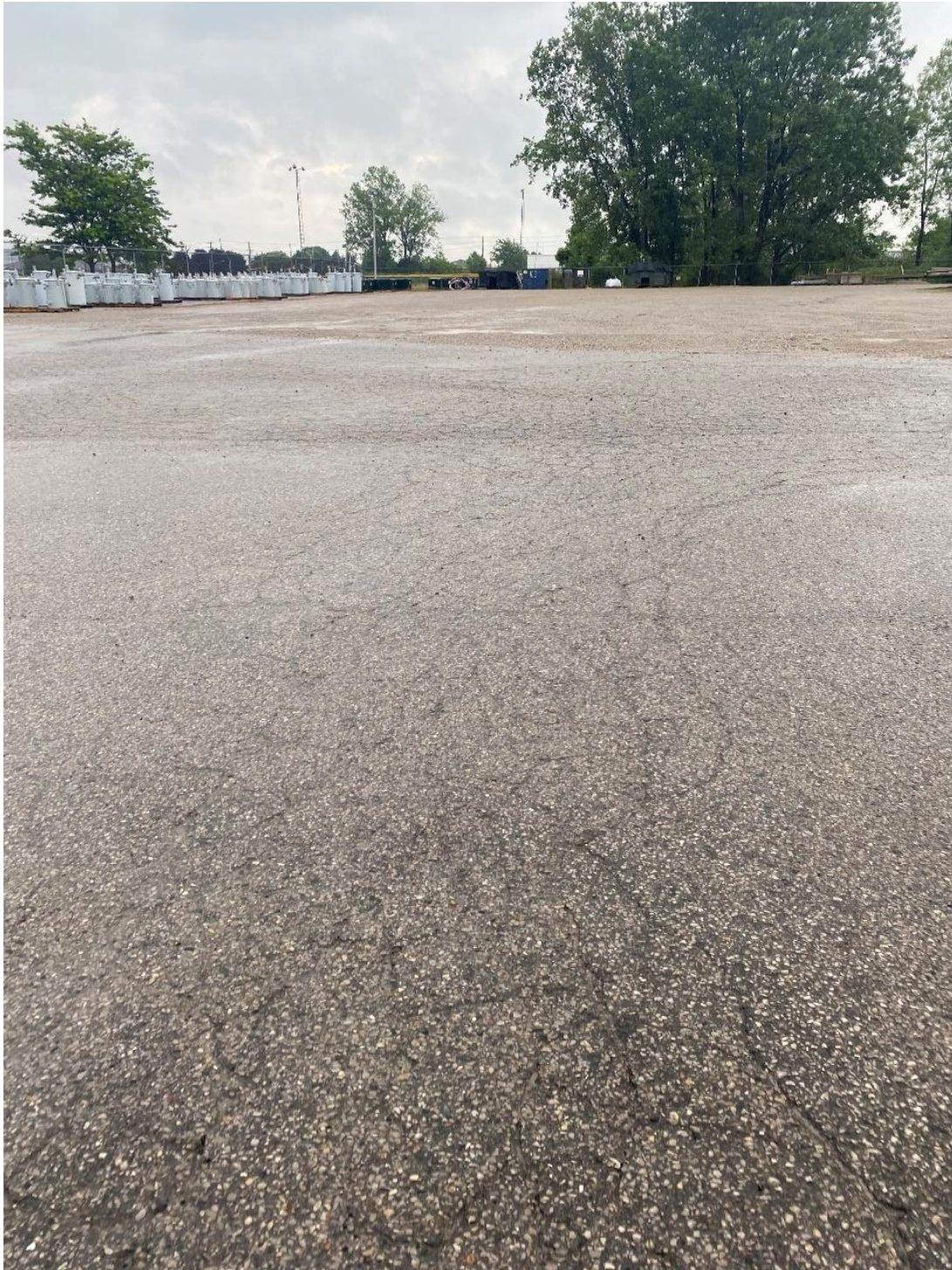
Back parking lot- minor cracking observed. Minor repairs/ filling recommended. Monitor for further damage.
