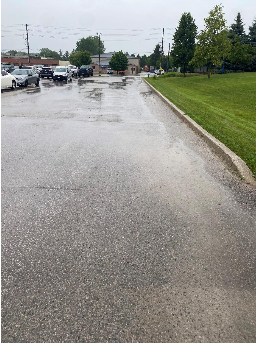
Employee parking area – asphalt generally in good condition, minor cracking should be monitored.
