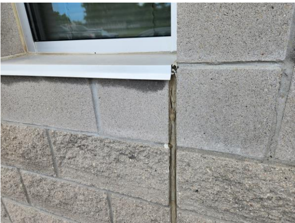
Control joint sealant failing - Sample
