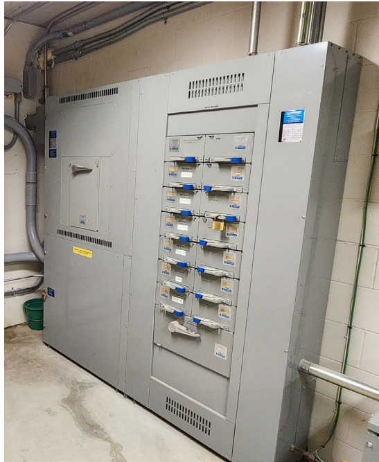
Figure 42: Electrical Service Switchboard
