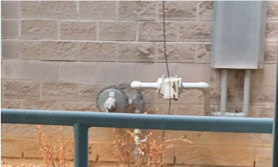
Figure 25: Gas meter header on exterior of building.
