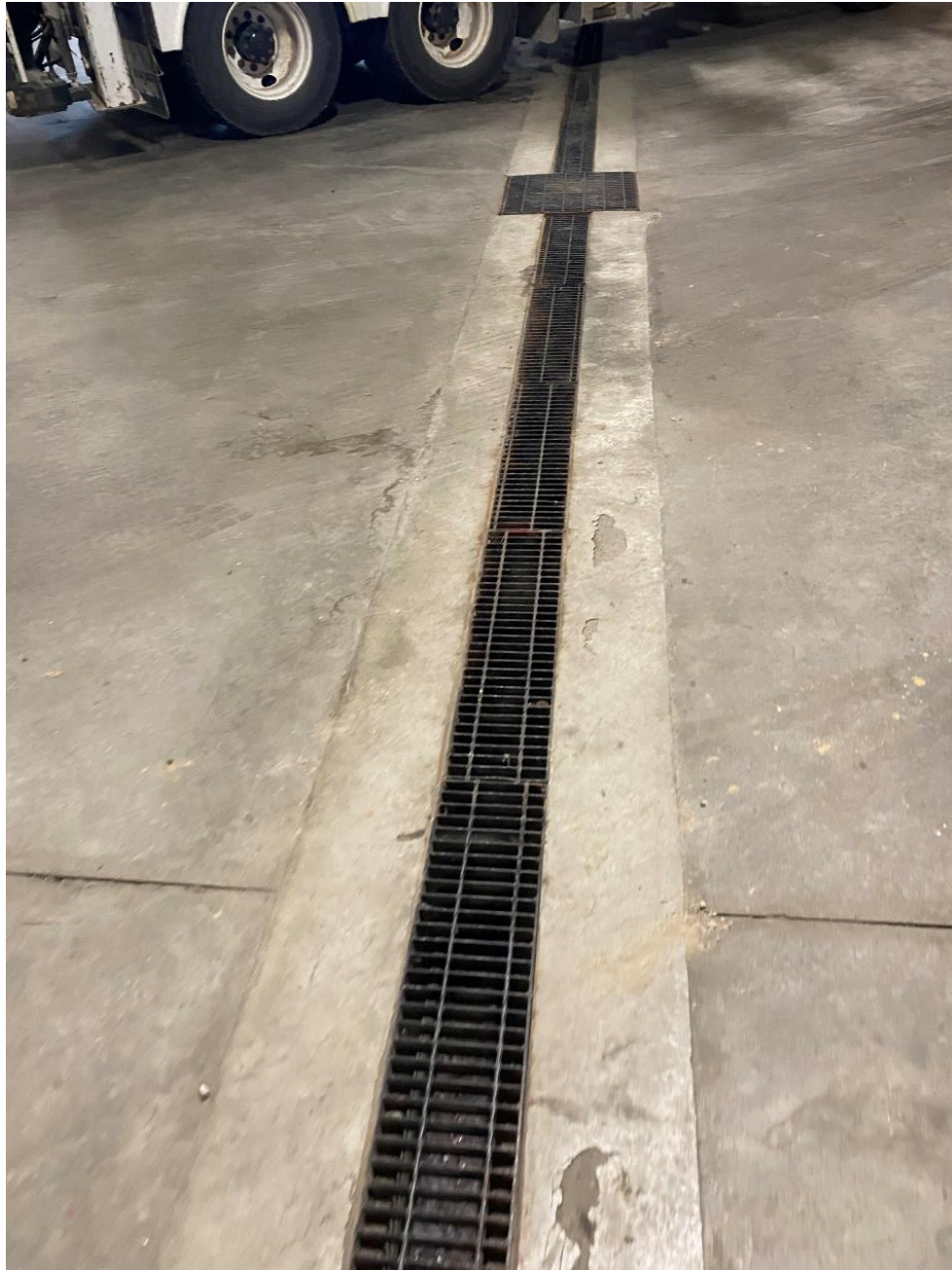
Trench Drain 2 – Located in garage – Clean and in good condition.
