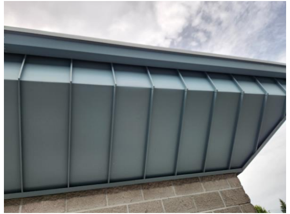
Sample of Metal Soffit Bay
