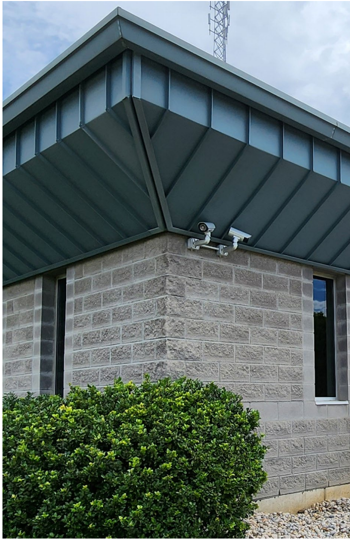
Figure 55: Exterior CCTV Camera
