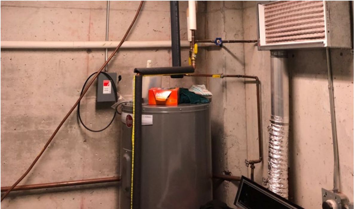
Figure 8: Electric Hot Water Heater located within Laundry Room
