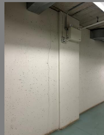
Cracks in Basement Walls Location: Corridor
