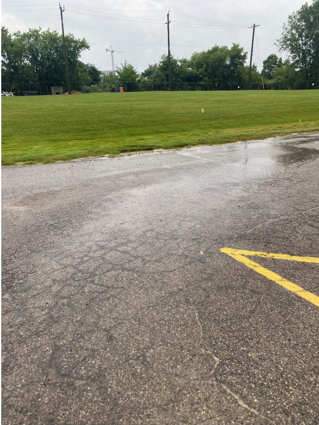
Back drive aisle, asphalt cracking. Asphalt will need to be removed and replaced.
