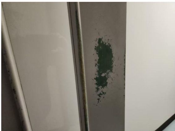
Sample of paint peeling – to be painted Location: Main Office
