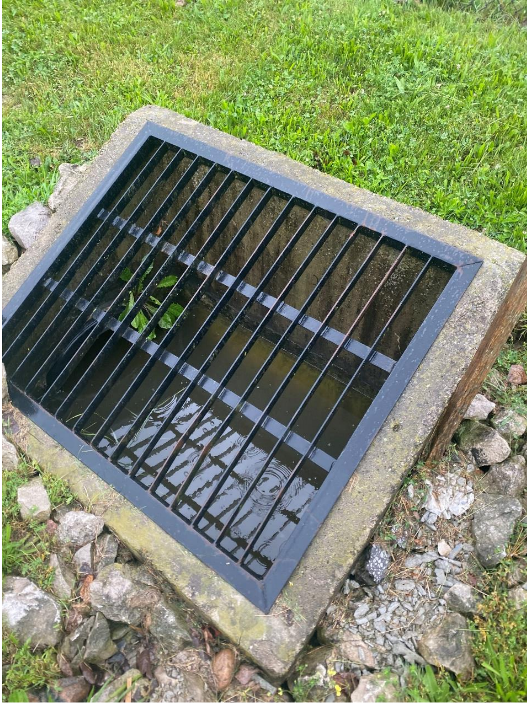
DICB – SWM outlet - rear of building – no issues
