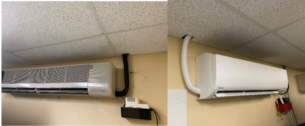
Figure 37: Existing Interior A/C Split Unit Heads and Cond. Pumps
