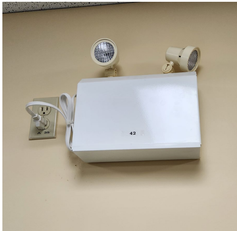
Figure 48: Remote Light Head/Battery Pack
