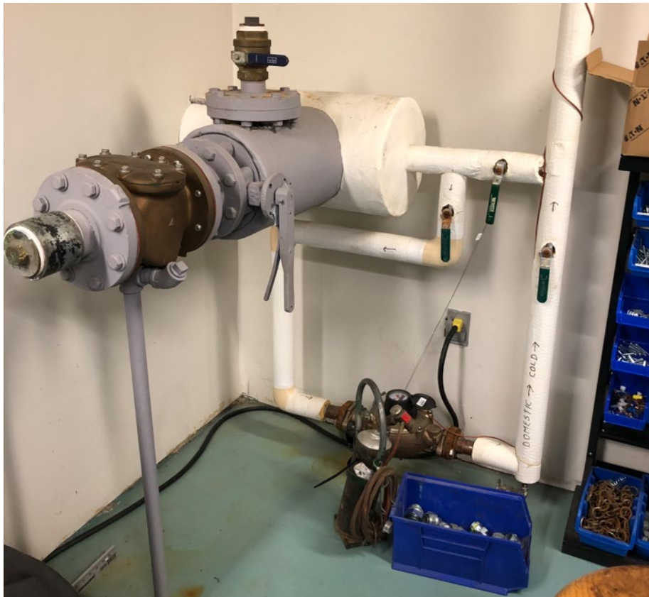
Figure 5: Existing Water Service entering building located in basement Room 011
