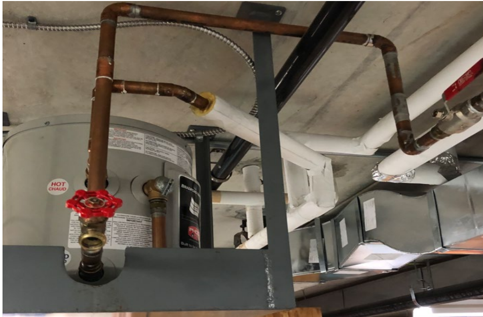
Figure 6: Electric Hot Water Heater hanging within Water Meter Room 011.
