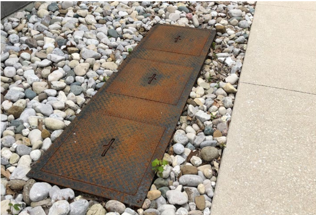
Figure 15: Oil Interceptor on exterior.
