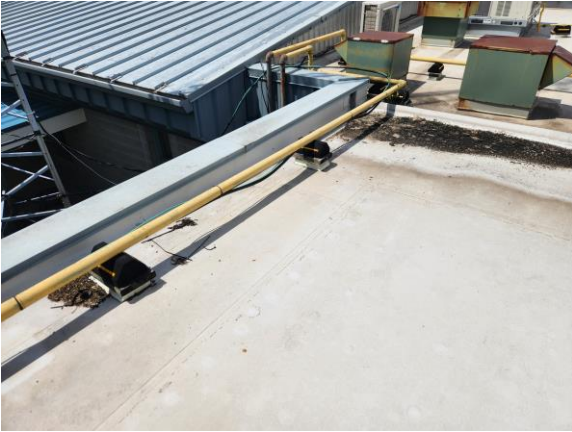
Sample: Single Ply Roof Membrane roof. Location: Main Office
