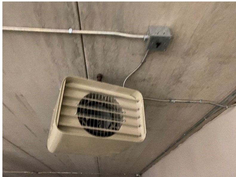
Figure 33: Basement Unit heaters
