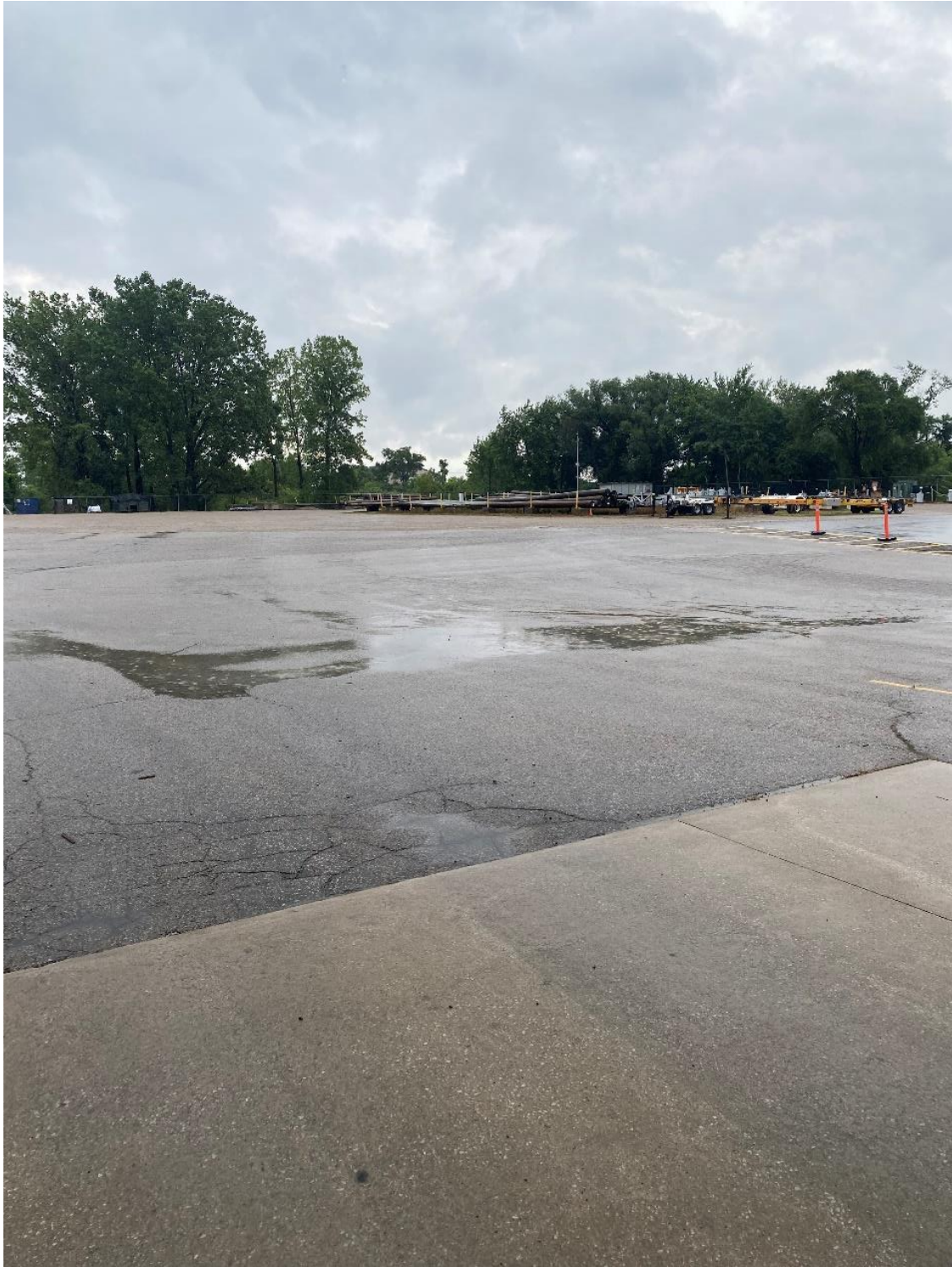
Back parking area, asphalt generally in good condition, some minor cracking. Minor repairs/ filling recommended. Monitor for further damage.
