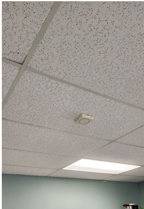
Figure 46: Light Fixture & Ceiling Mounted Occupancy Sensor
