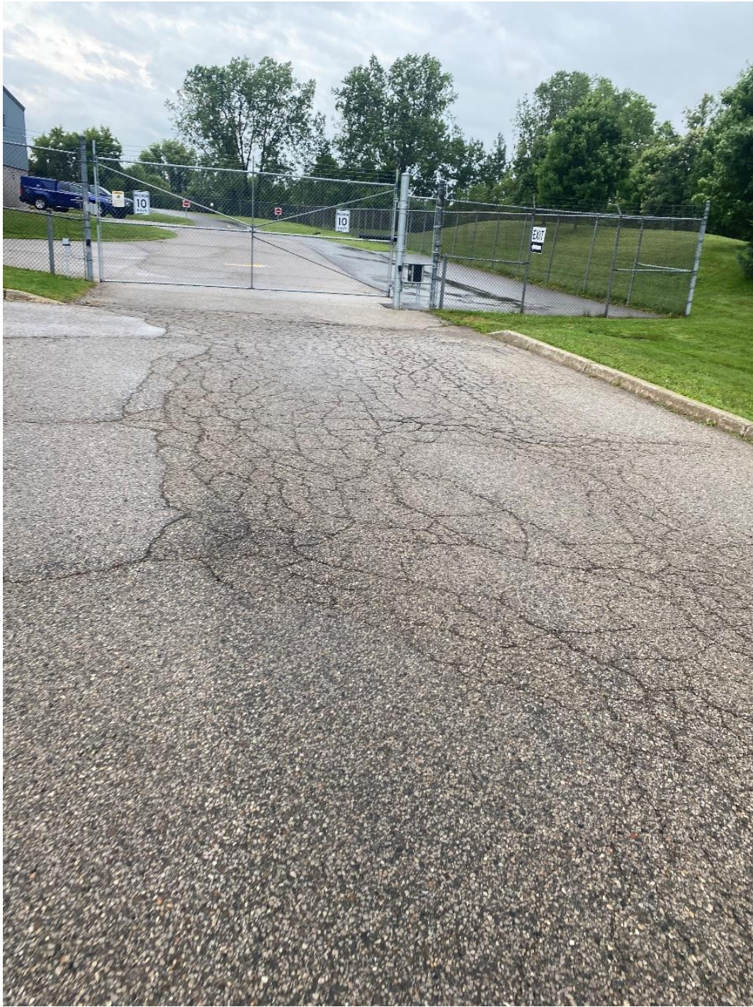
Front driveway – asphalt cracking and some separation along joint. Asphalt will need to be removed and replaced.
