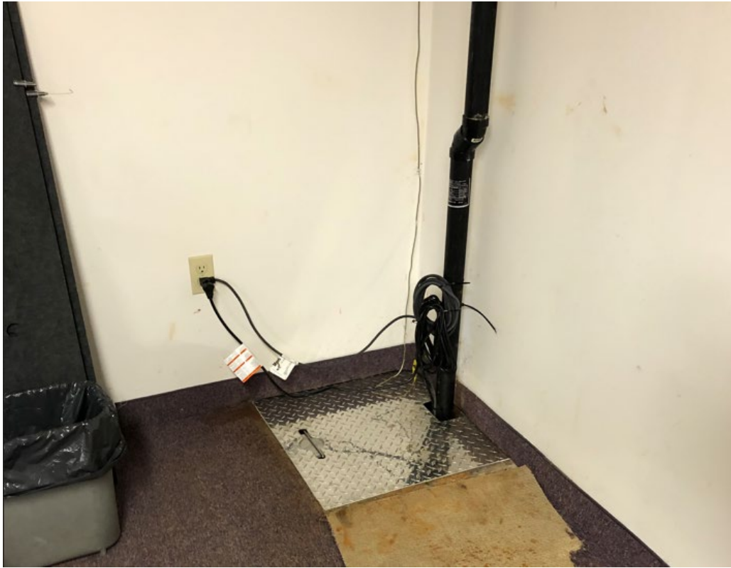
Figure 10: Weeping Tile Sump Pump located in Basement Room 002
