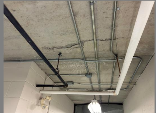
Localized Concrete precast soffit spalling. Location: At freight elevator
