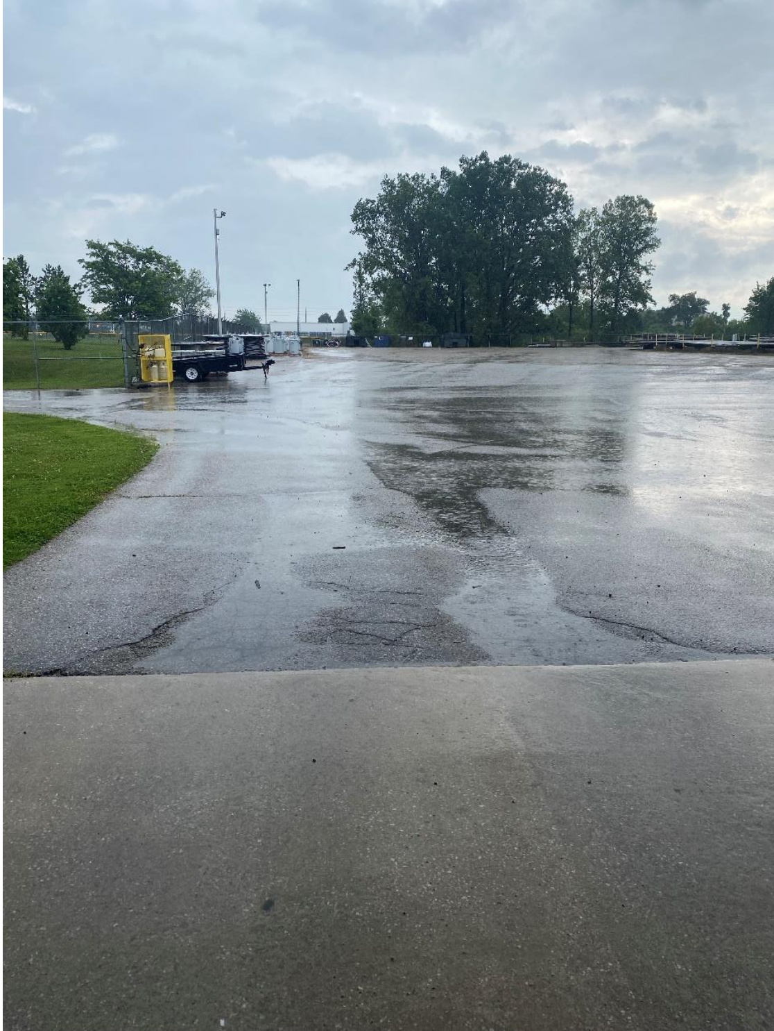
Driveway into garage is settling/cracking. Asphalt will need to be removed and replaced.
