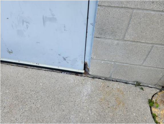
Frame rusted out Location: Garage
