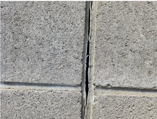
Repair: Control Joint Failing Location: Garage
