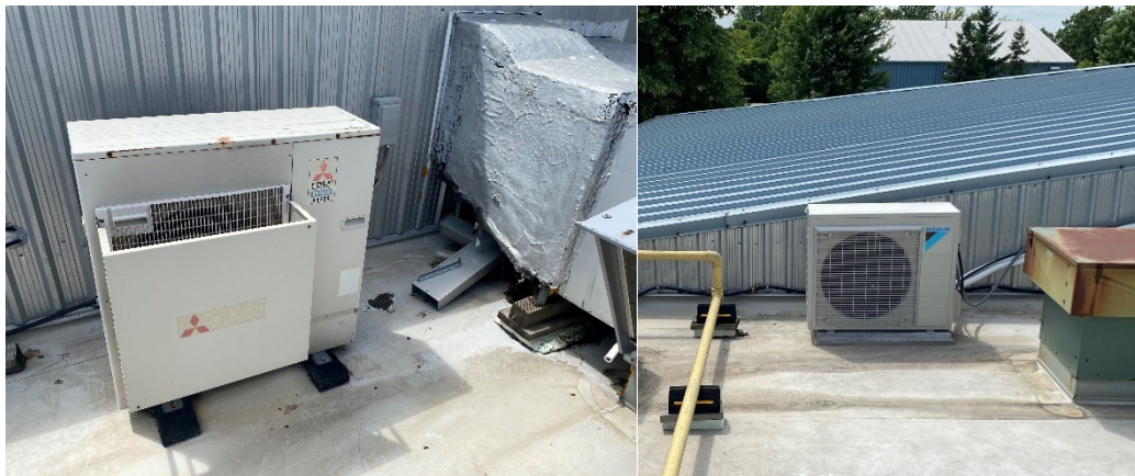
Figure 36: Existing Exterior Condensers
