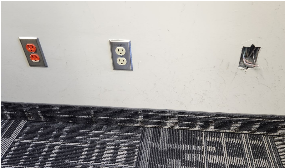
Figure 56: Junction box cover plate missing
