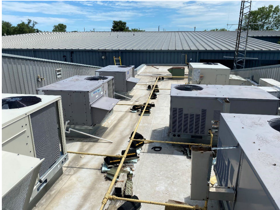
Figure 28: Existing RTU's on Office Roof
