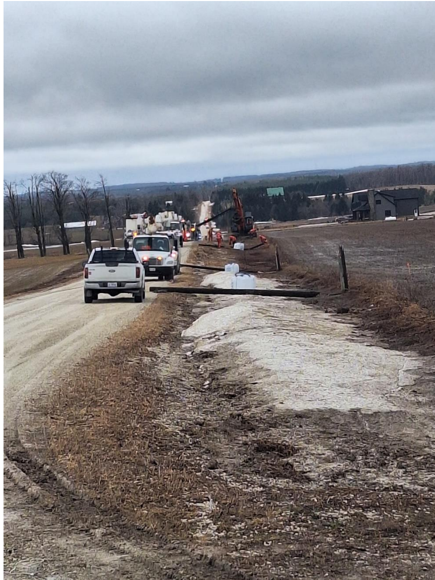
Figure 2: Series of Poles Requiring Replacement
