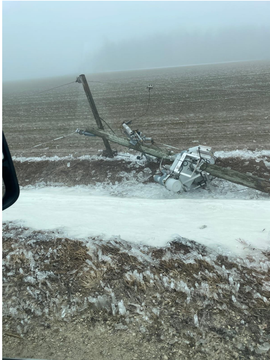
Figure 1: Fallen Pole/Transformer
