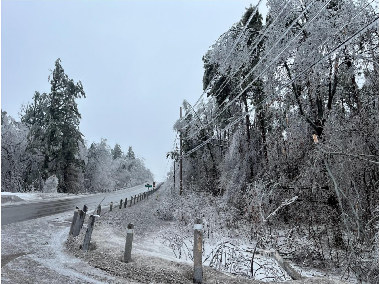
Figure 10: Ice Accumulation on Lines and Trees
