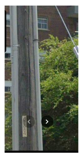
One existing pole (Pole 7684) supported two egress cable risers, which is no longer considered best practice due to the increased reliability (animal contact, pole failure) and safety (clearance issues) risk posed by a single point of failure affecting two main feeders. This pole was replaced, and an additional dedicated pole was installed to separate the feeders.
