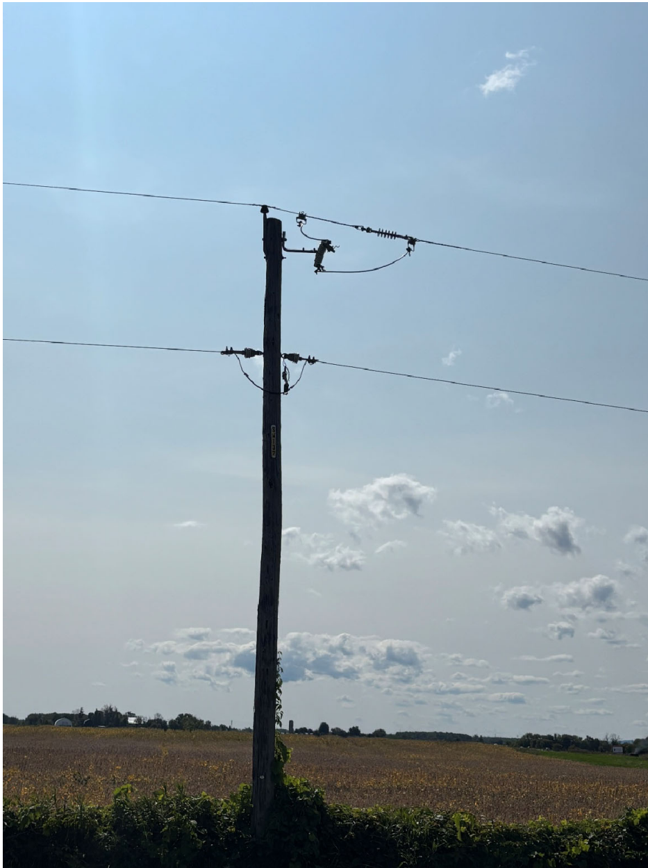
Picture #5: Hydro One SW1137
