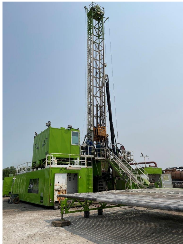
2. Well drilling rig set up on the Waubuno temporary drill pad
