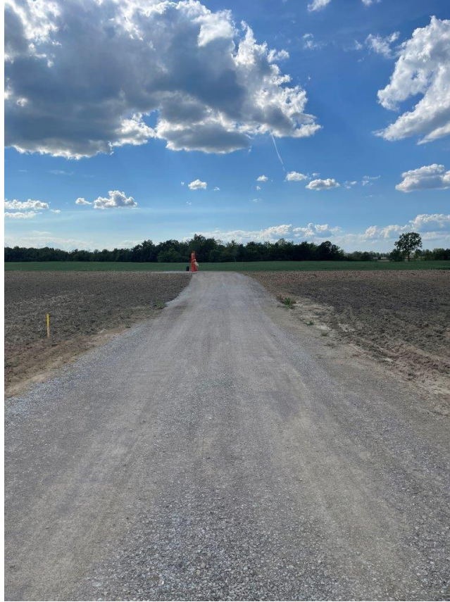
3. Permanent access road to well UW4.
