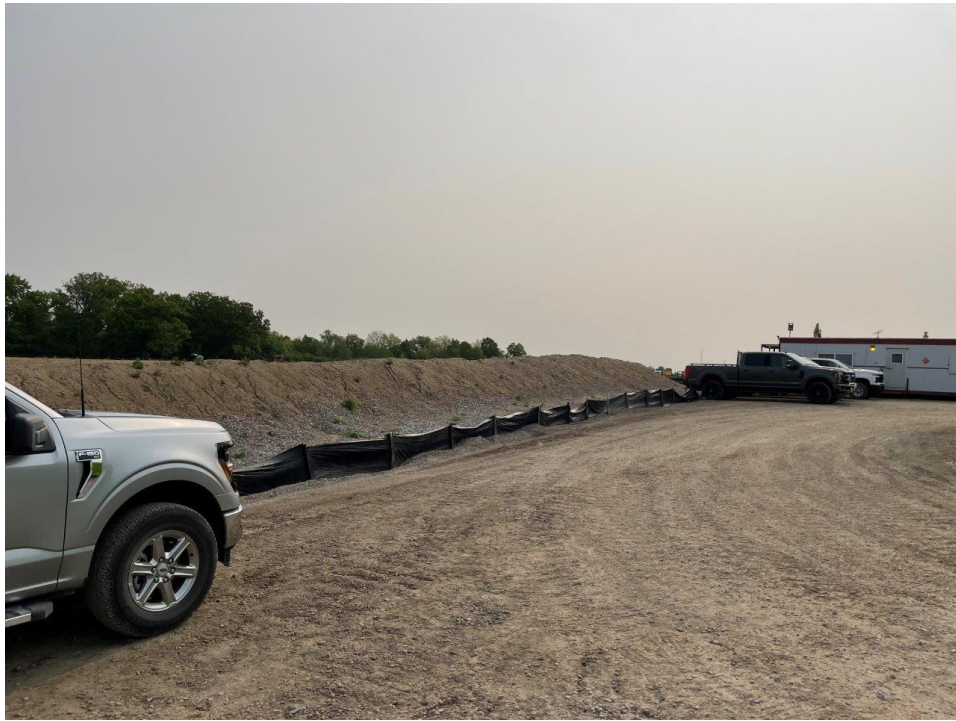
1. Temporary drilling pad, topsoil storage and silt fence (sediment and erosion control)
